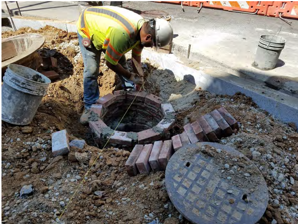
Adjusting Sewer Manhole at the NE corner of N Street Eastside
