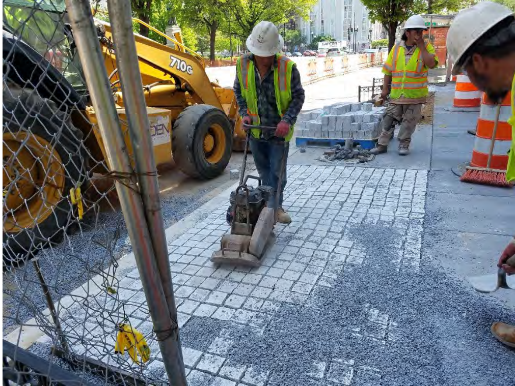
Placing Granite Cobble Stone between Thomas Circle and N Street Westside
