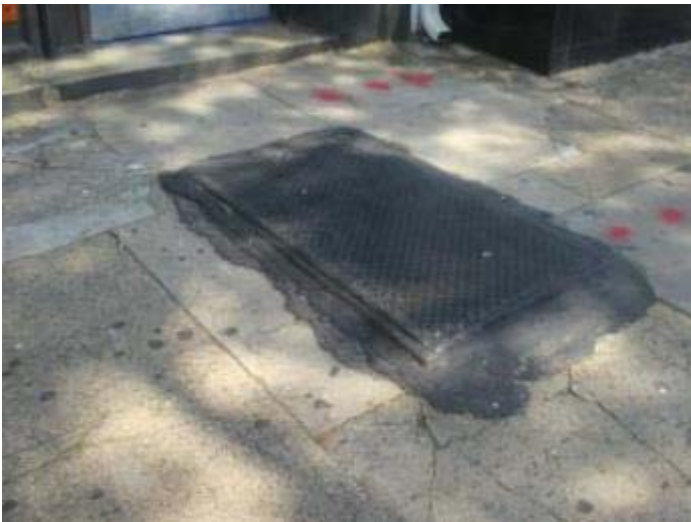
Existing Building Vault
