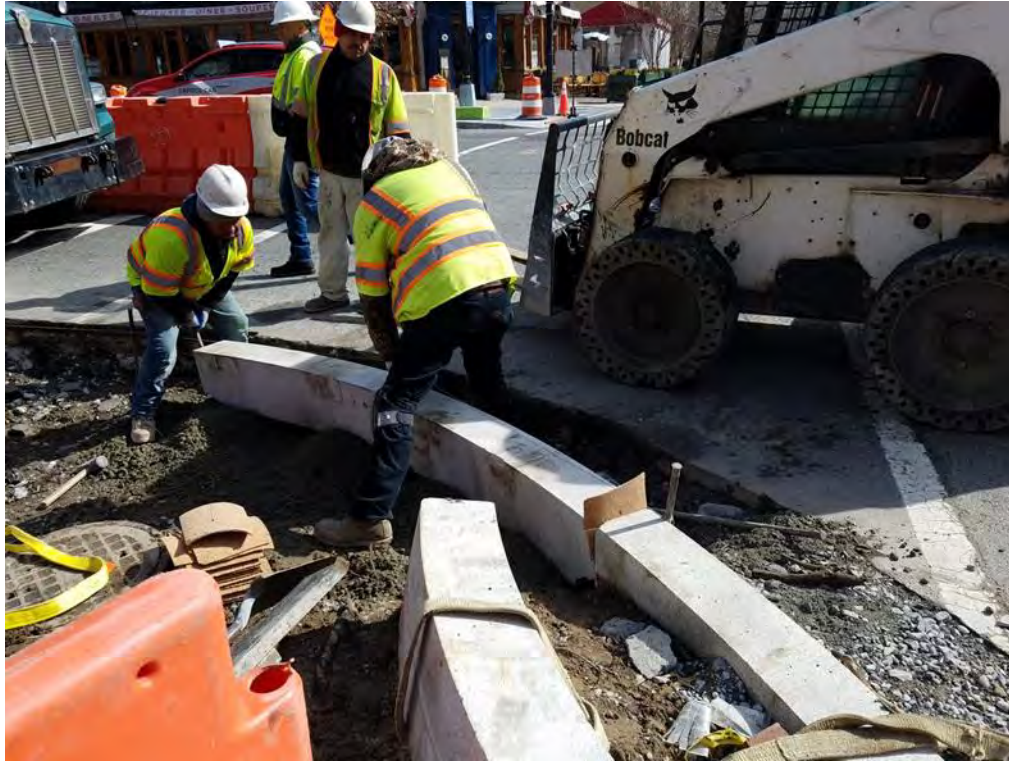
Installation of Granite Curb at the SW corner of 14 th and Q Street
