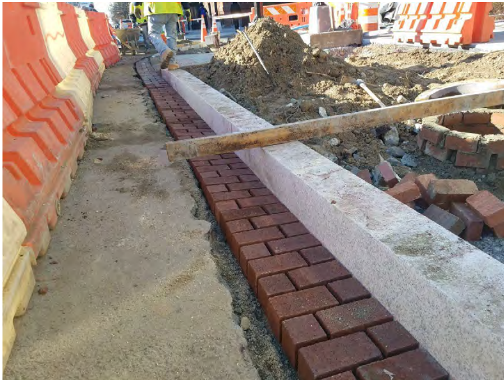
Installation of Granite Curb at the SW corner of 14 th and Q Street
