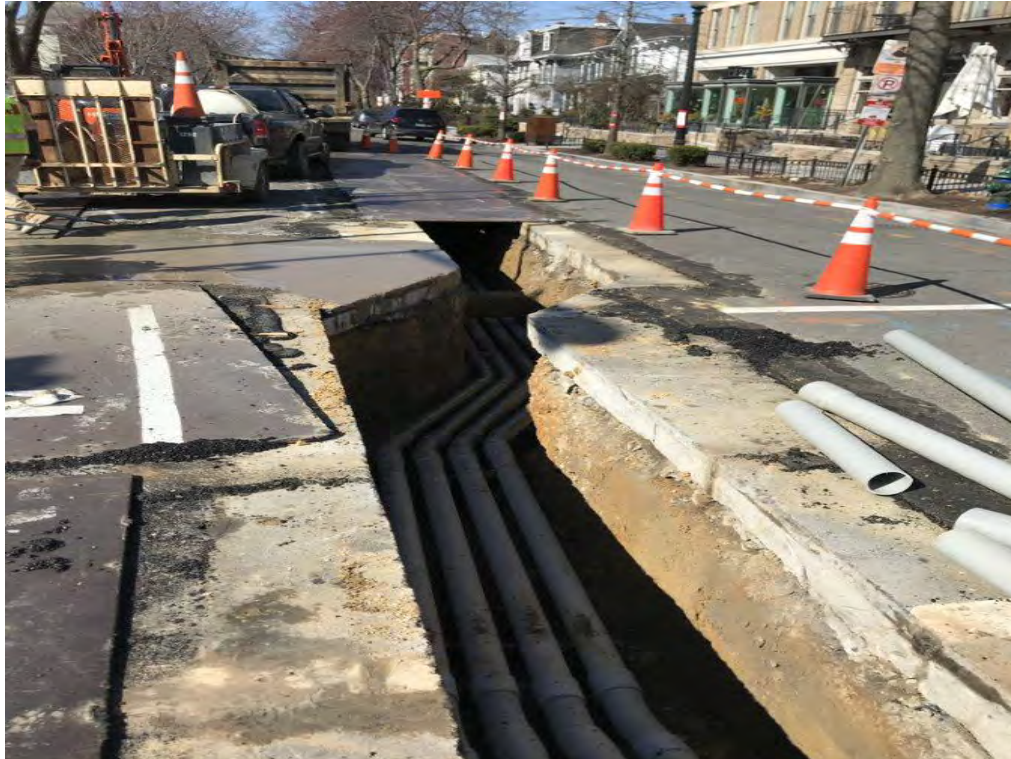
Installation of 4" PVC Conduit on S Street
