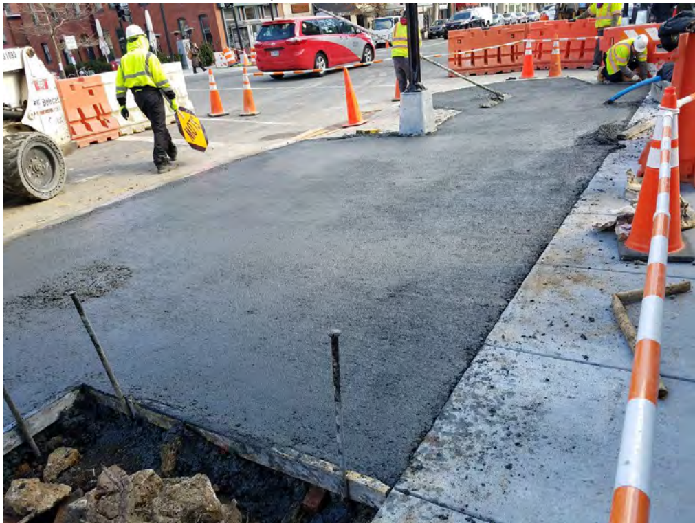
Installation new PCC Sidewalk
