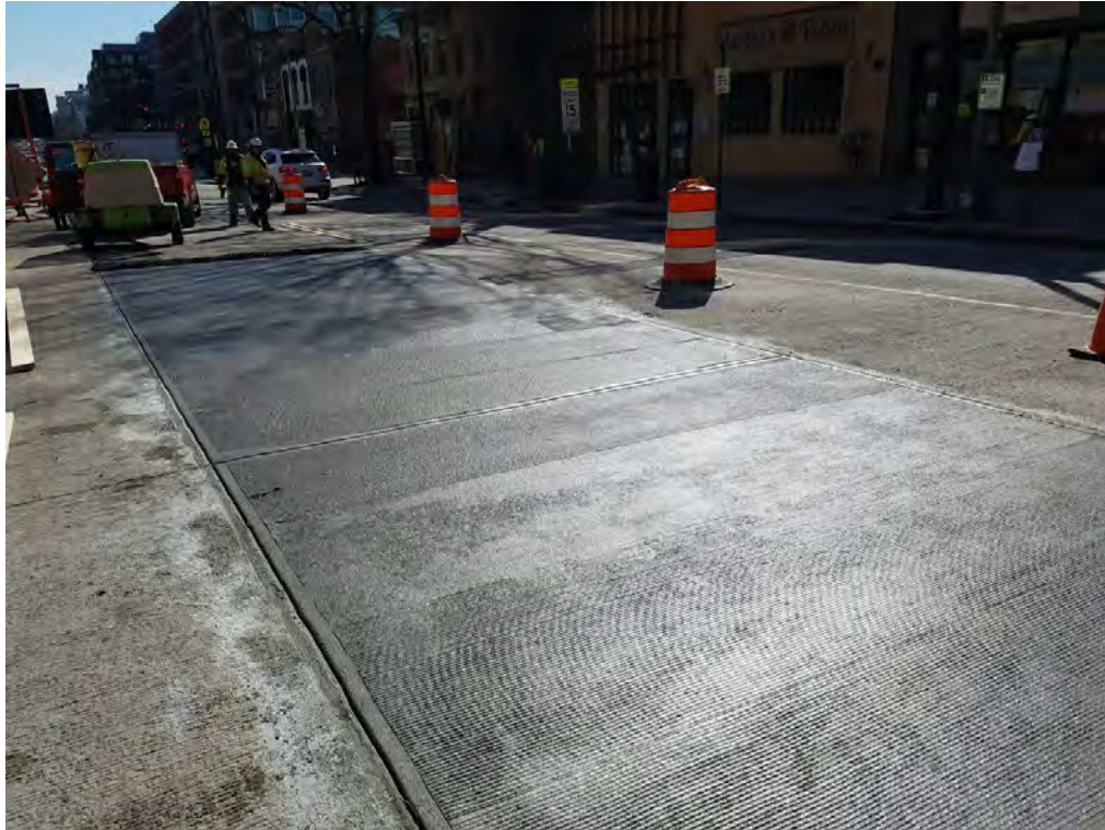
PCC Pavement Repair between Florida Ave and W Street
