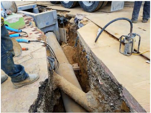
Installation of 15" PCC Sewer Connection Pipe at the NE corner of Rhode Island Ave
