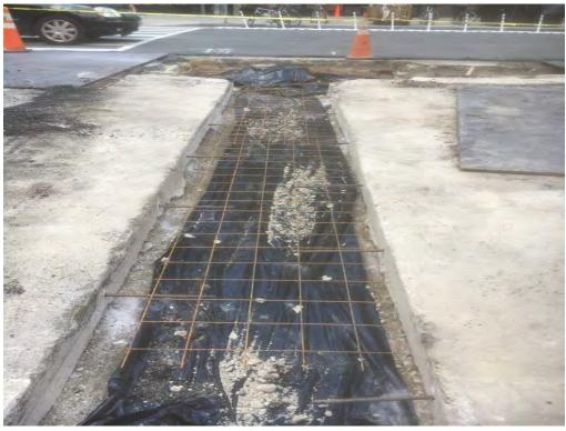
Wire mesh and Rebar prior to placement of PCC Base on Wallach St.
