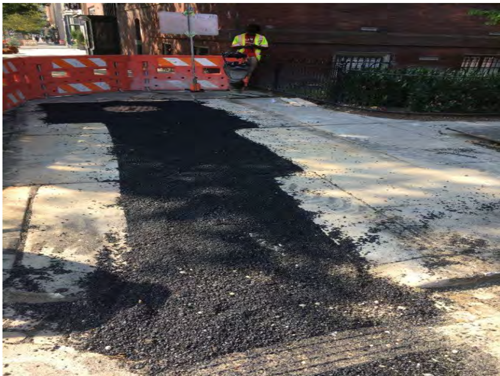
Placement of Temporary Asphalt over electrical trench in sidewalk
