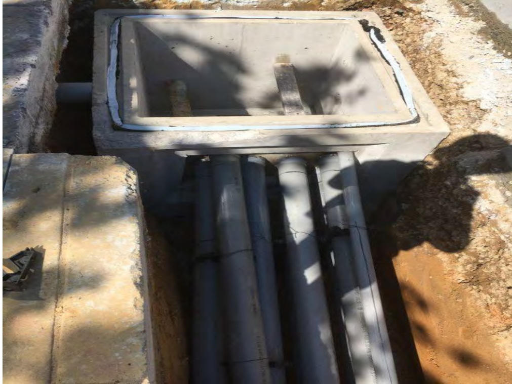
Installation of 4" and 2" PVC Conduit into 3' Manhole
