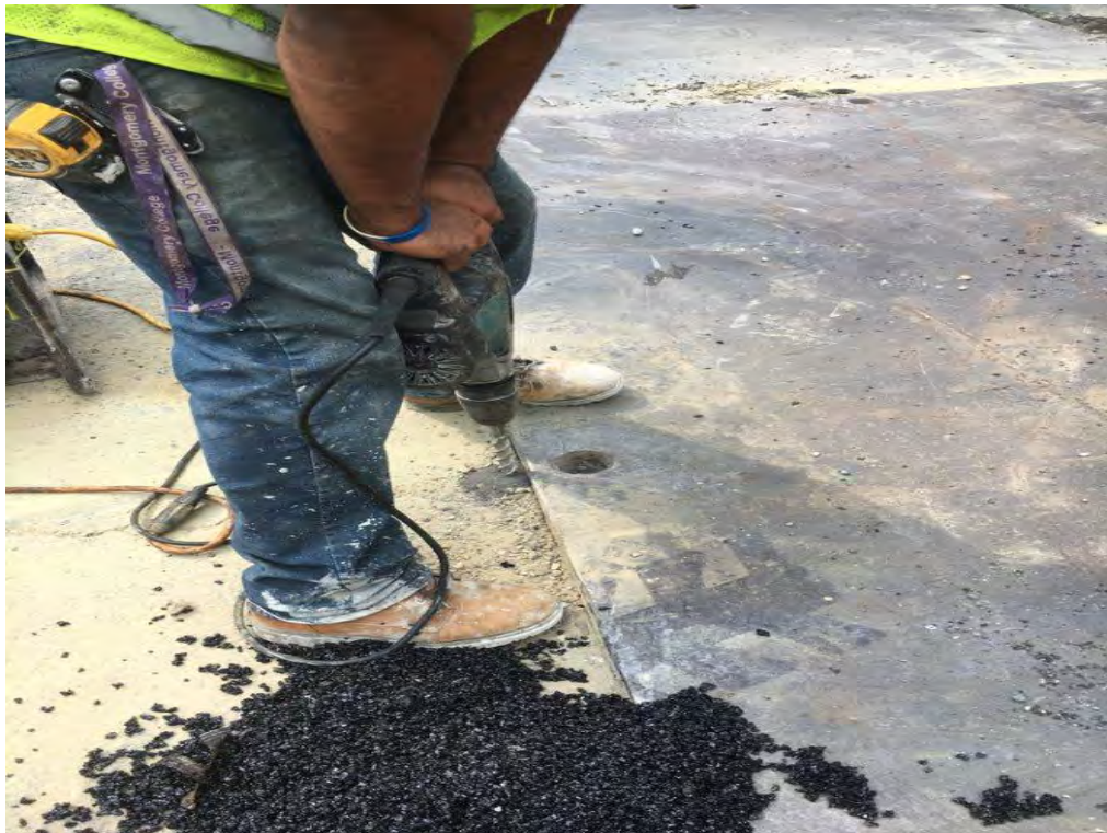
Contractor Pre-drilling prior to pinning the Steel Plates
