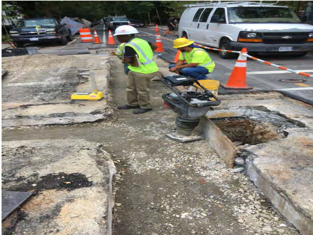
Compaction Test of GAB material prior to PCC Base placement
