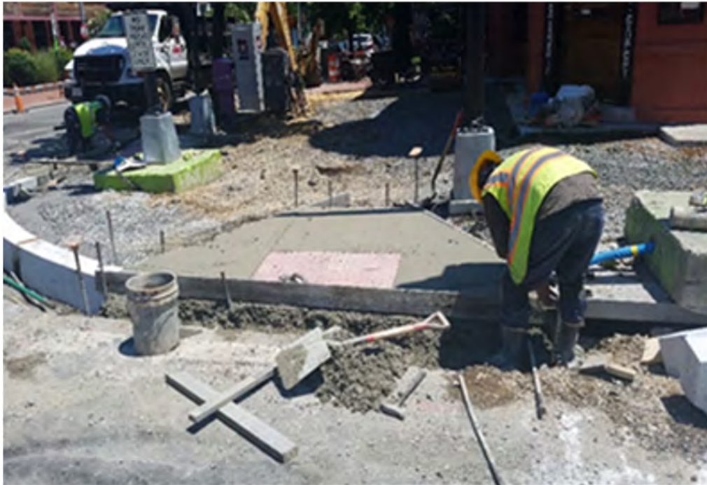
PCC concrete placed at bicycle/wheelchair ramp at T St.
