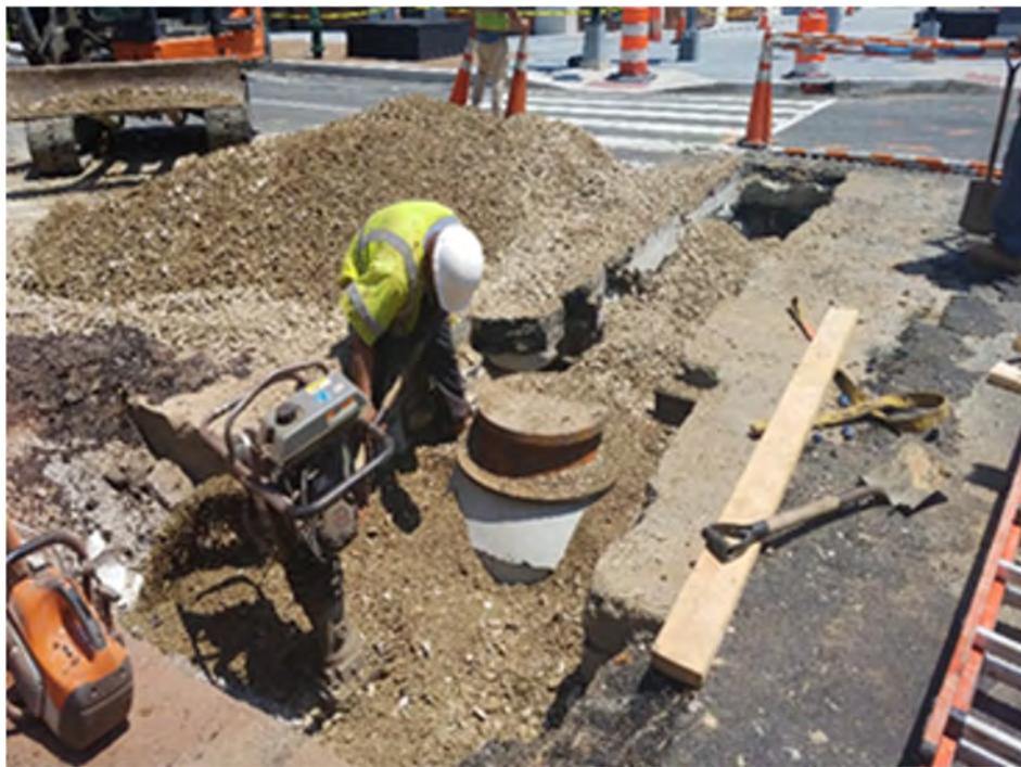
Valve Casing installed at gate valve.
