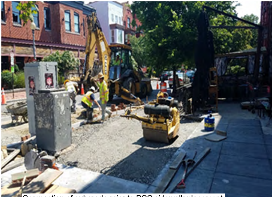
Compaction of subgrade prior to PCC sidewalk placement.
