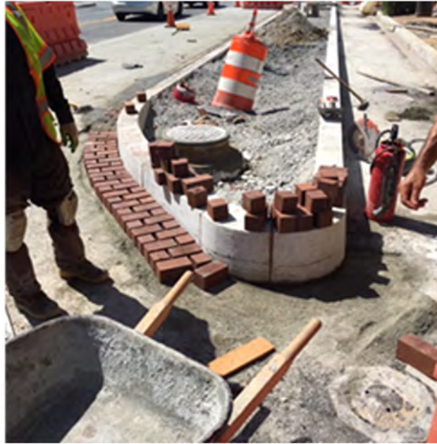
Brick Gutter installation
