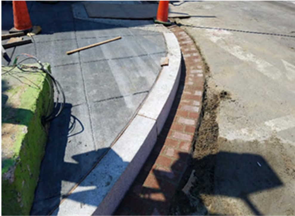
Brick gutter placed at SEC of 14 th & T St.
