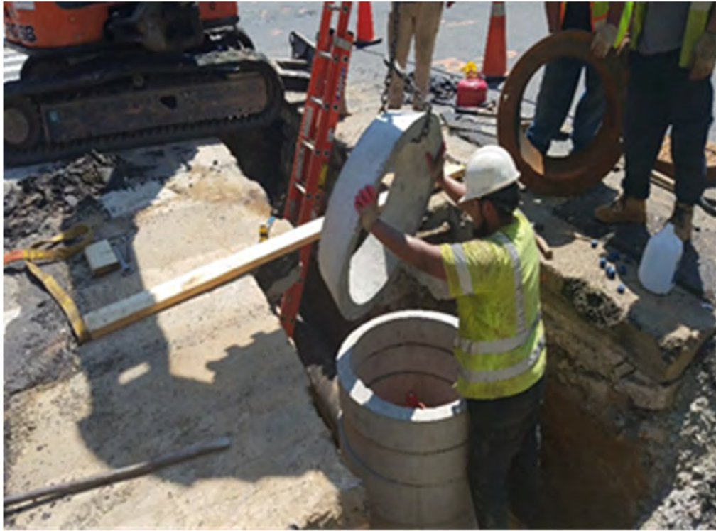
Valve Casing installed at gate valve.
