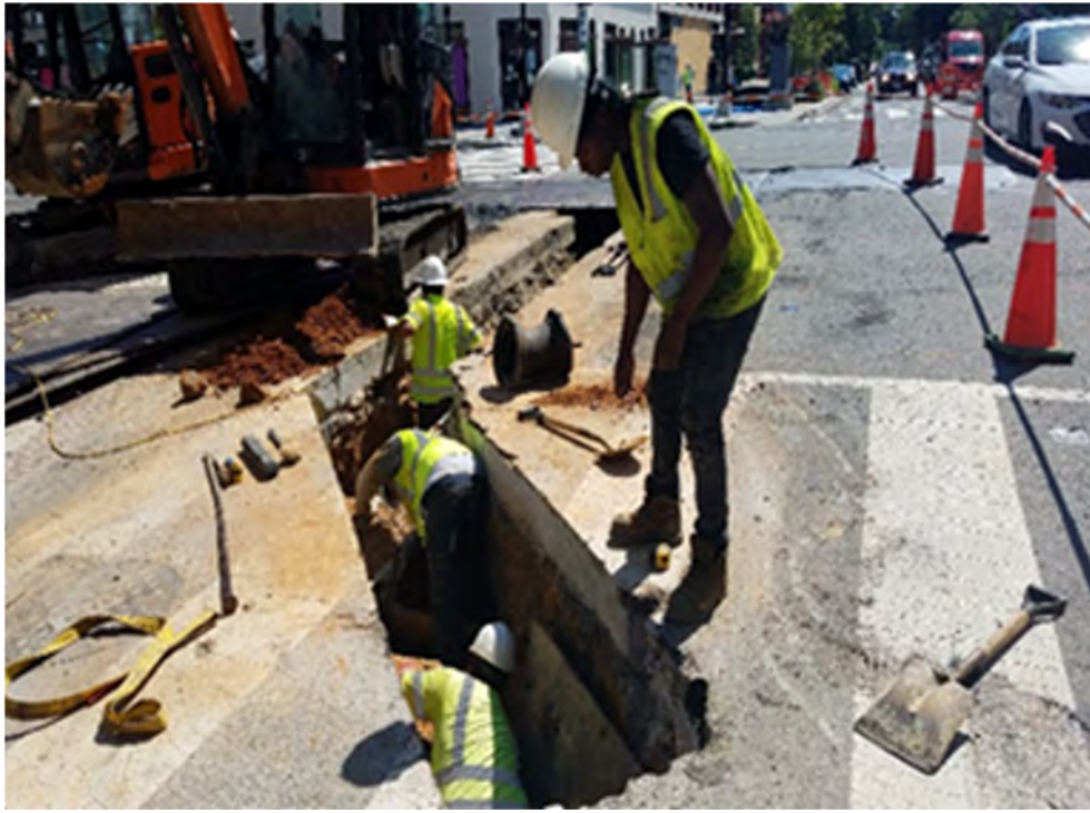
Excavation at 8" main underway at westbound R St
