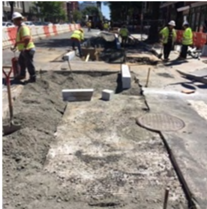
Curb Installation Preparation at Bus pad Island
