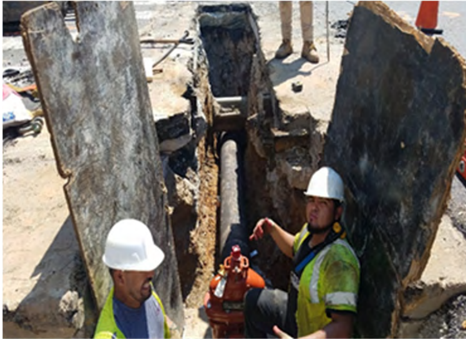
12" gate valve and 2 sections of 12" D.I.P. connected
