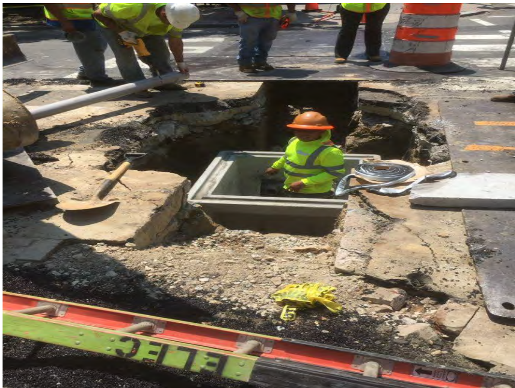
Installation of Manhole on T Street on the Eastside
