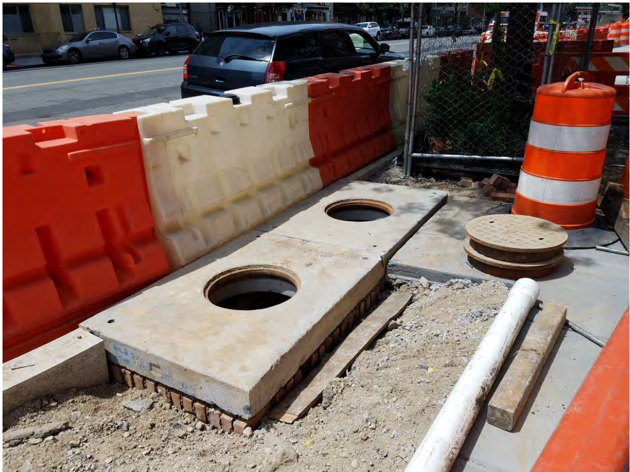
Adjusting Catch Basin Top between N Street and Rhode Island Ave Eastside
