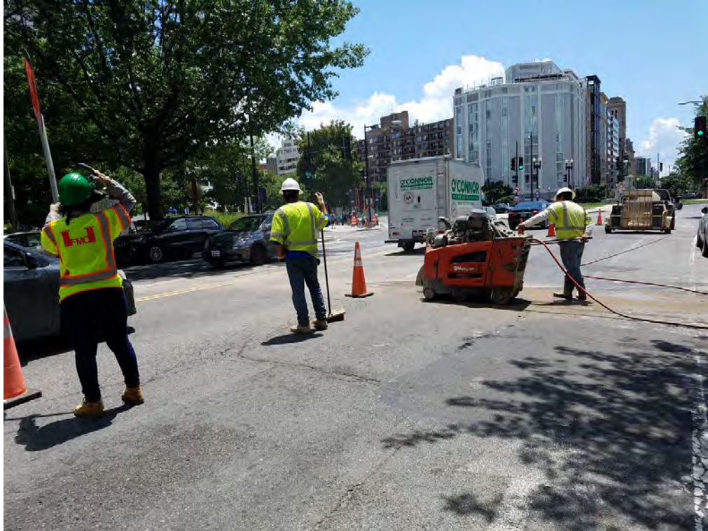
Saw Cutting between Thomas Circle and N Street on the Westside
