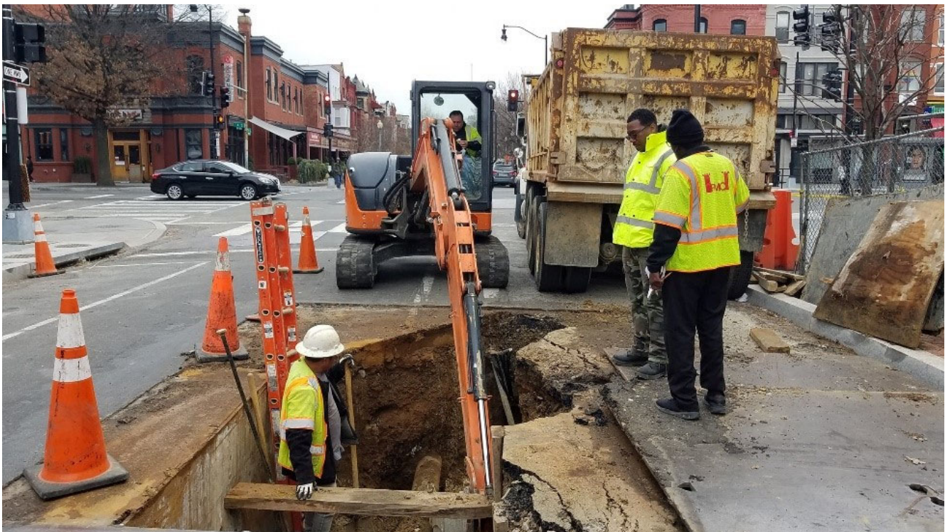
Omni was preparing for chlorination test and flushing at T Street
