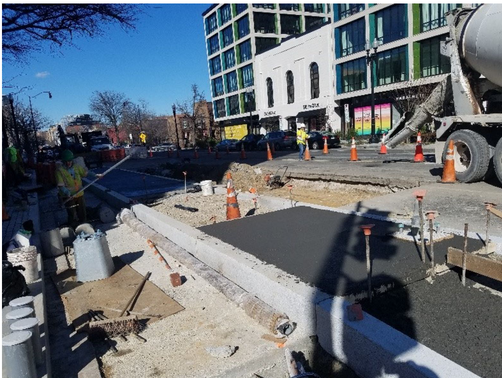
Finishing of concrete completed by FMCC
