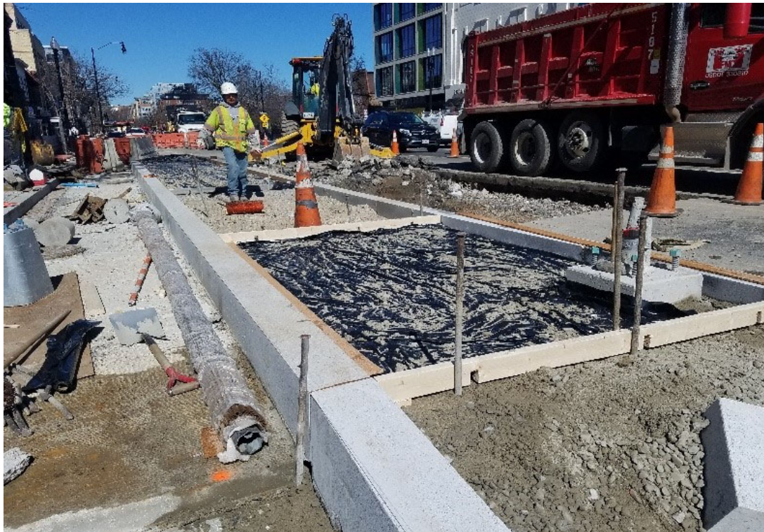
Aggregate base course placed and compacted by FMCC
