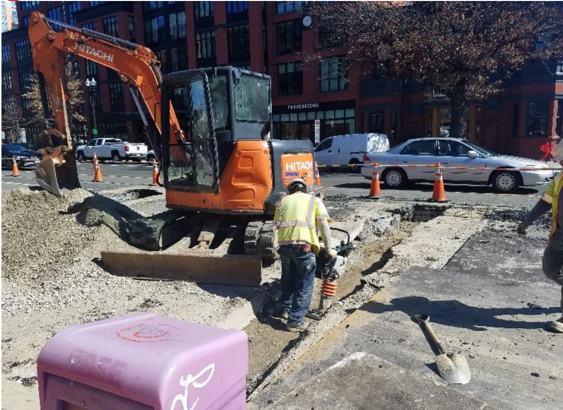
Backfill of trench at 1902 14 th St by Omni Excavators
