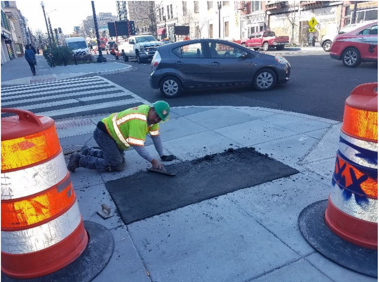
PCC sidewalk repaired following pole base removal at Riggs St.
