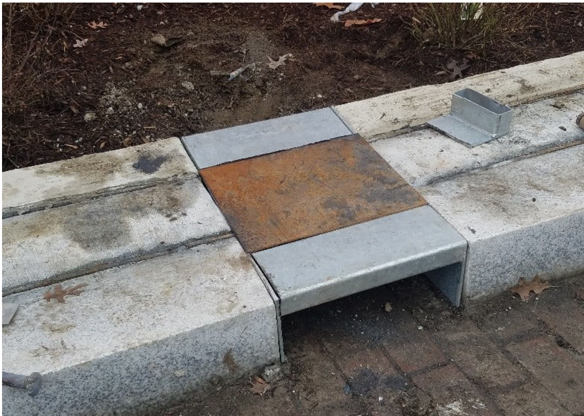
D.E.N. onsite placing grates at bio-retention planter near S St
