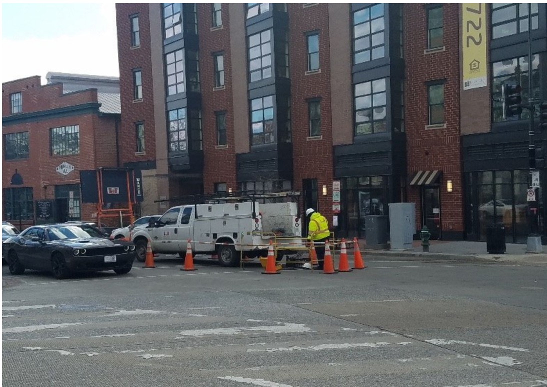
Electrical crew working splicing cable at electrical manhole M106.
