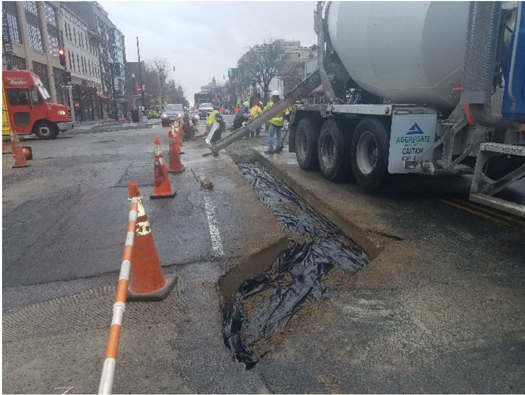
PCC base placement at backfilled water main trench
