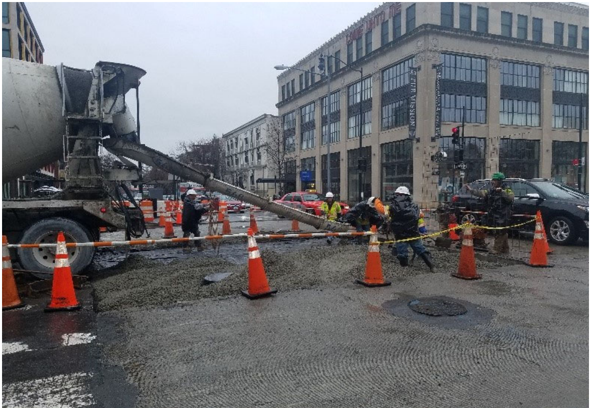
PCC Base concrete placement underway
