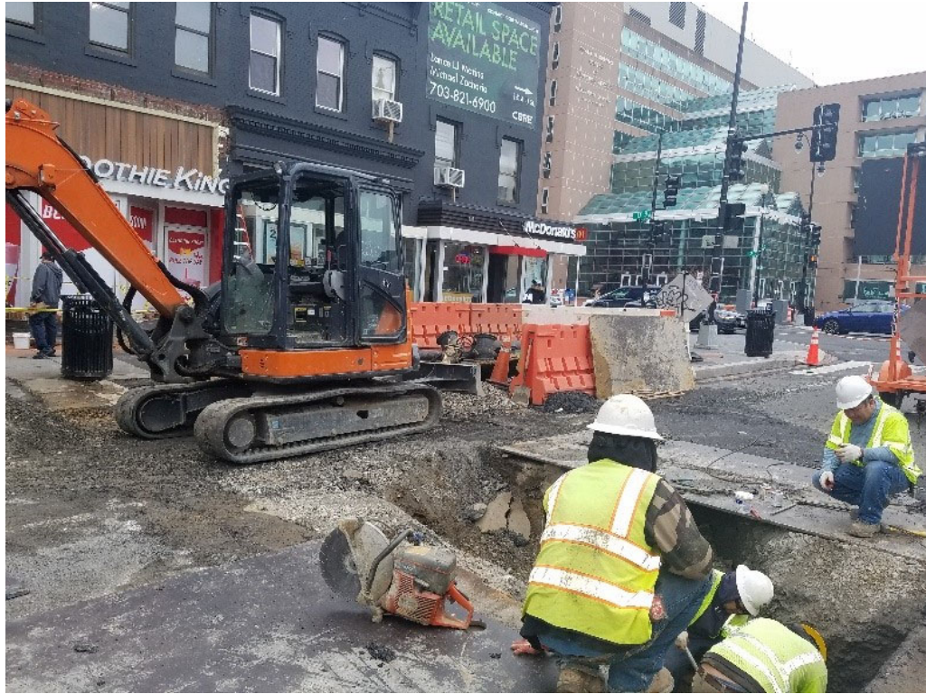
1" service connection by Omni underway.
