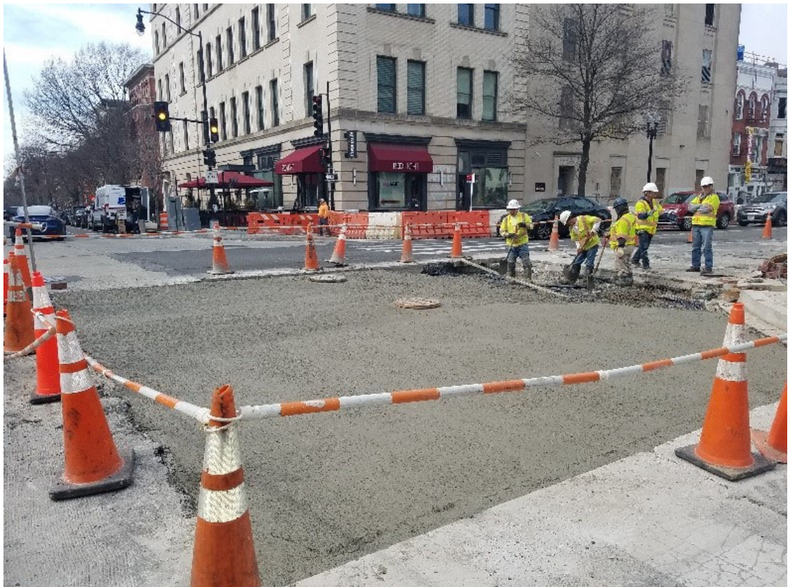
Placement of Class C concrete base underway
