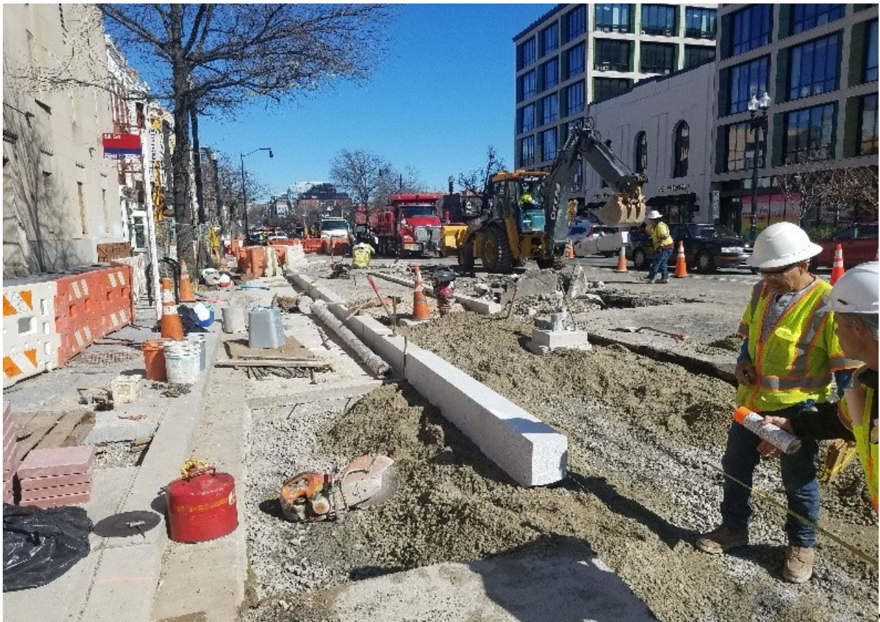
FMCC civil crew installing straight granite curb.
