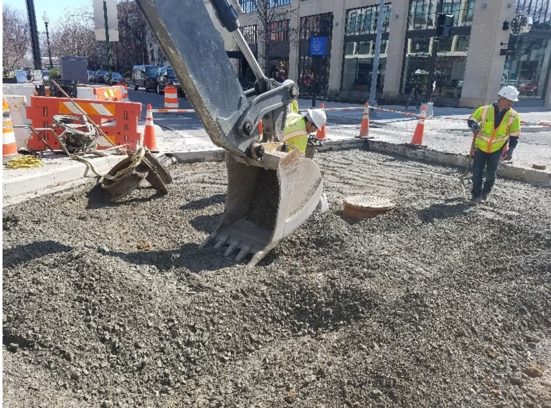
Aggregate base course placed prior to PCC concrete base placement
