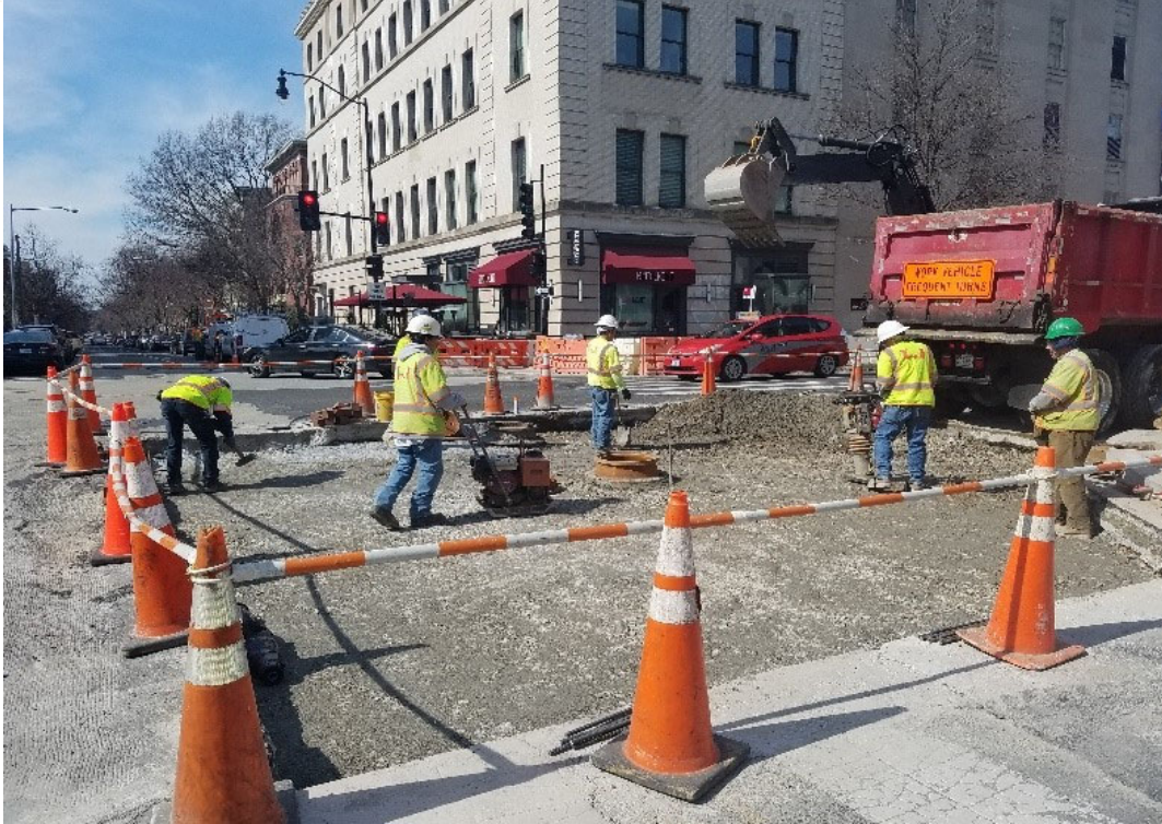
Compaction of subgrade underway by FMCC civil crew
