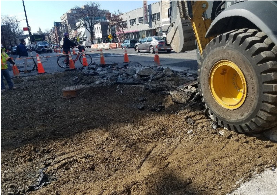
FMCC Civil crew demolishing NEC of 14 th & R St roadway
