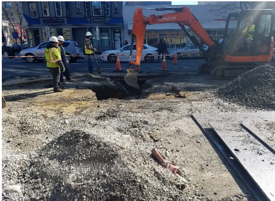
Omni Excavators backfilling water main at SWC of 14 th & U St
