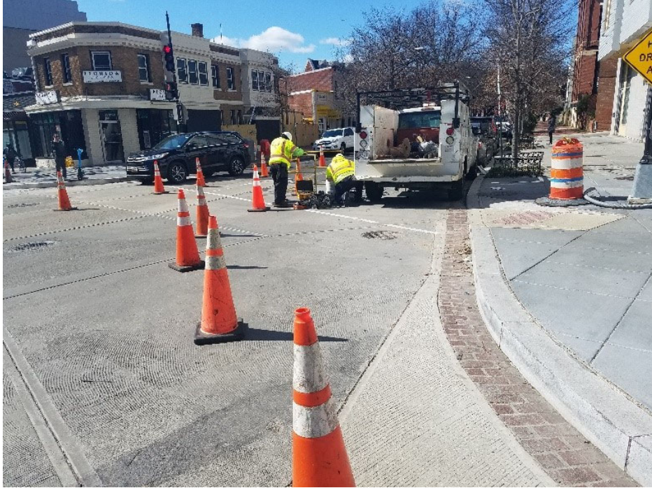
Electrical crew working splicing cable at electrical manhole M101.
