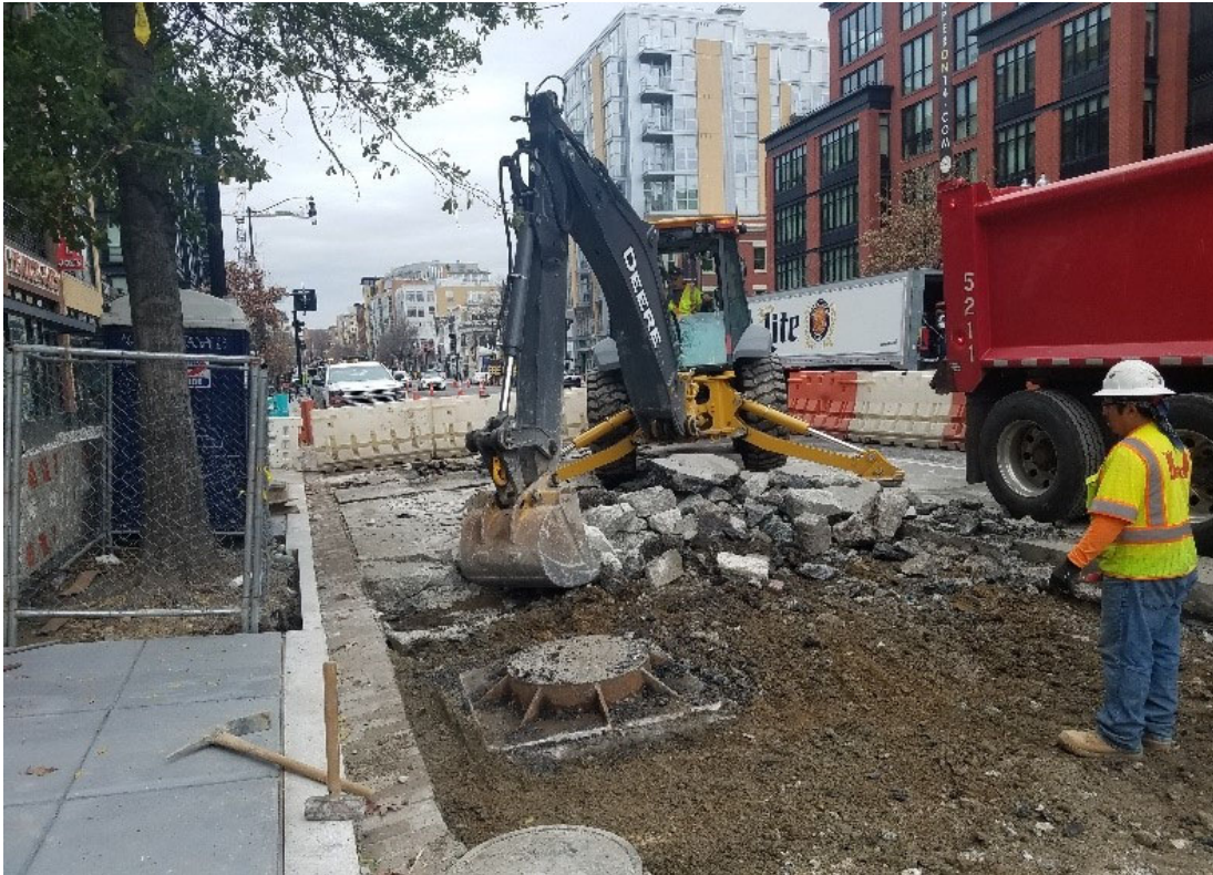
FMCC civil crew removing roadway materials via backhoe and dump truck.
