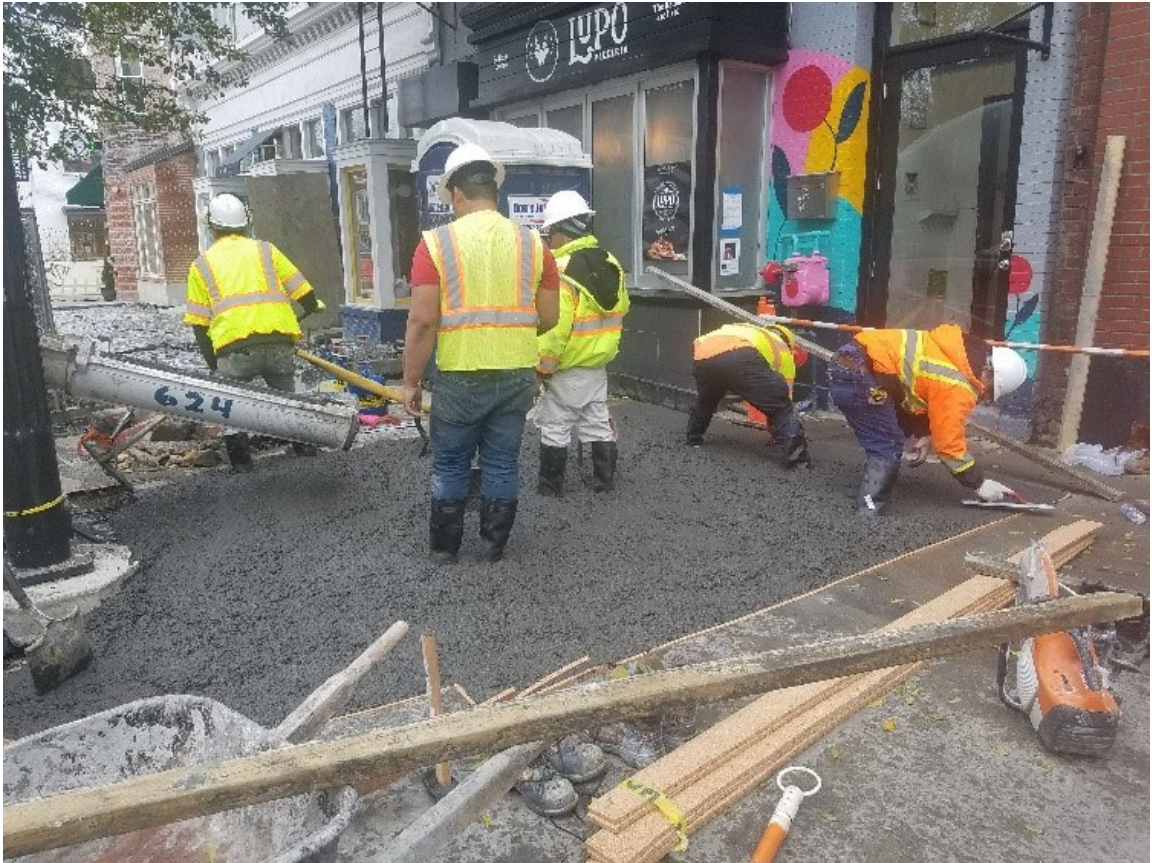
D.E.N. placing PCC sidewalk near 1908 14 th St
