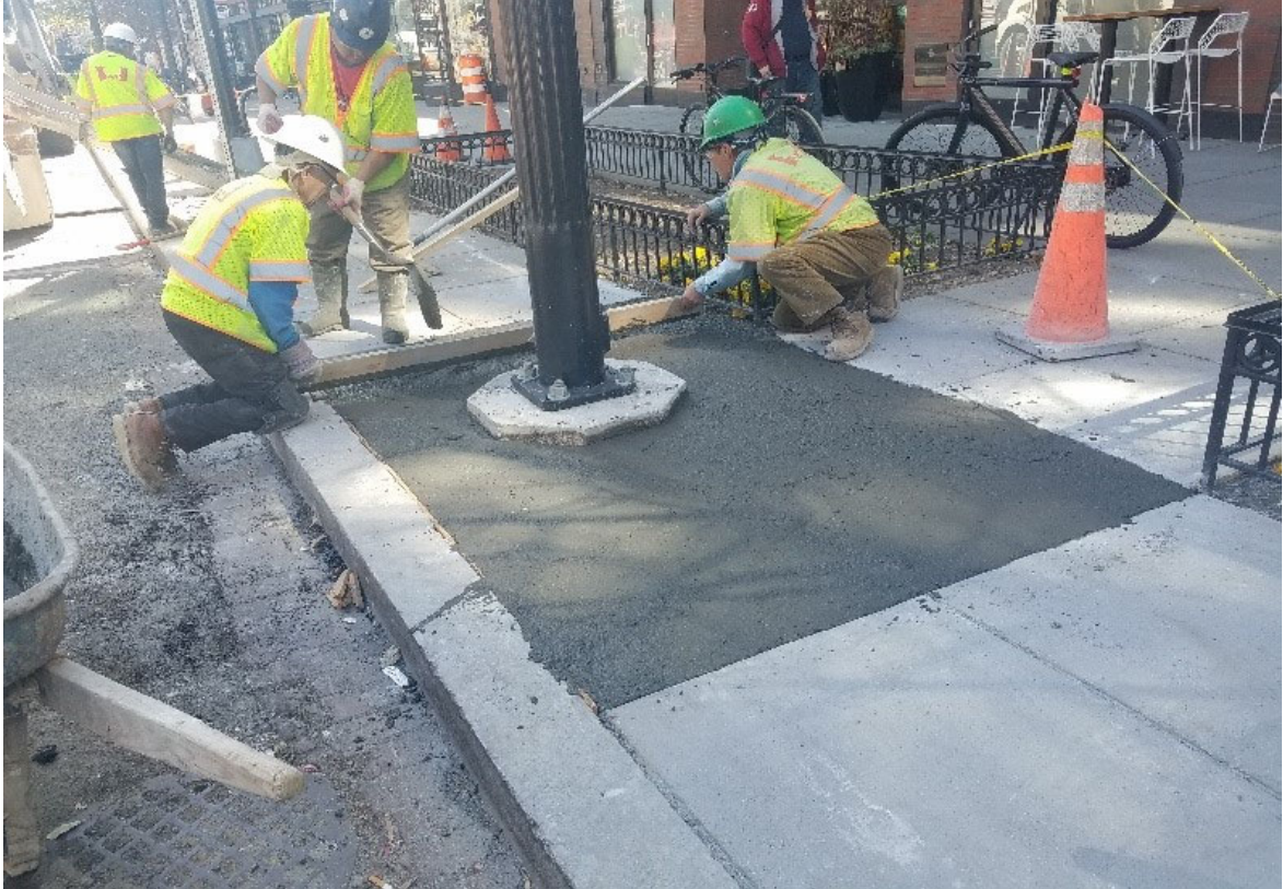
PCC Sidewalk repaired by FMCC Civil crew
