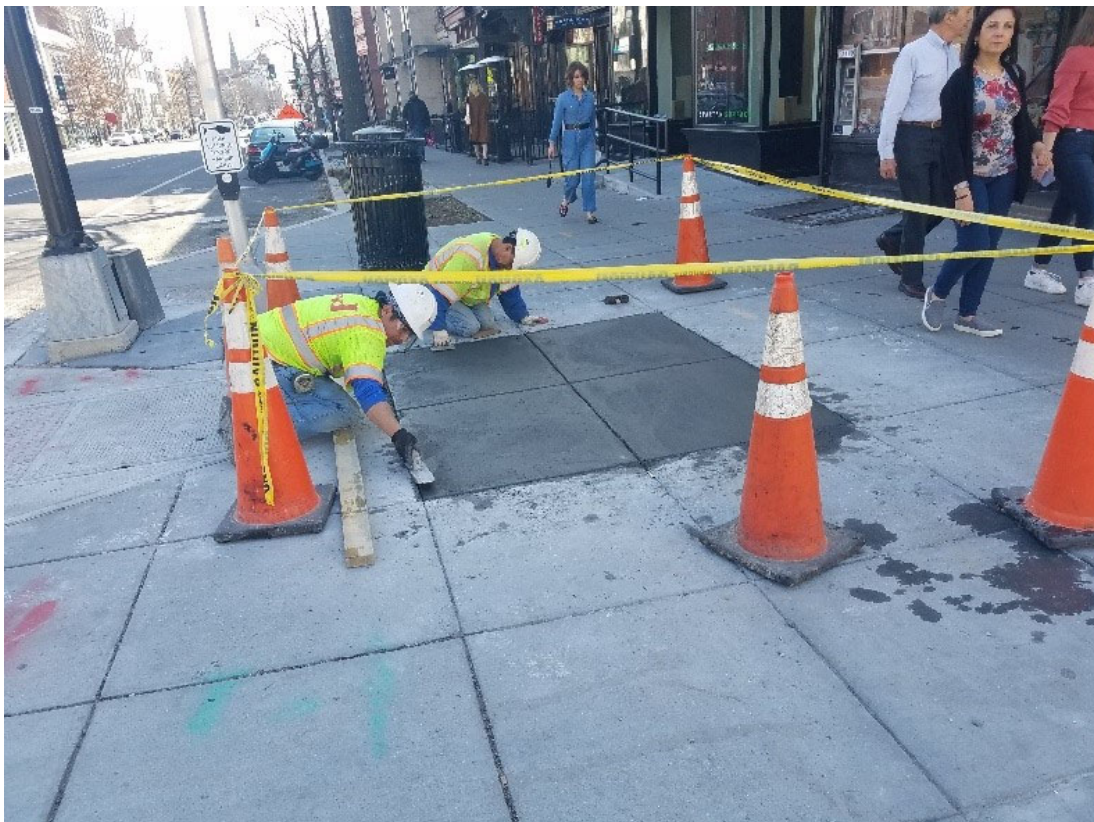
Sidewalk repaired by FMCC Civil crew following light pole foundation removal.
