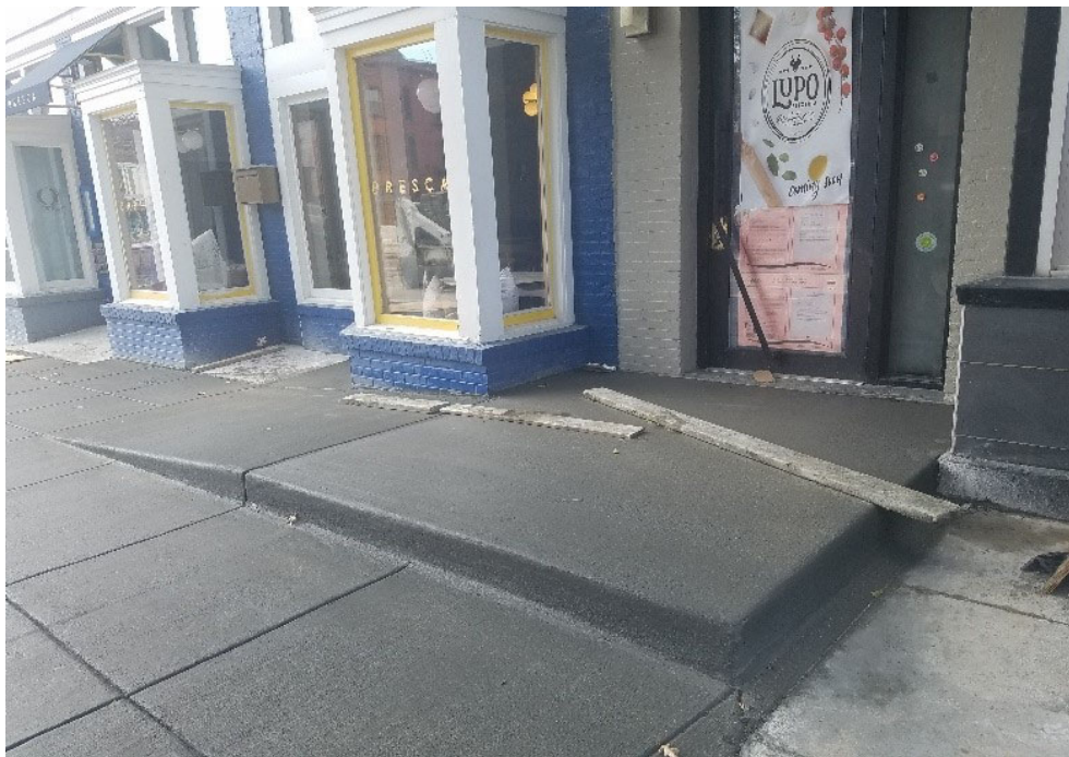
Building ramp placement near 1908 14 th St
