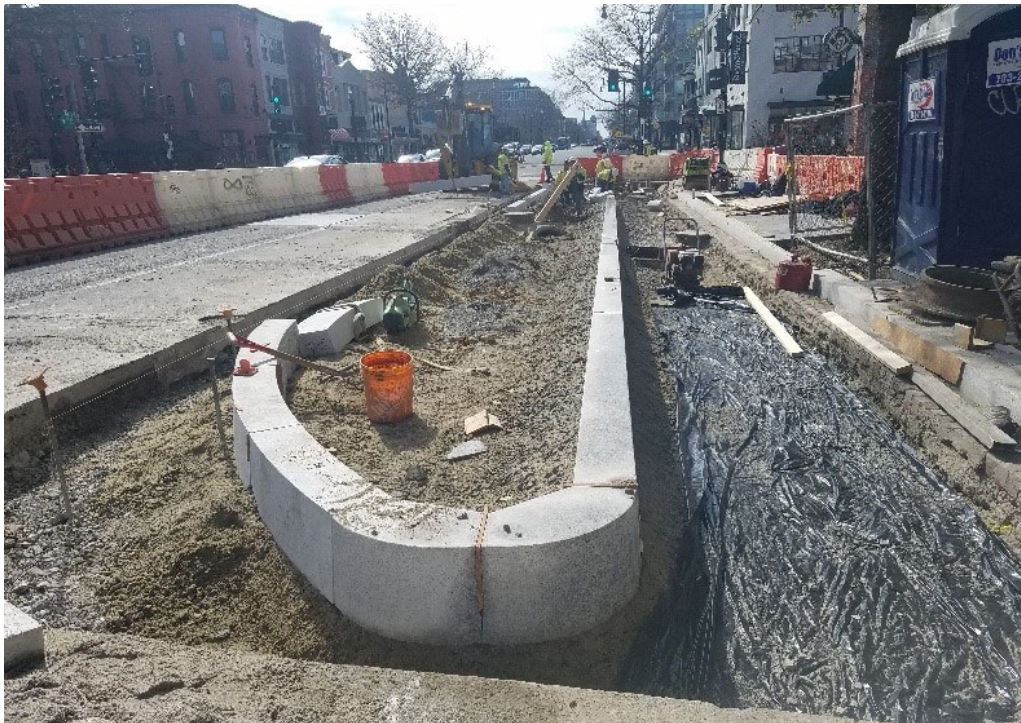
FMCC Civil at NWC of 14 th & T St granite curb installation
