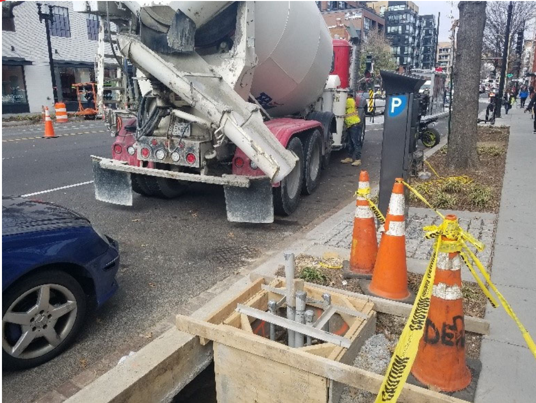
Twin pole foundation L-82 foundation prior to concrete placement
