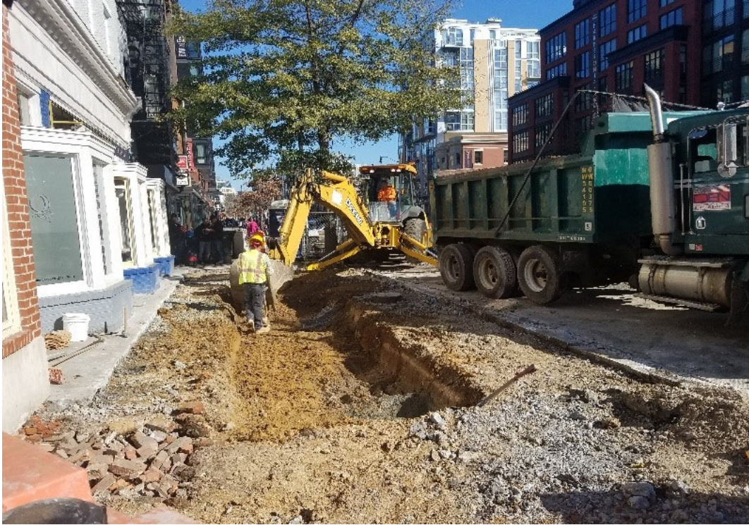
D.E.N. excavating tree zone from 1902 to 1910 14 th St
