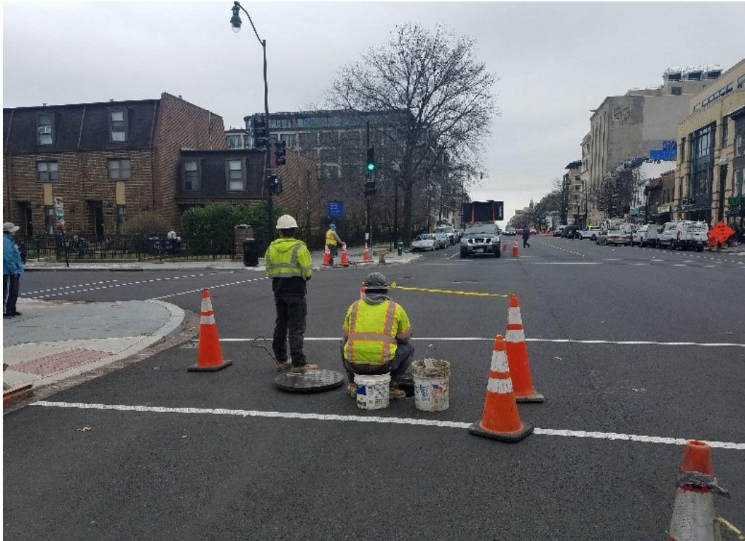
Omni Excavator crew parging traffic signal manhole at S St.
