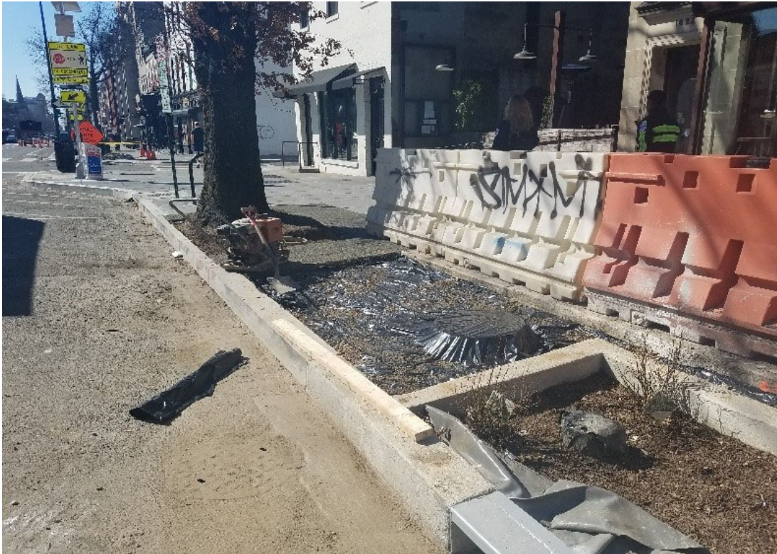
D.E.N. excavating tree zone from 1902 to 1910 14 th St
