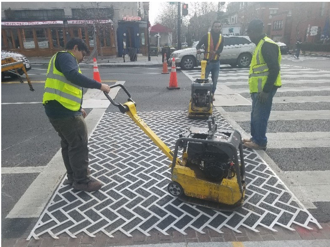
Compaction of marking grid underway
