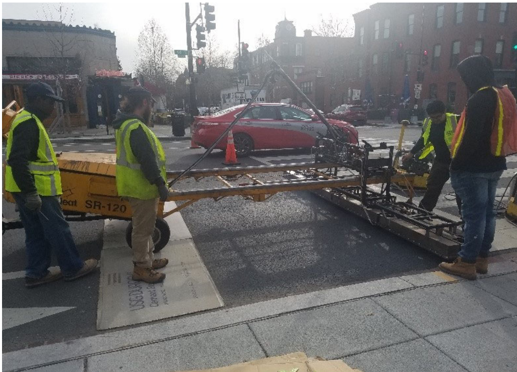
Inlaid thermoplastic marking system underway at NWC of 14 th & Q St
