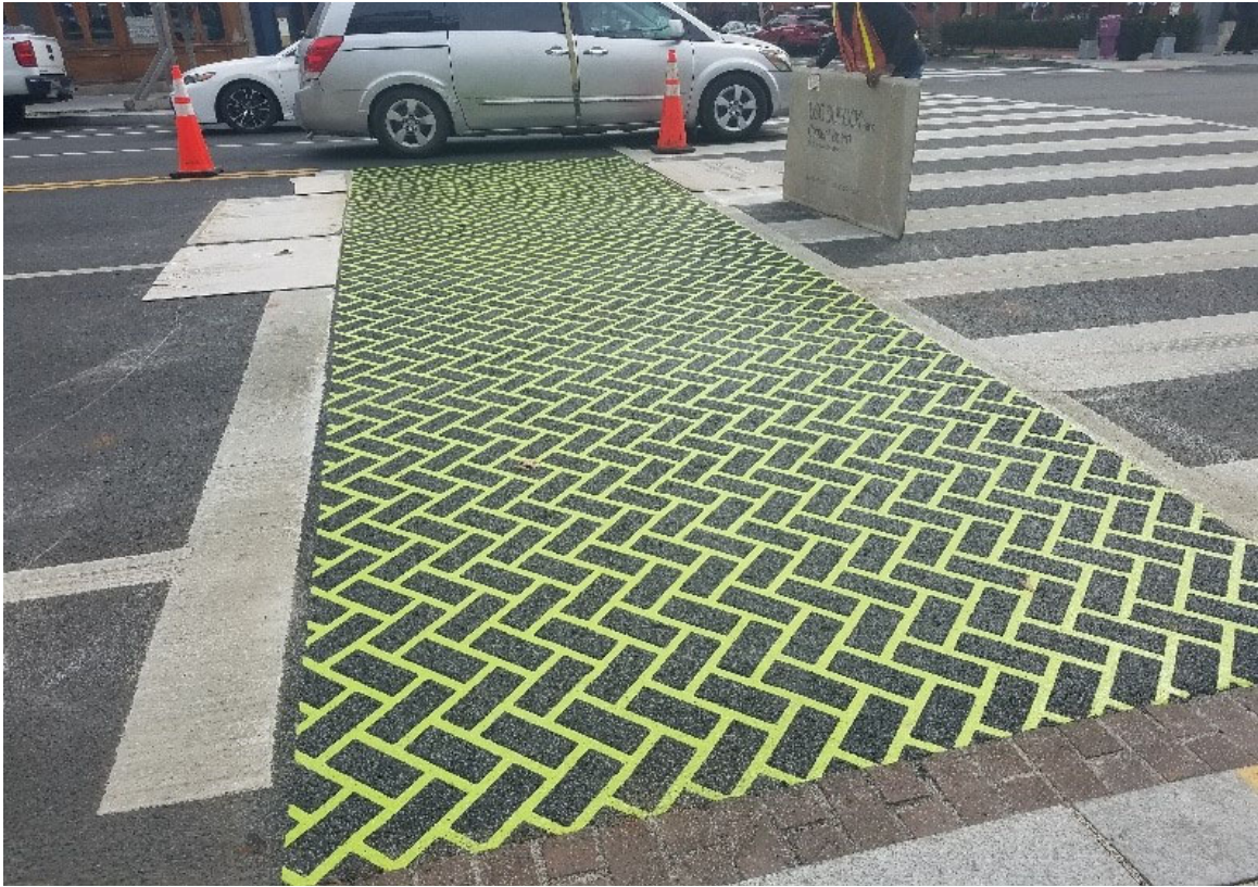
Inlaid pavement marking system completed
