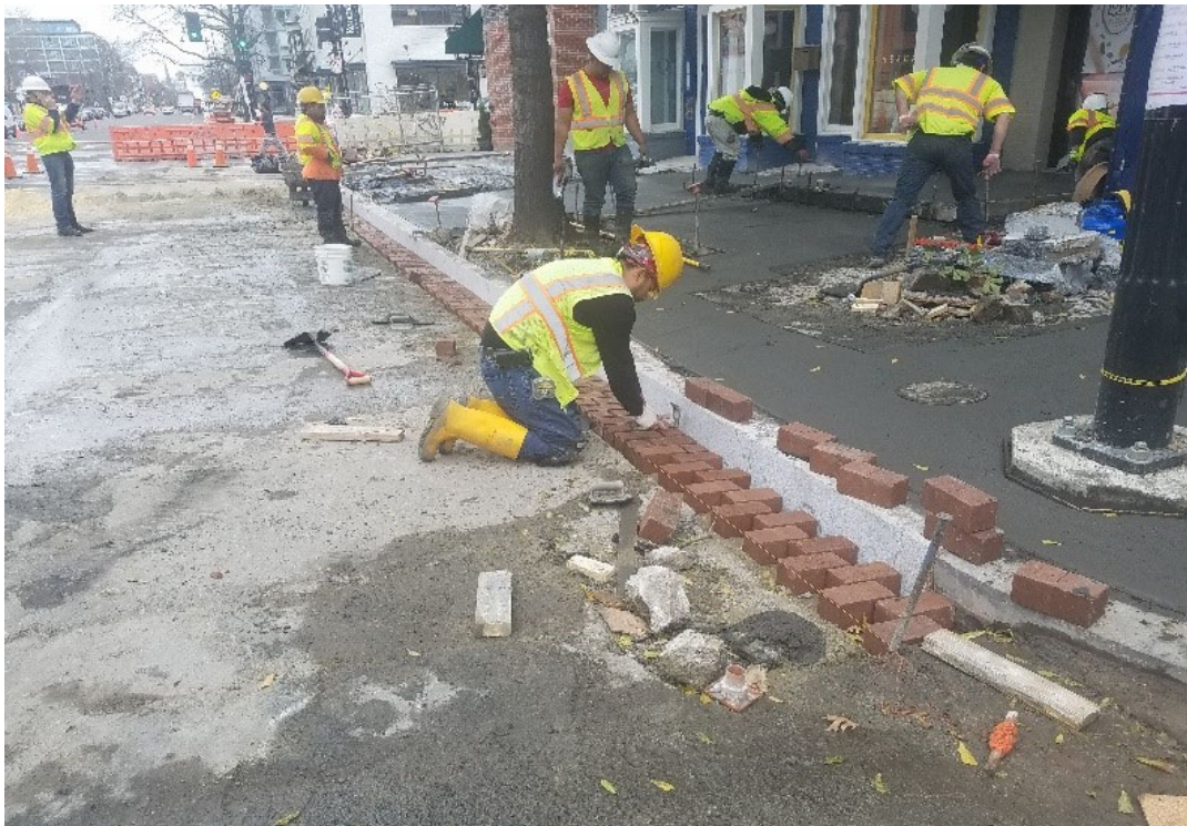
D.E.N. placing PCC sidewalk near 1908 14 th St
