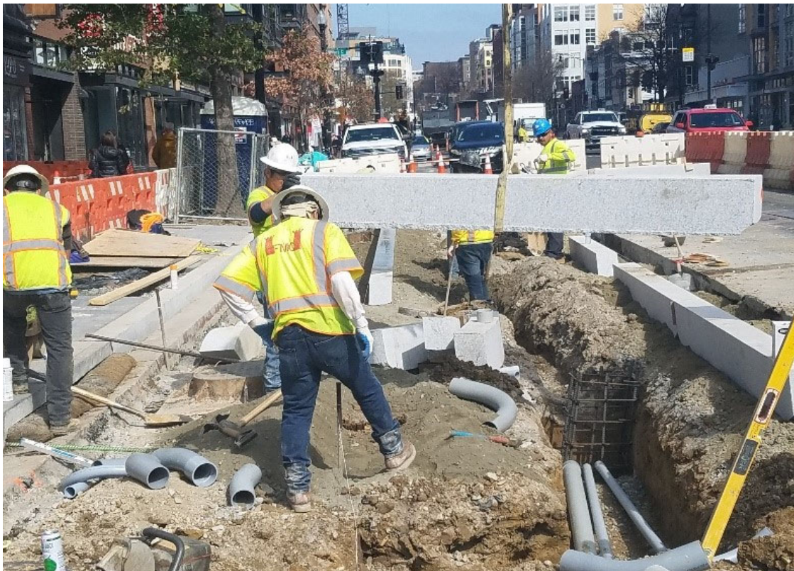
FMCC civil crew installing straight granite curb.
