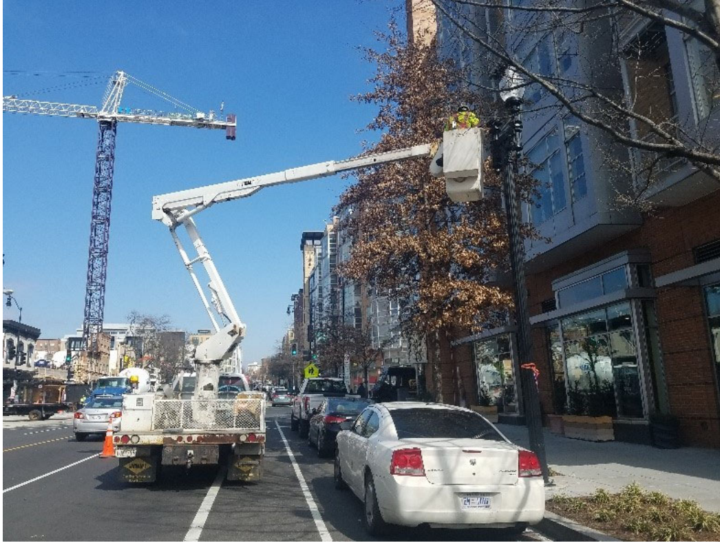
FMCC electrical crew at 2000 block of 14 th St
