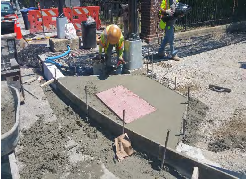
Brick gutter completed at SEC of 14 th & V St.
