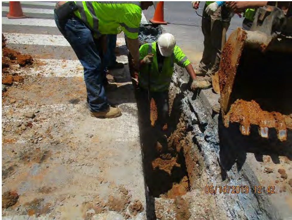
Omni continued the Installation of 8-Inch D.I.P at 14 th & R Street NW
