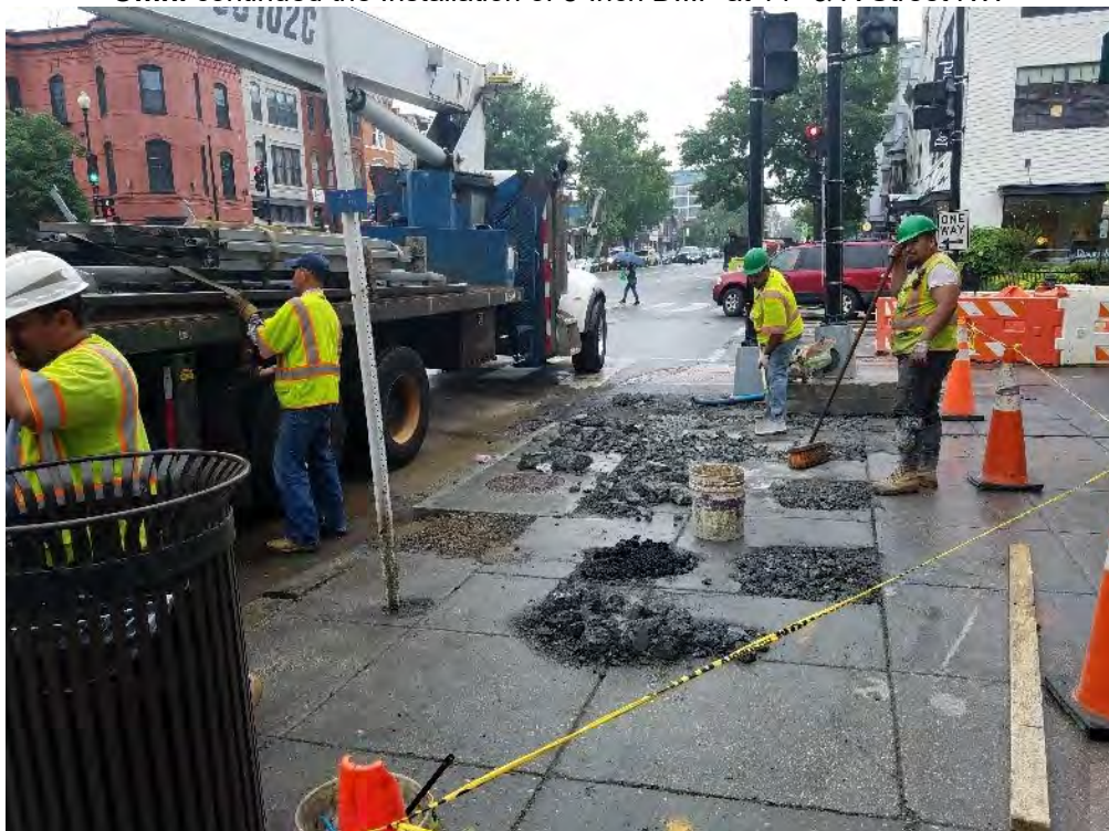
Omni continued the Installation of 8-Inch D.I.P at 14 th & R Street NW
