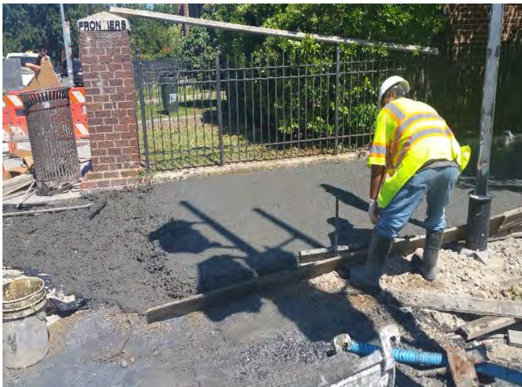
Granite curb placement placed prior to brick gutter placement
