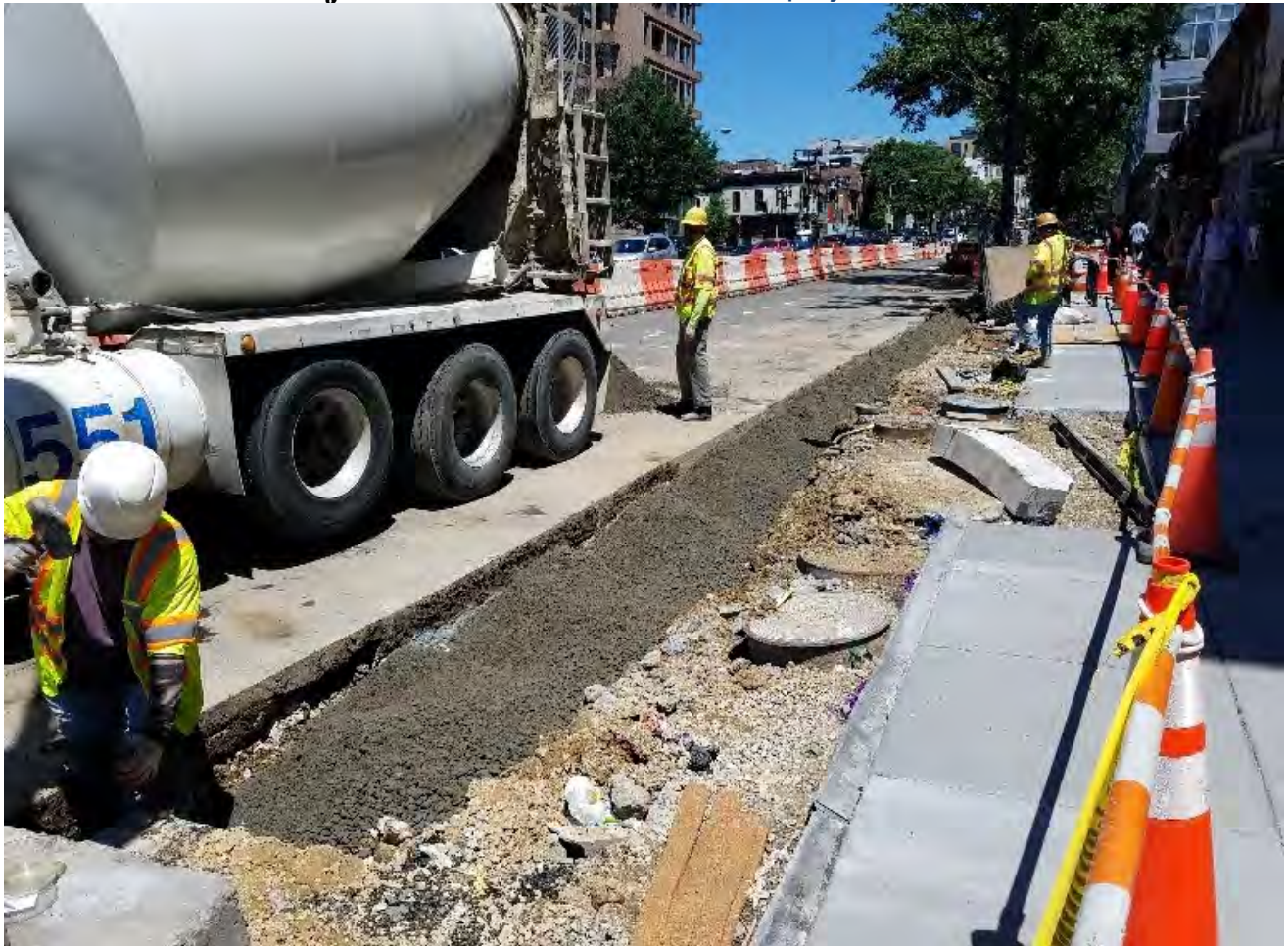
Delivery of dry mix in preparation for granite curb installation.
