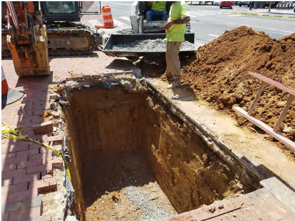
Excavation for Catch Basin at SE corner of Rhode Island Ave
