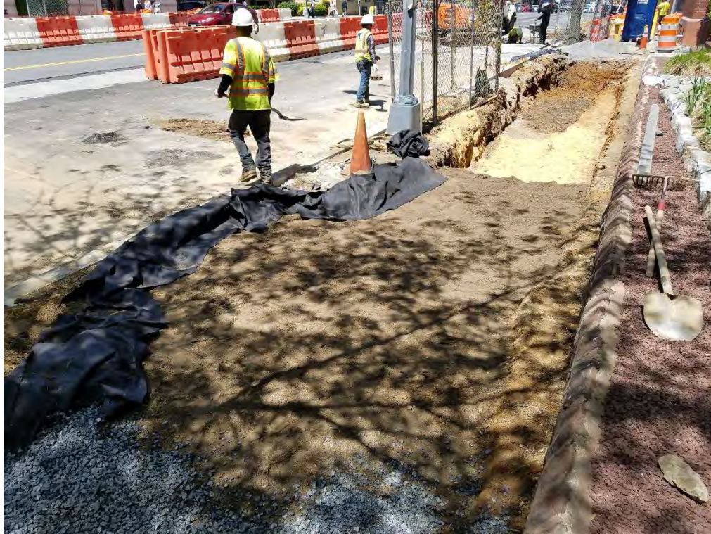
Placement of the Structural Soil between Thomas Circle and N Street Eastside
