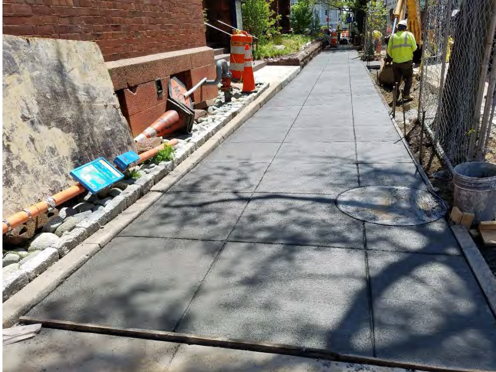
PCC Sidewalk between Thomas Circle and N Street Eastside
