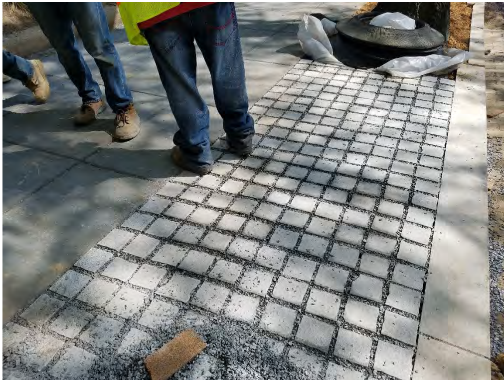
Placing Granite Cobble Stone between Thomas Circle and N Street Eastside
