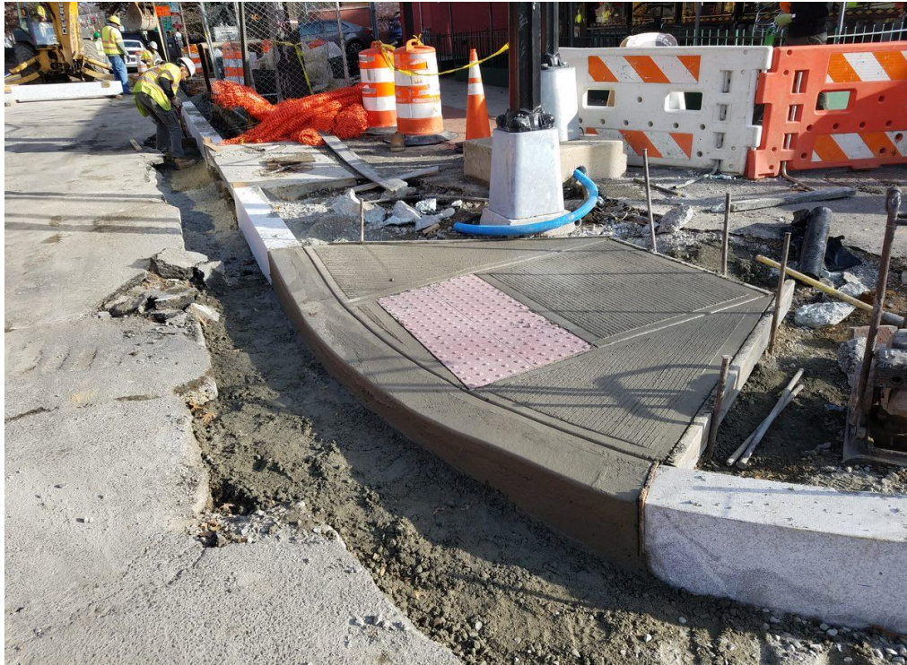
Placing ADA Ramp at the SE Corner of 14 th and P Street
