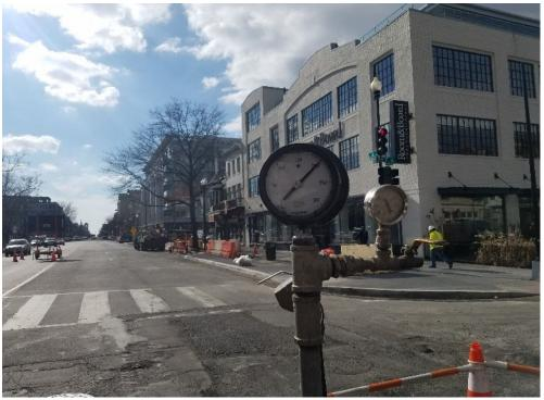
Pressure gauge maintained for 2 hours at 200 psi
