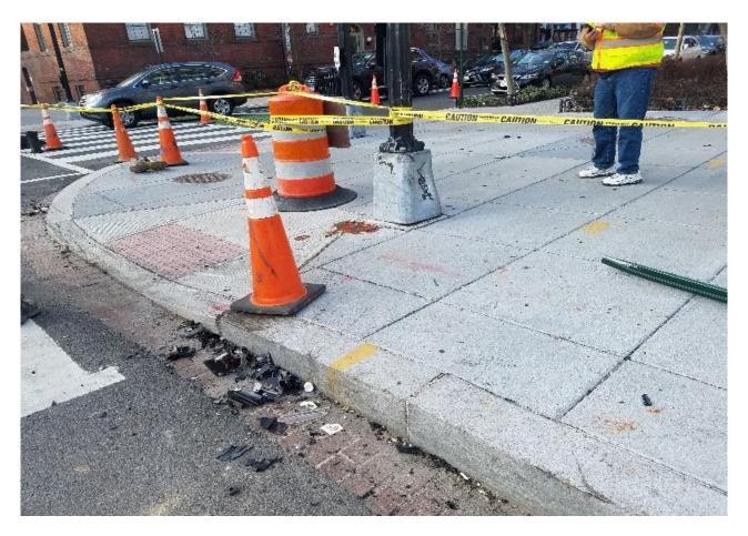
Traffic signal foundation, base and pole TS-21 damaged by car at NWC of 14th & Q St
