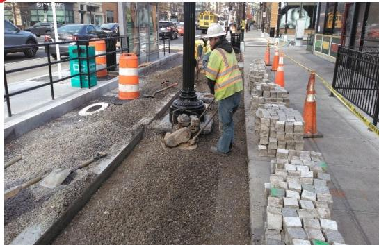
DEN compacting the bedding stone for the Permeable pavers after installing the geo grid at 1412 14th Street NW
