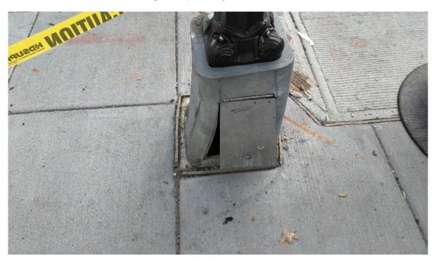
The damage to the light pole base and foundation from the accident at NW corner of Q Street & 14th Street NW
