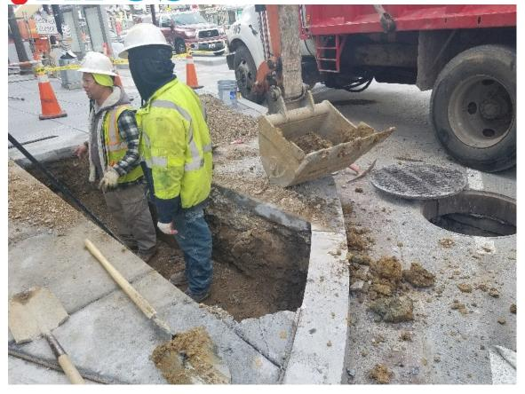
Omni installing 15 LF of 2" PVC conduit from Pepco vault (P16) to streelight manhole M106
