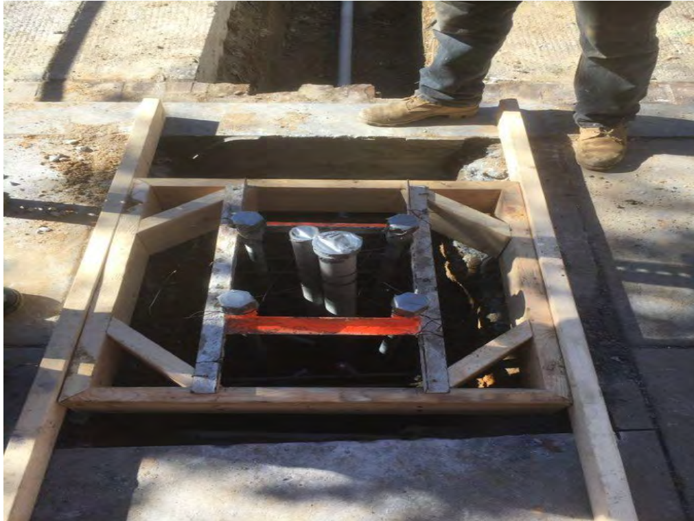
Formed Street Light Foundation
