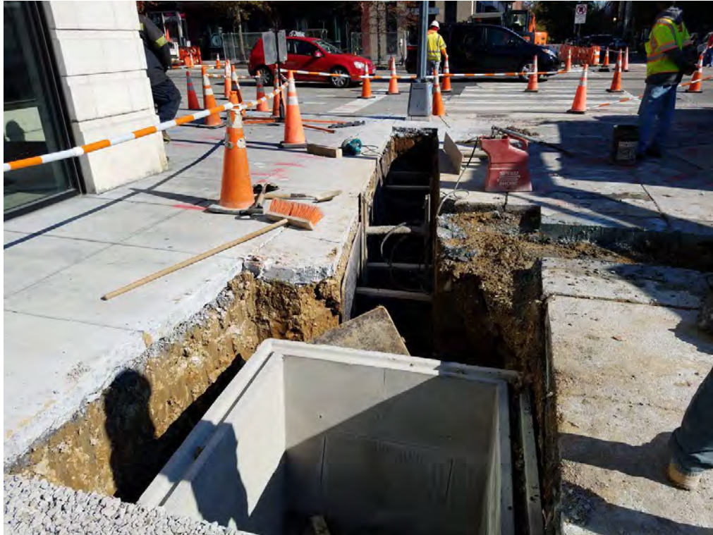
Installation of manhole at the NW Corner of W Street
