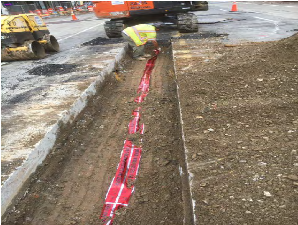
Backfill of Encased Electrical Trench and placement of Electrical Tape
