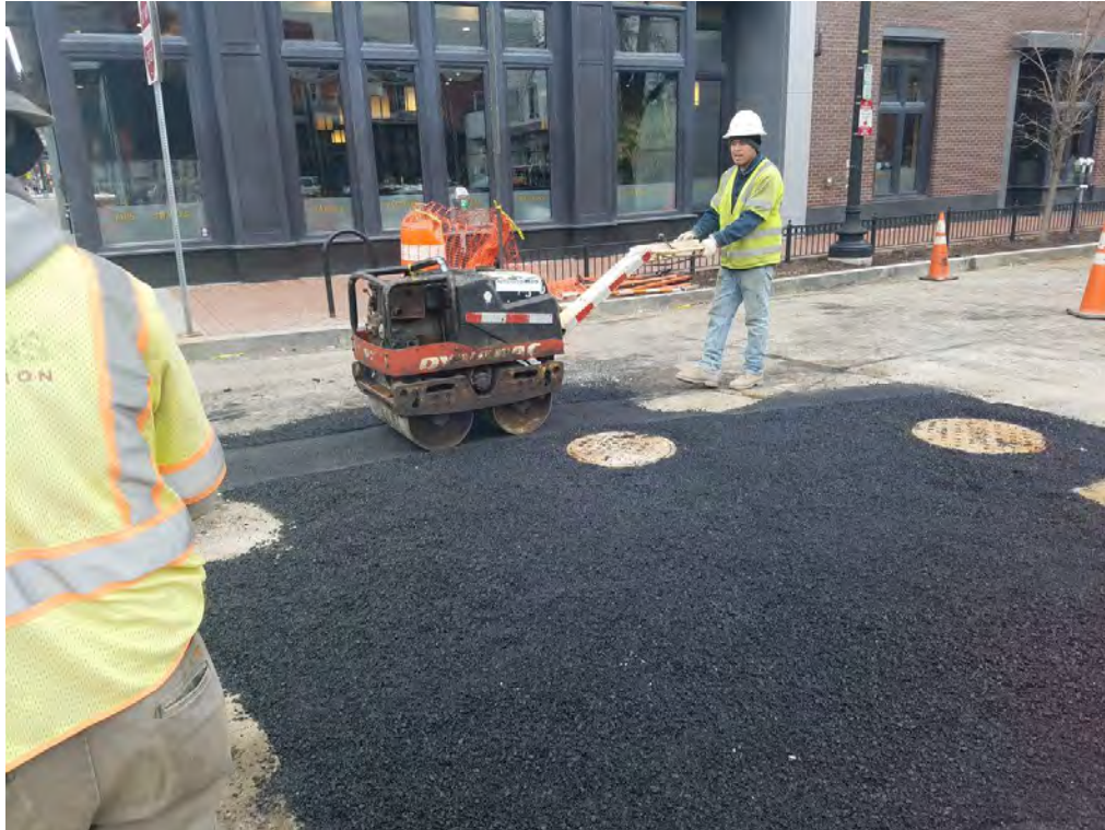
Placement of Temporary Asphalt
