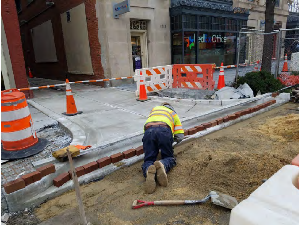
Installation of Brick Gutter at 1508 14 th Street
