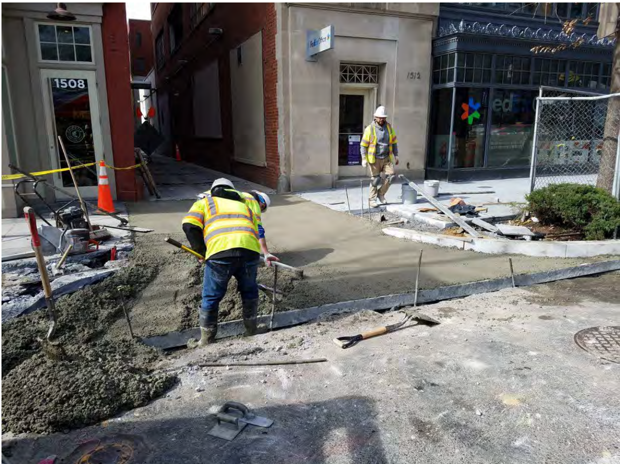
Installation of New Driveway Entrance at 1508 14 th Street
