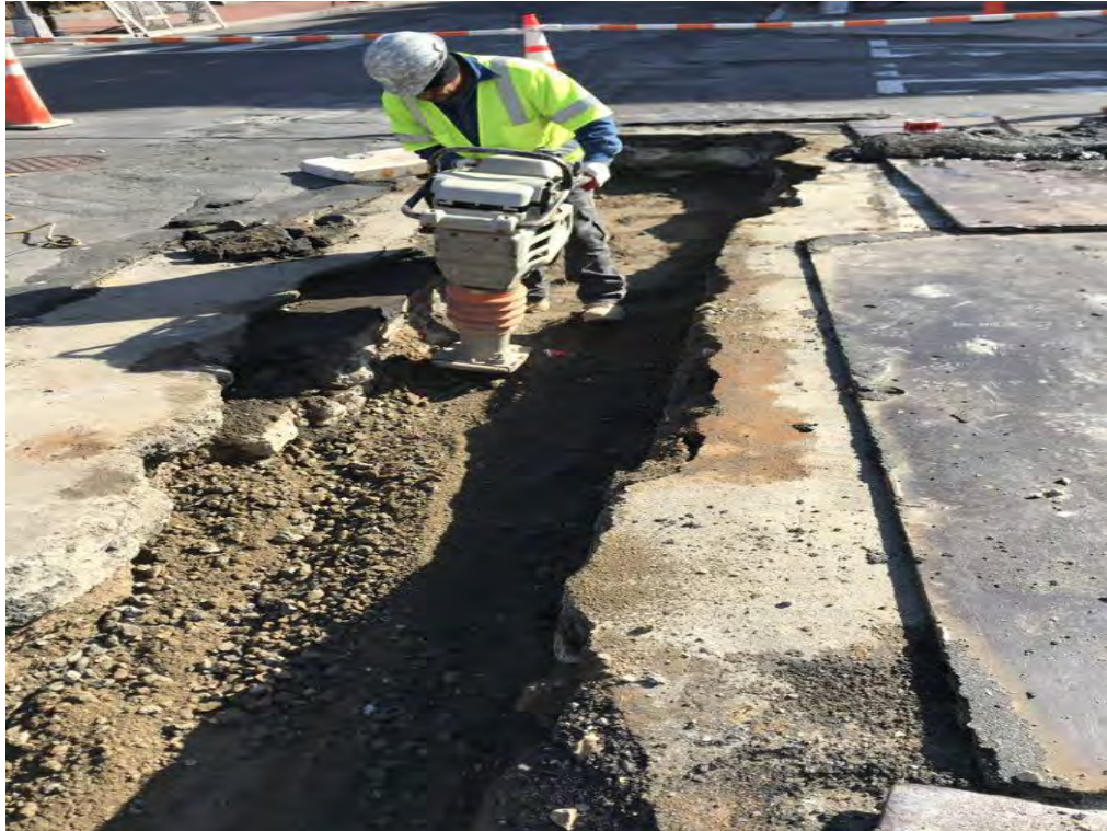
Compaction of RC6 material used for Backfill
