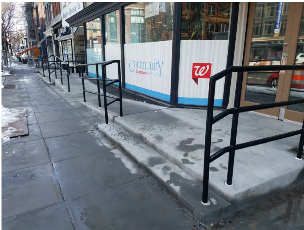
Handrail at the Newly installed ADA Entrance Ramps
