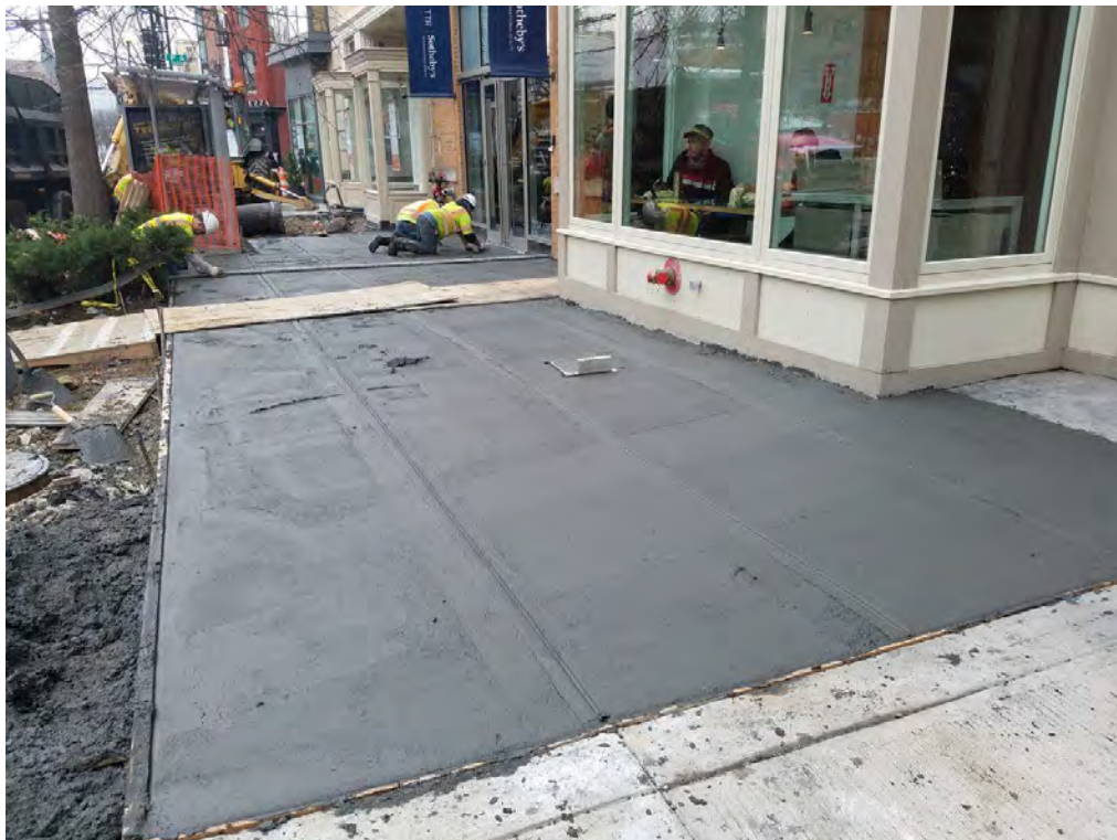
Installation new PCC Sidewalk
