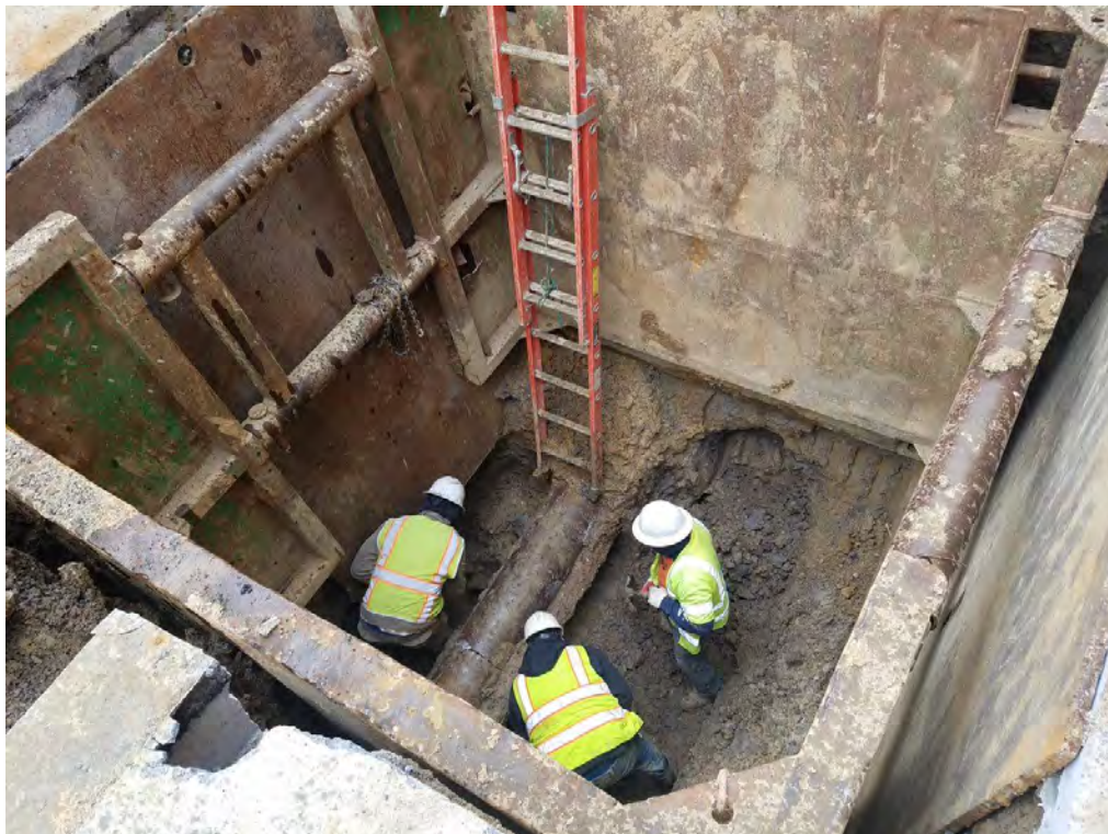
Digging around Combine Sewer line for installation of New Manhole
