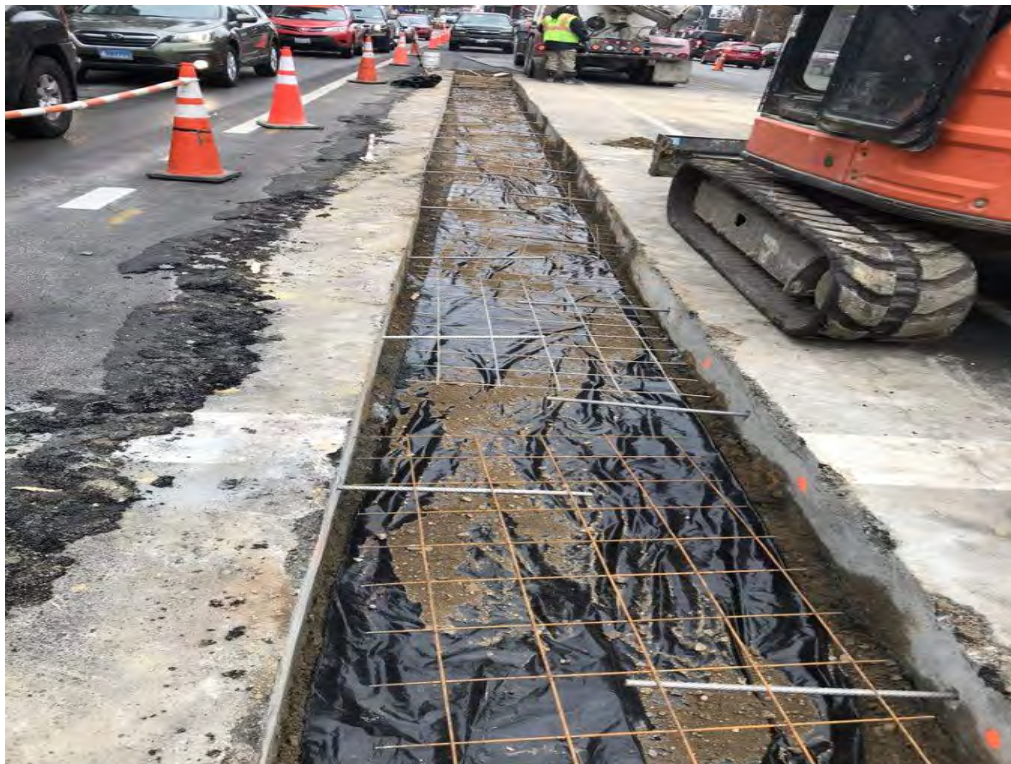
Placement of PCC Base between V Street and U Street
