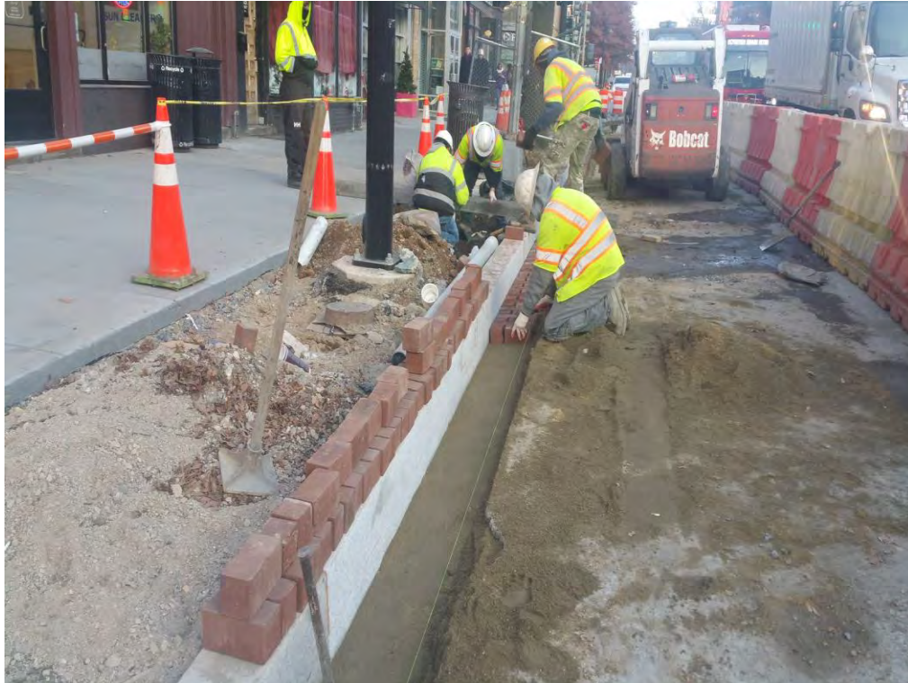
Installation of Brick Gutter Between Rhode Island and P Street
