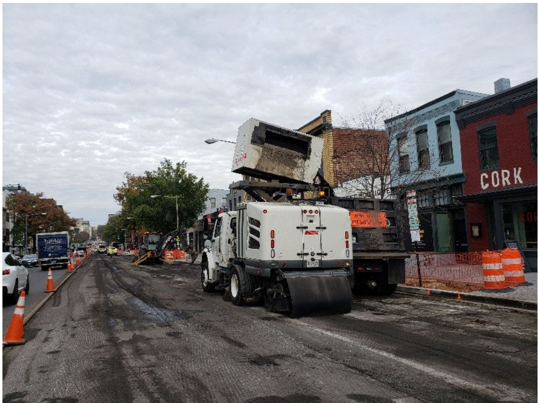
FMCC Broom Truck swept the dust and debris continuously to eliminate dust and debris along 14 th St. NW during the Milling Operation on Thursday, 11-7-2019.
