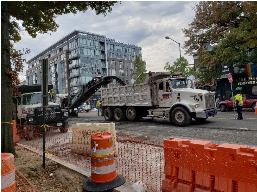
FMCC Asphalt crew Milling Operation In-Progress on Thursday, 11-7-2019 from R St. thru S St. to T St. and Wallach Place at 14 th St. NW Corridor.
