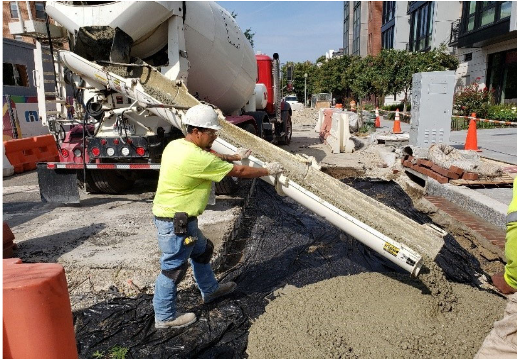
DEN Placed DC-DoT Class E with Roadway Dowels, WWF (6X6) Wire Mesh at 14 th & W St. SWC.
