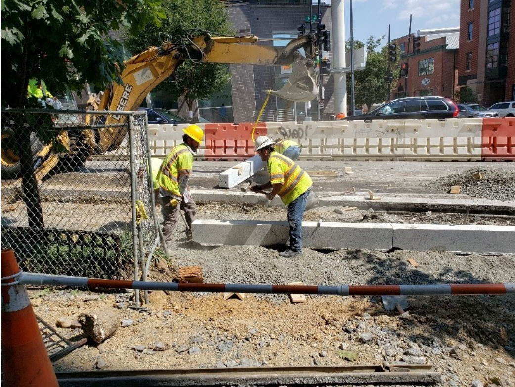
D.E.N crew placed Dry Mix, the installed a total of 74 LF of Straight Granite Stone at 14 th St. NW.
