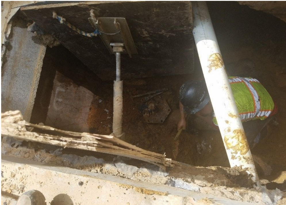
Omni removing 8" plug and installing standpipe.
