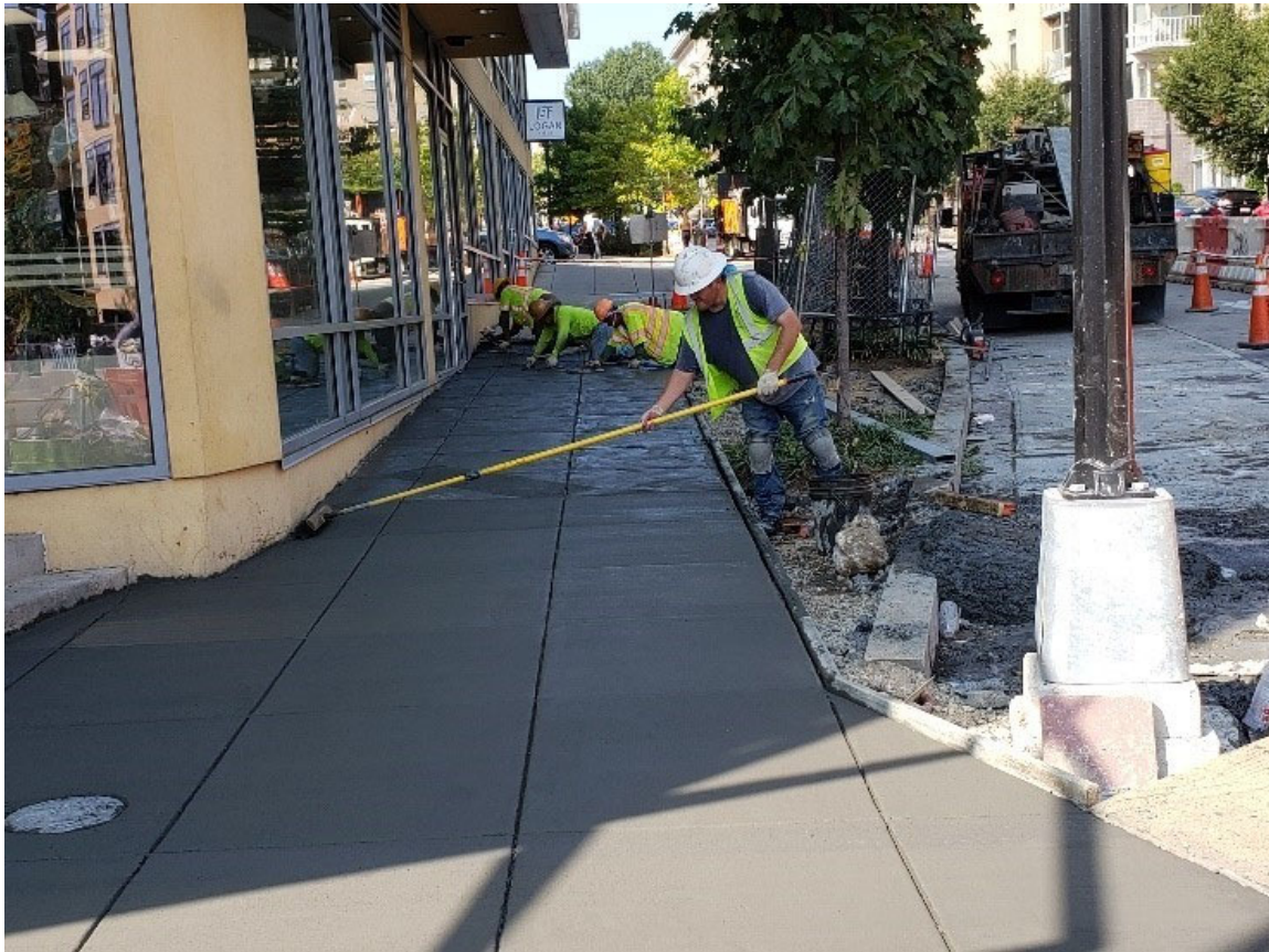
DEN placed PCC Sidewalk at 2300 Block in Front of 7-Eleven Store at 14 th St. NW.
