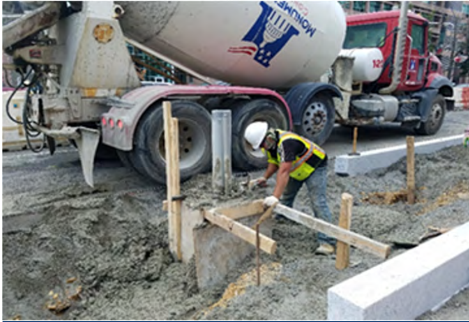
PCC concrete placed at TS-40 including encased PVC to HB-13
