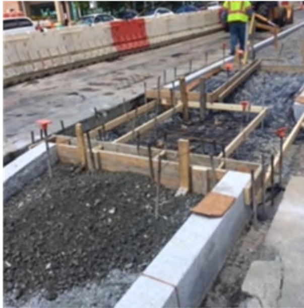
Bus Stop Island, New Bicycle Ramp
