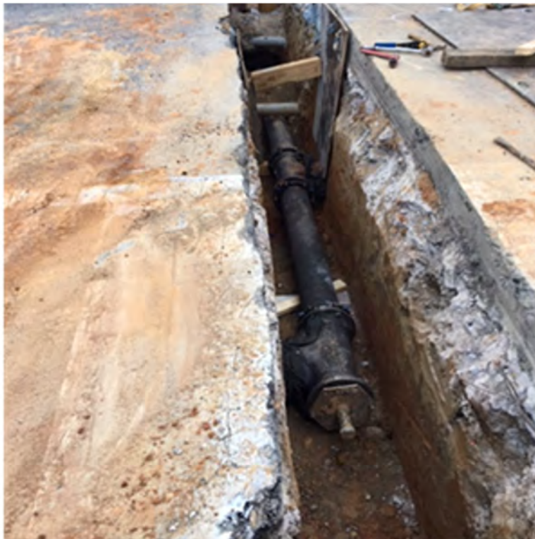
Laying pipeline 8 Inches
