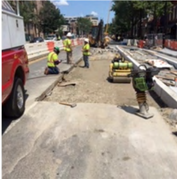
Bus Stop pad sub-grade
