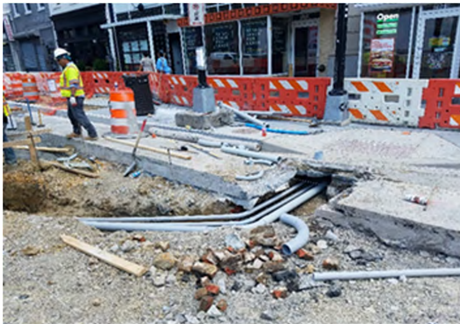
PVC conduit connected from M80 to TS40 & HB-13
