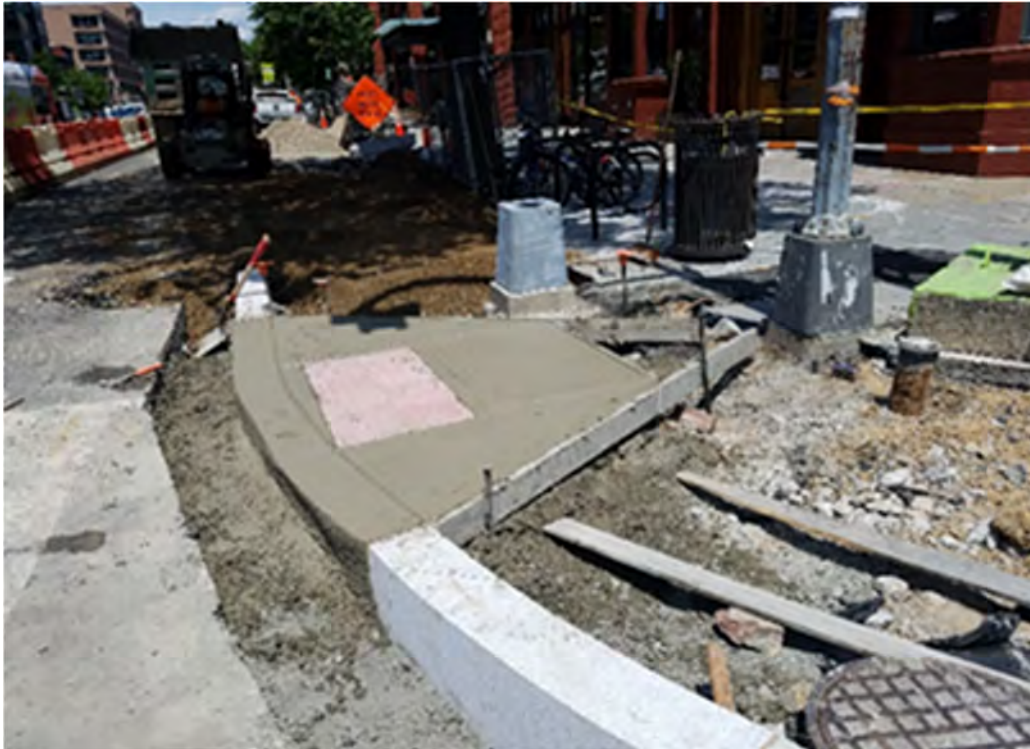
Wheelchair ramp #2 at NEC of 14 th St placed
