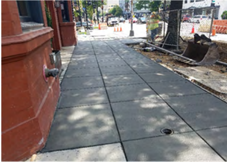
PCC sidewalk completed by D.E.N. at 1901 14 th St
