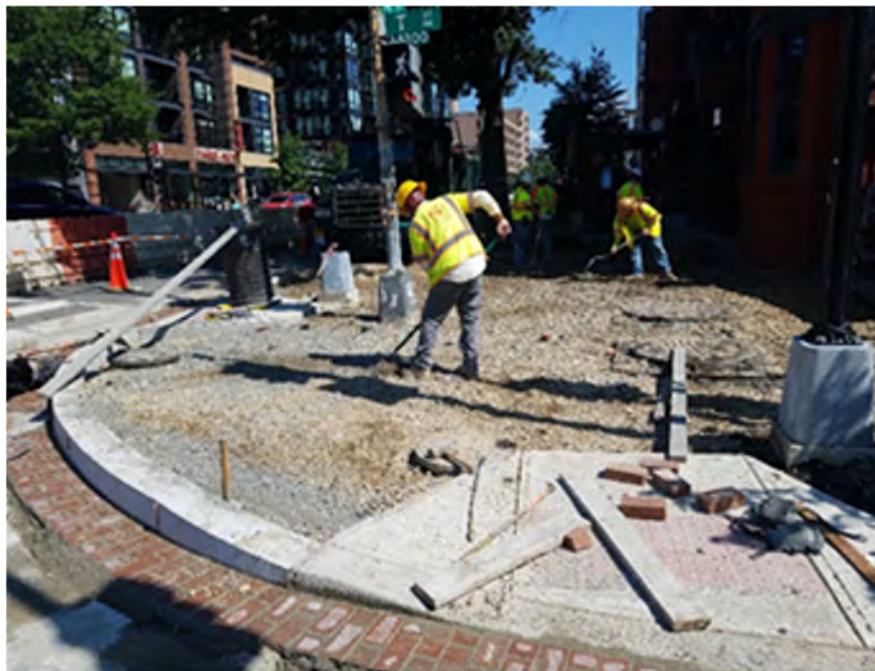
Preparation of NWC of 14 th & T St PCC sidewalk subgrade
