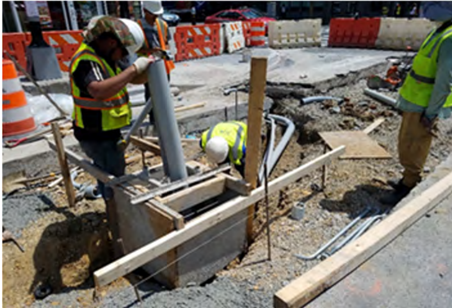
Formwork preparation of traffic signal foundation TS-40 by Omni Excavators
