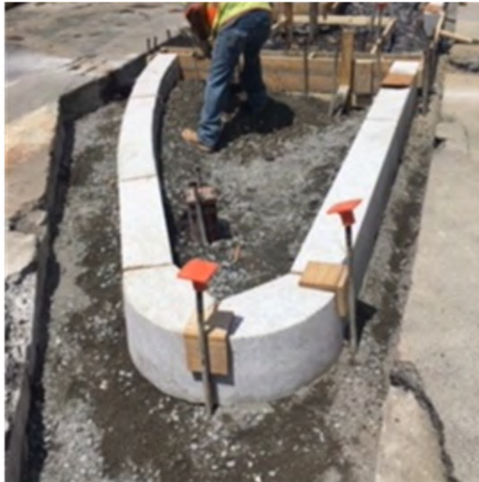
Bus Stop Island, New Bicycle Ramp
