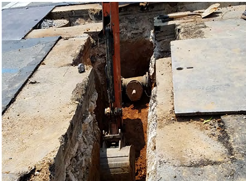
Trench excavation headed north on 14th & R St southbound lane.
