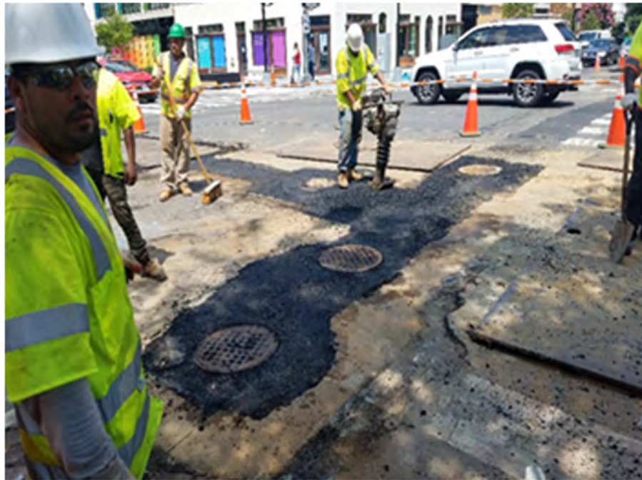
Temporary asphalt placed atop 8" water main connection.
