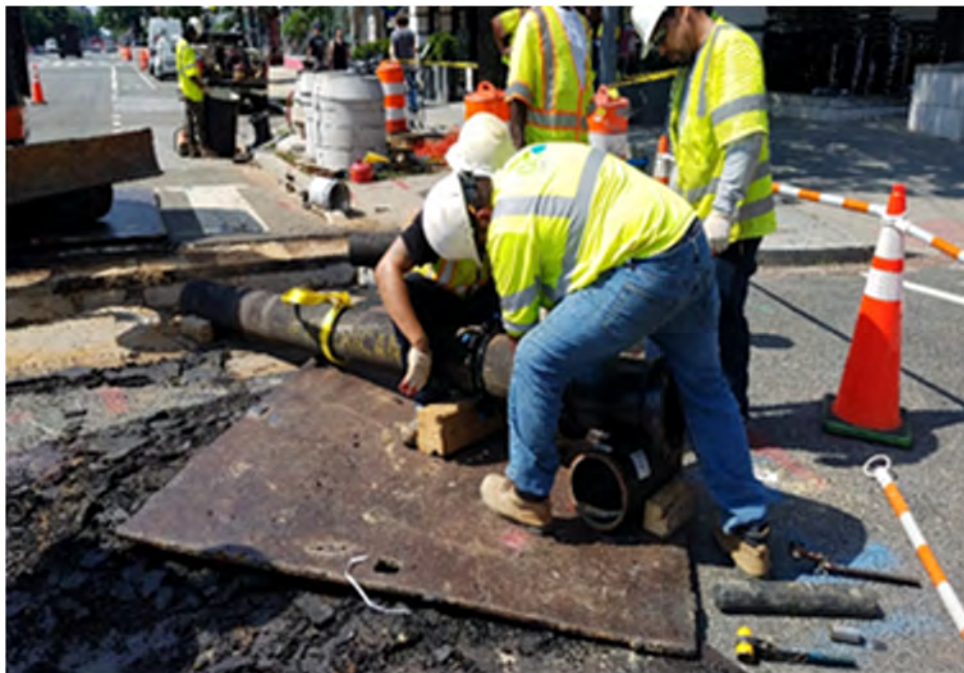
Omni Excavators working on 8" gate valve connection
