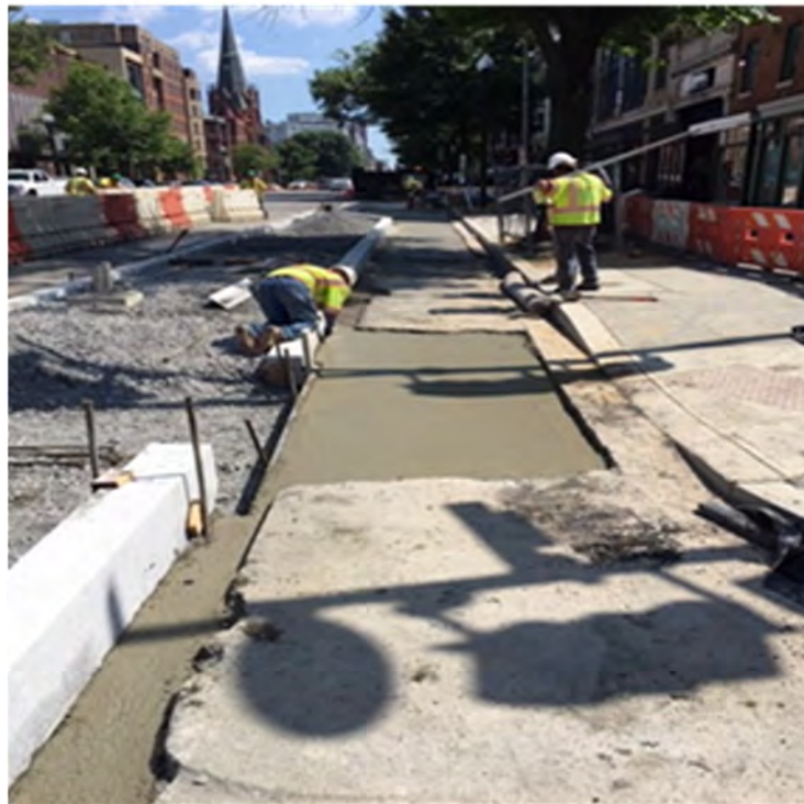
PCC 10 Inches Finishing
