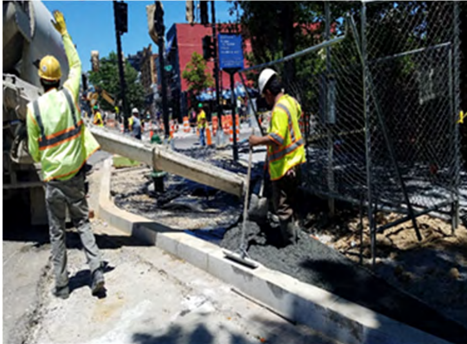
PCC sidewalk placement underway.
