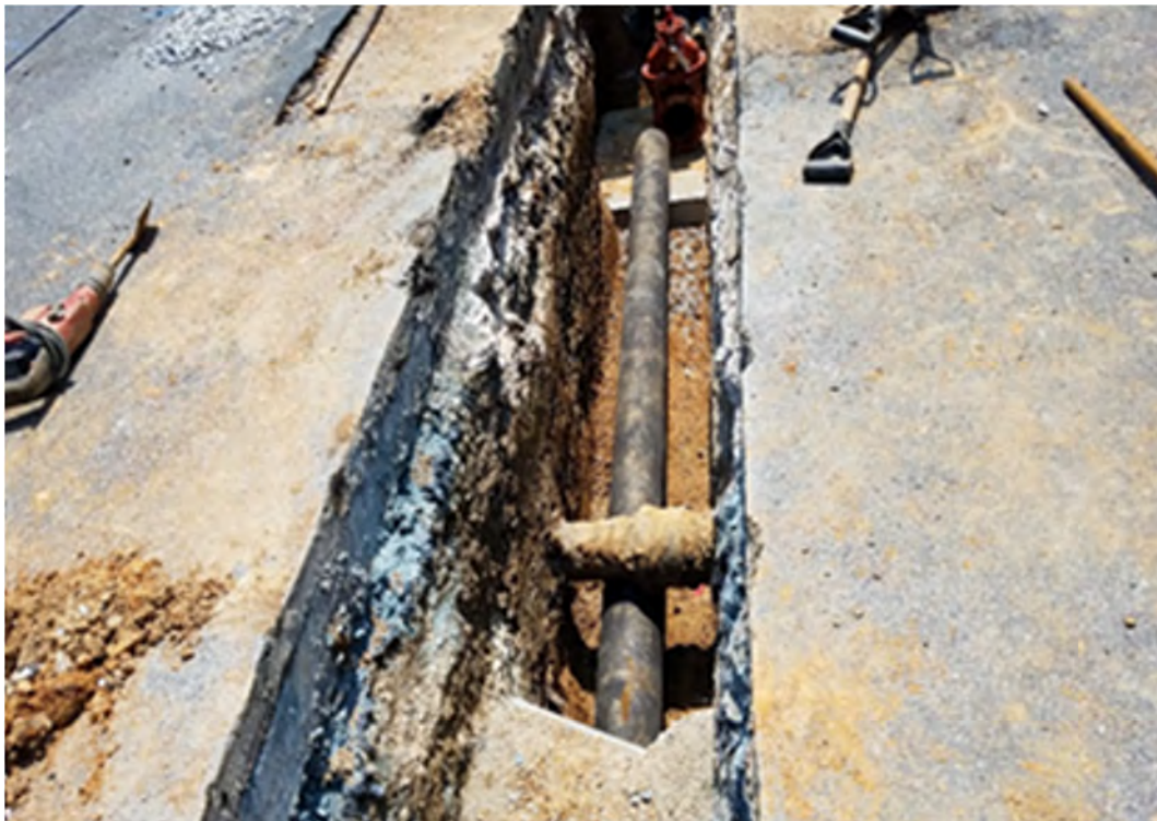
8" ductile iron pipe placed at water main trench at R St.
