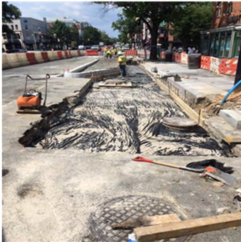
Preparation for PCC
