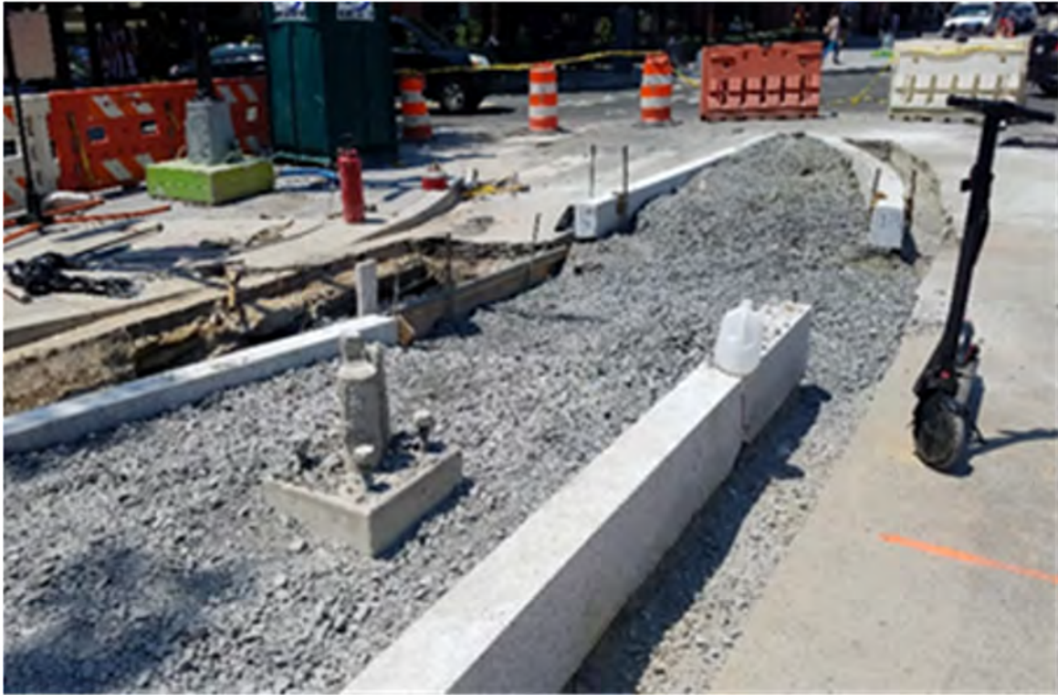
View of TS-08 foundation at SWC of 14th & RIA..
