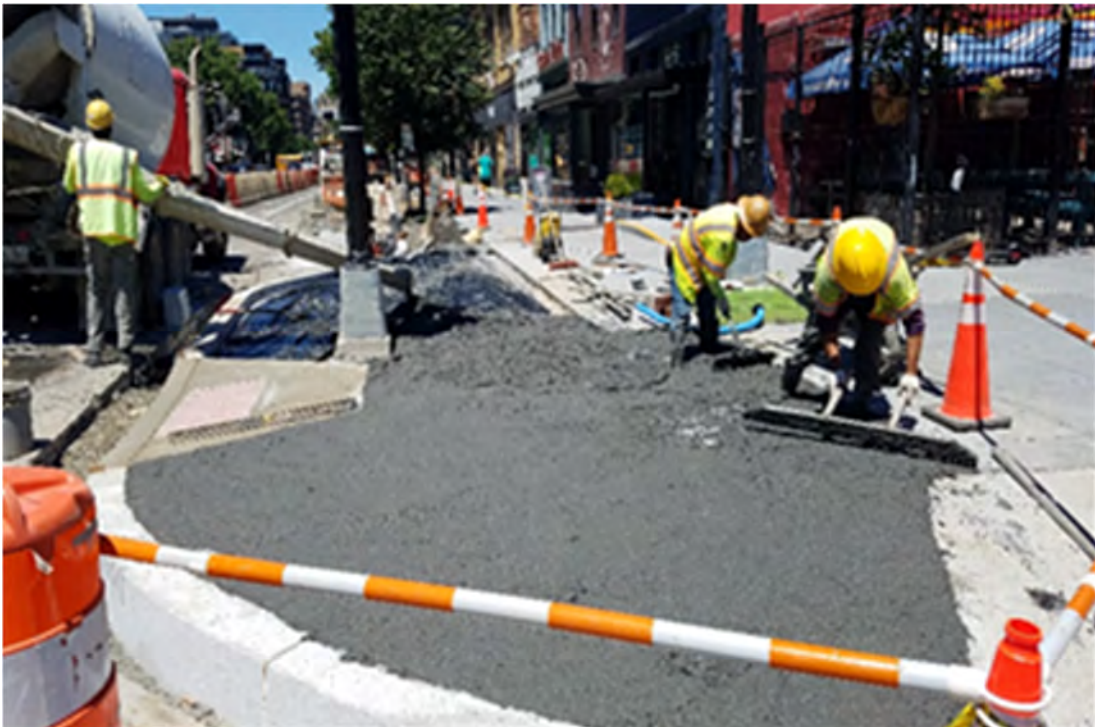
PCC sidewalk placement underway.
