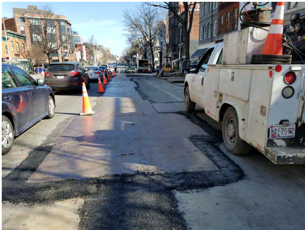
Steel Plates welded and wedged on 14 th Street
