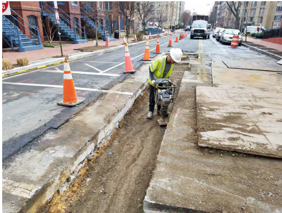
Contractor compacting Backfill Material on N Street
