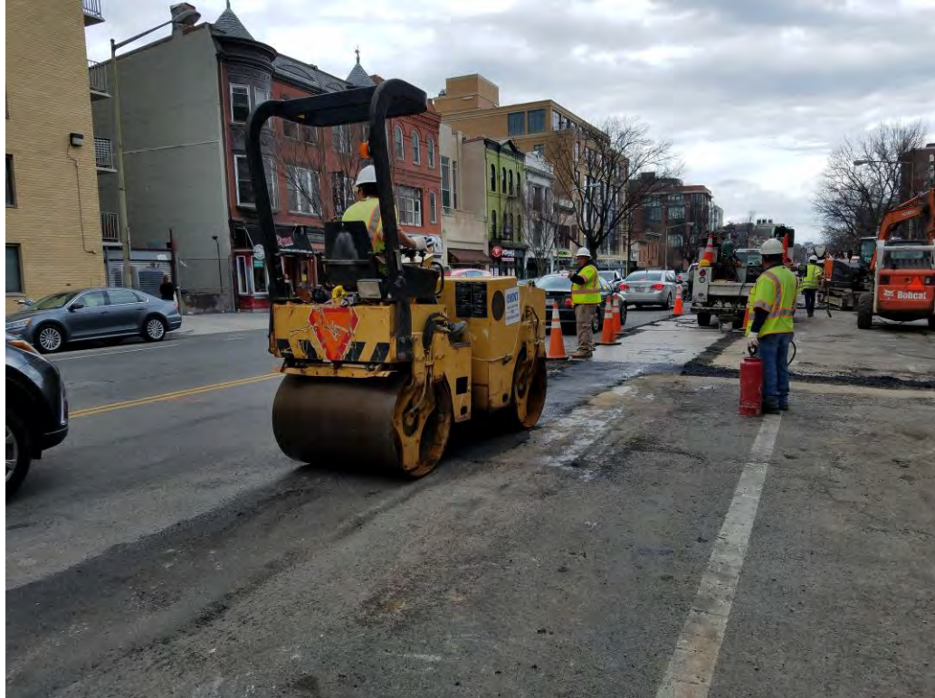
Compacting Temporary Asphalt between N Street and Rhode Island Ave
