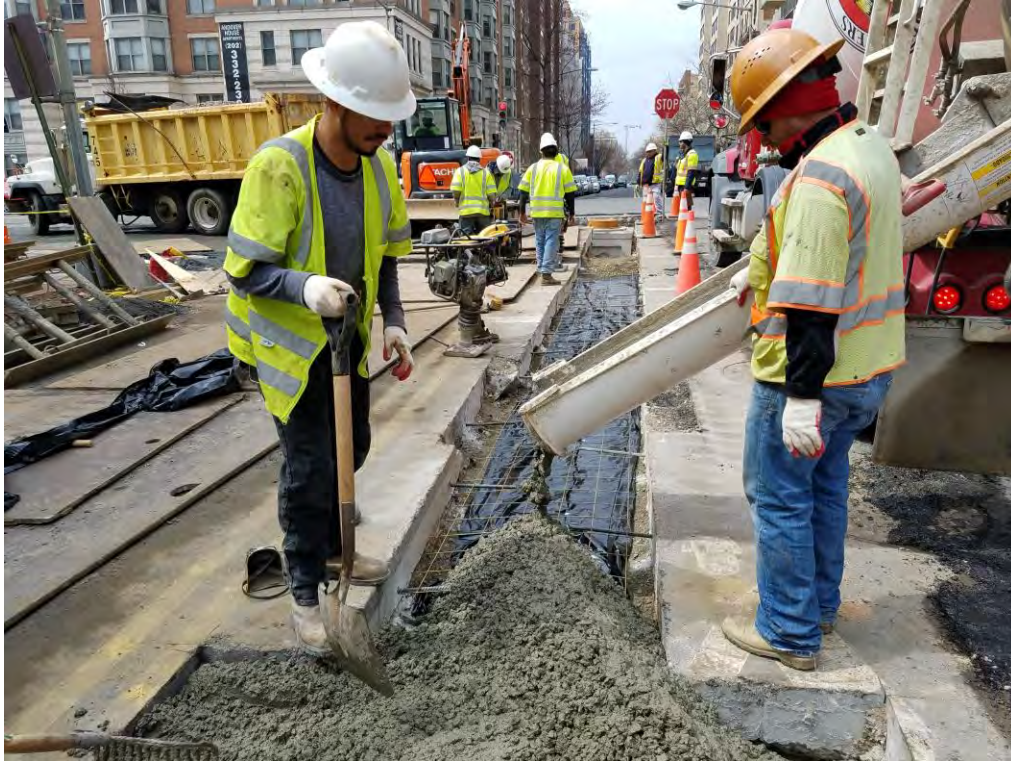
Placing PCC Base on N Street
