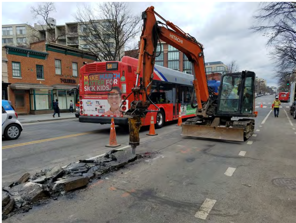
Demo of existing asphalt between N Street and Rhode Island Ave
