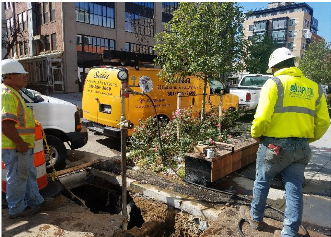
Pressure testing at 1357 R St standpipe by Omni.
