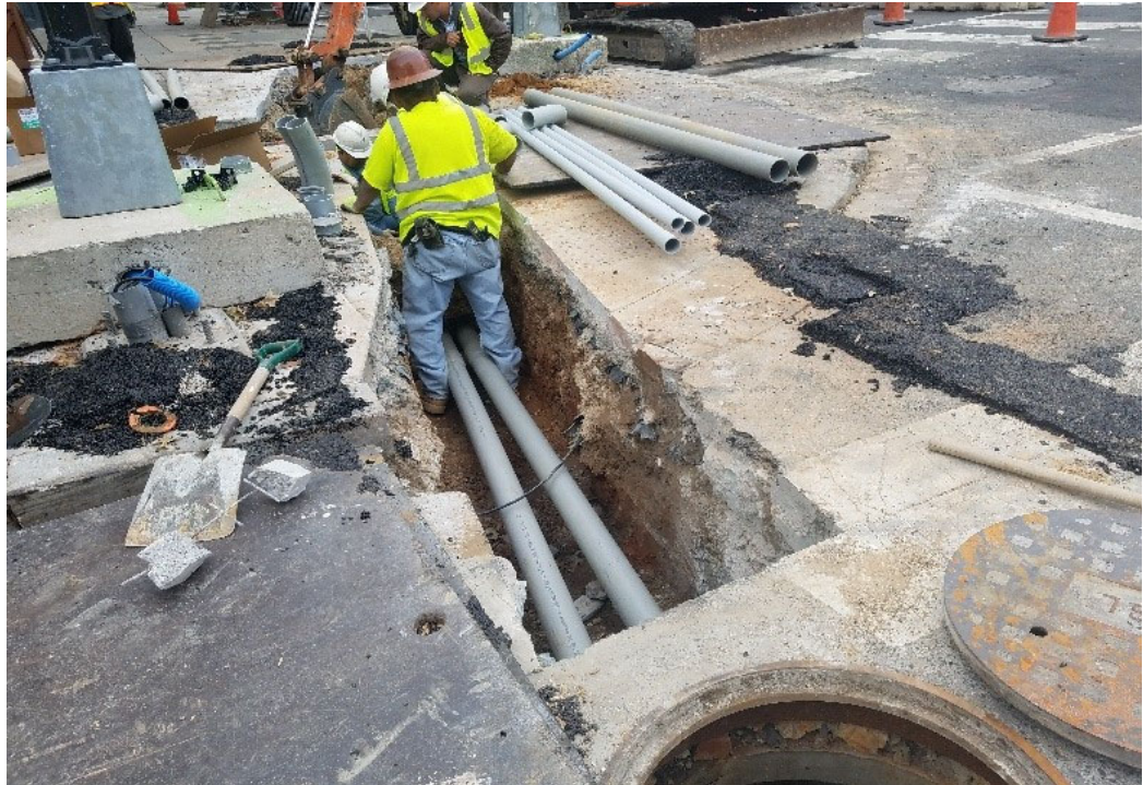
PVC conduit placed from M46 to EM05.
