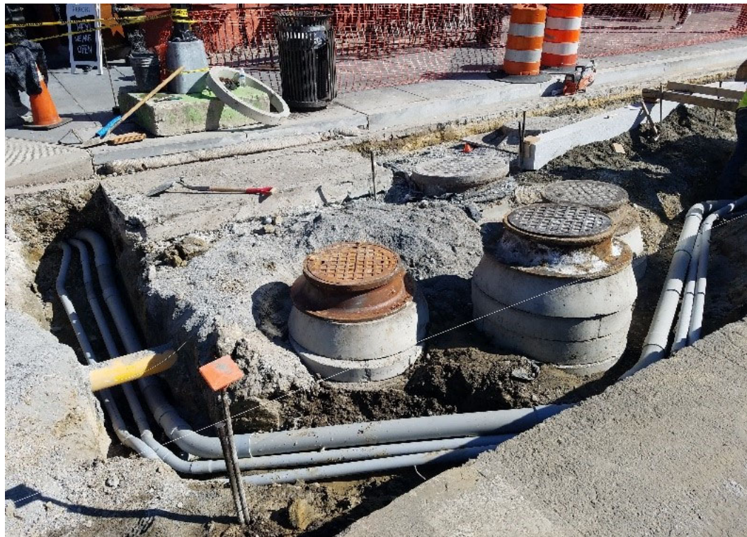
Ramhoe used to demolish for PVC conduit tie-in by Omni
