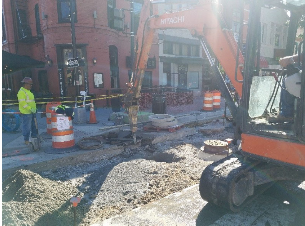
Ramhoe used to demolish for PVC conduit tie-in by Omni
