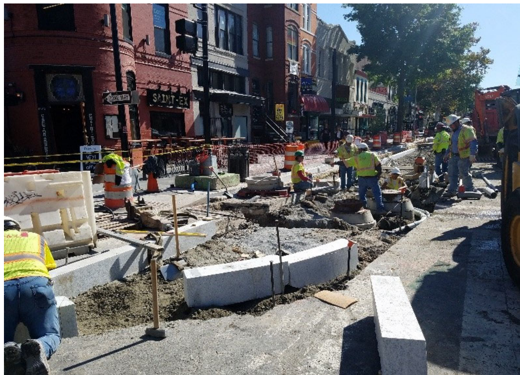
Omni and FMCC working at bus island location
