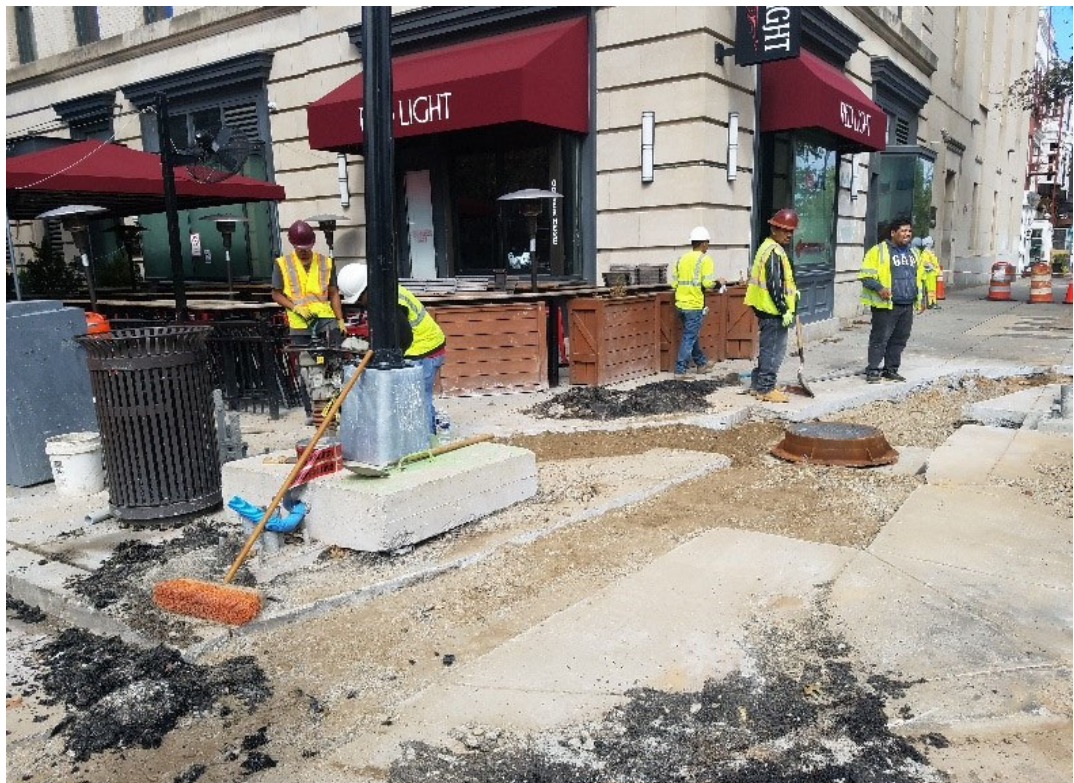
Backfill of NWC of 14th & R St near signal manhole M46
