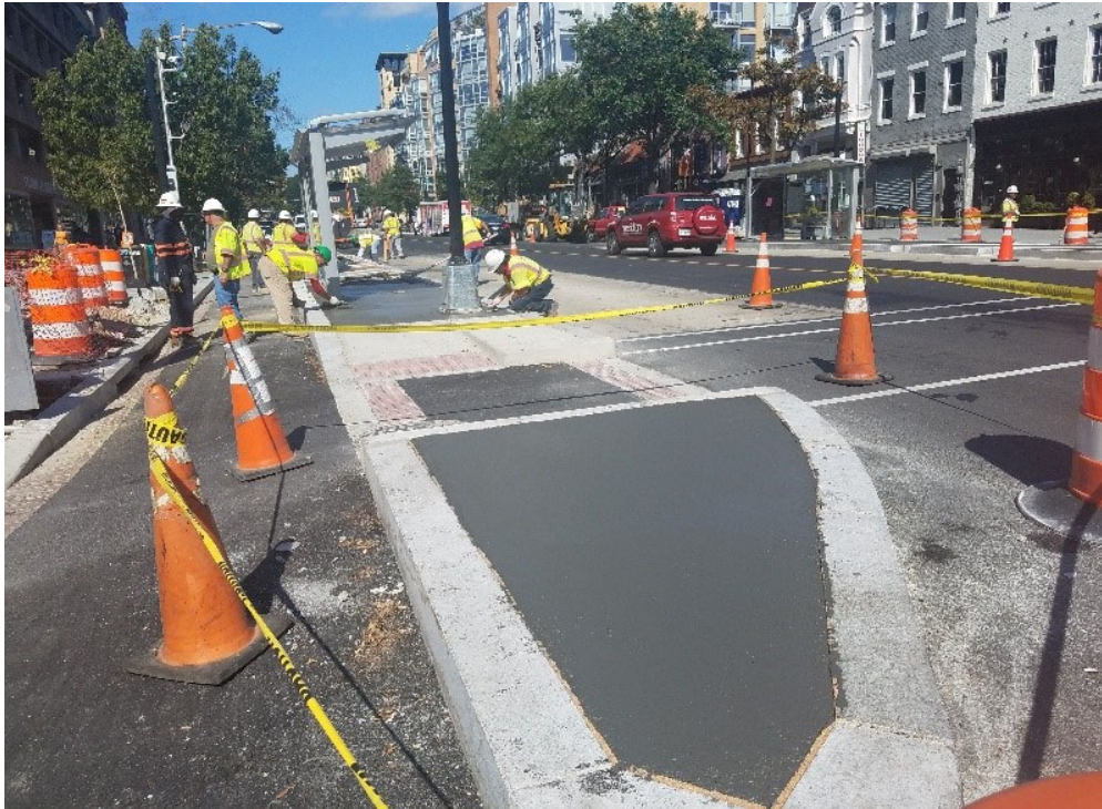
Class F concrete completed at NWC of 14th & U St.
