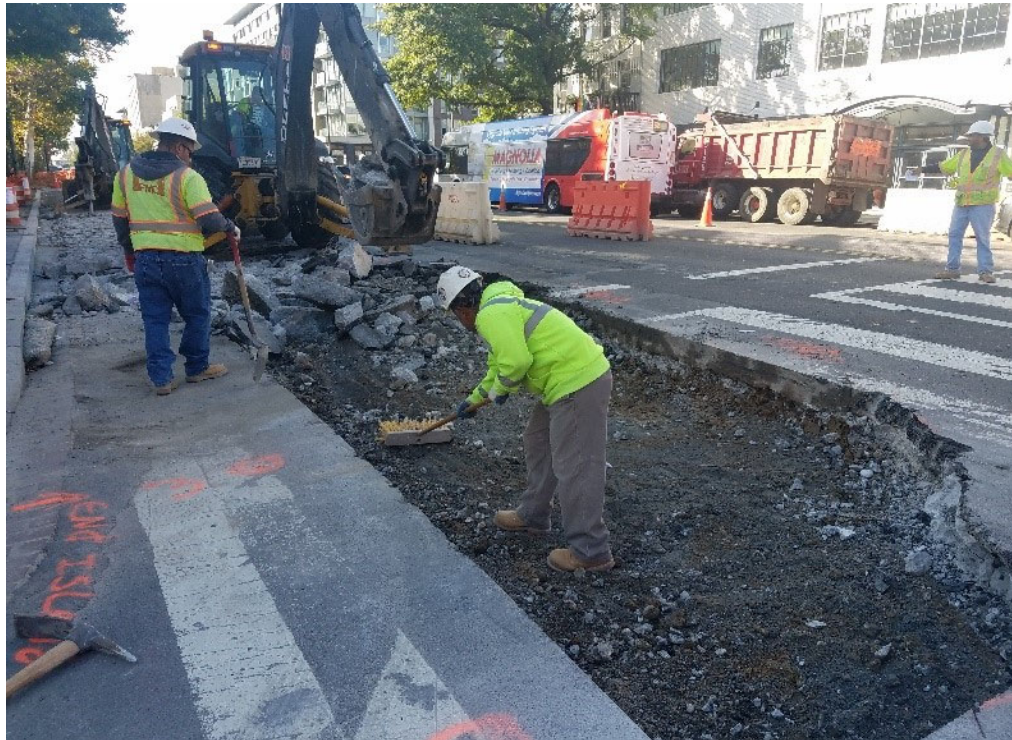
Excavation of SEC of 14th & T St bus island
