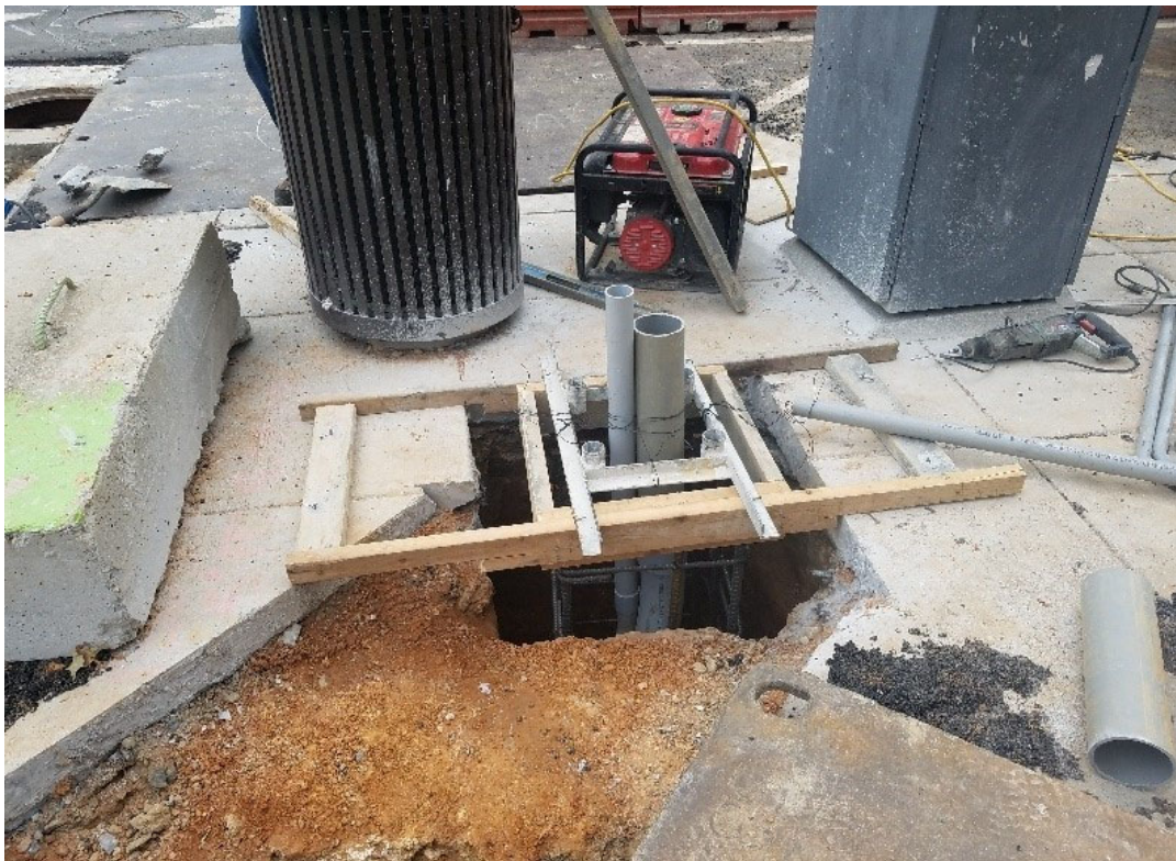
Signal pole foundation L58 at NWC of 14th & R St.
