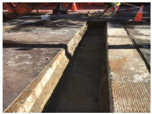
PVC Conduit electrical trench to Street Light L113
