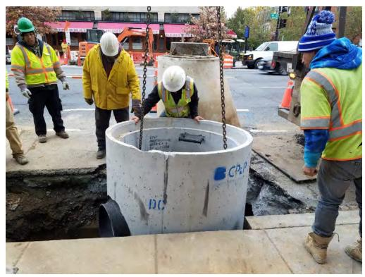
Installation of Combined Sewer manhole at the near 14th and Q Street
