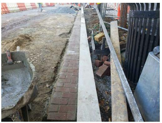
Installation of Brick Gutter between N Street and Rhode Island Ave westside
