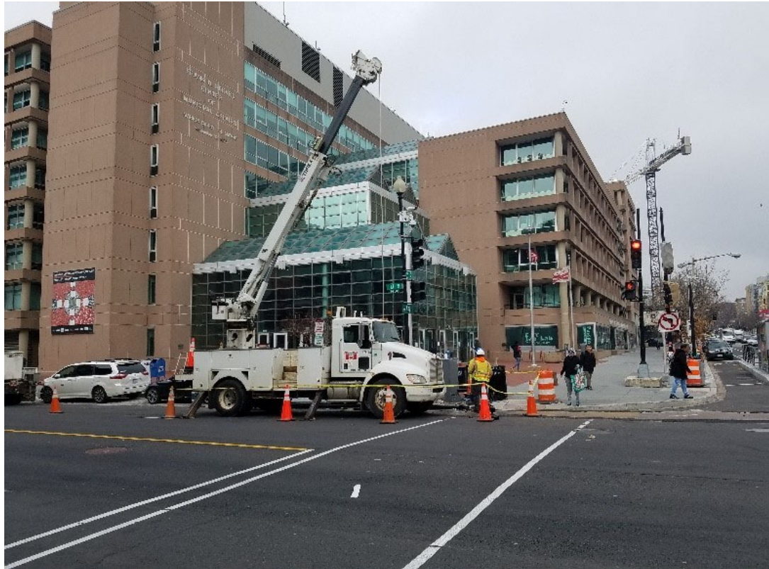
FMCC electrical crew at NWC of 14 th & U St installing signal poles
