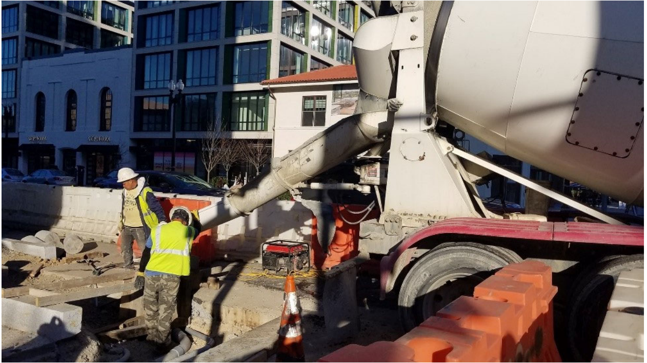
Foundation pouring at TS-27
