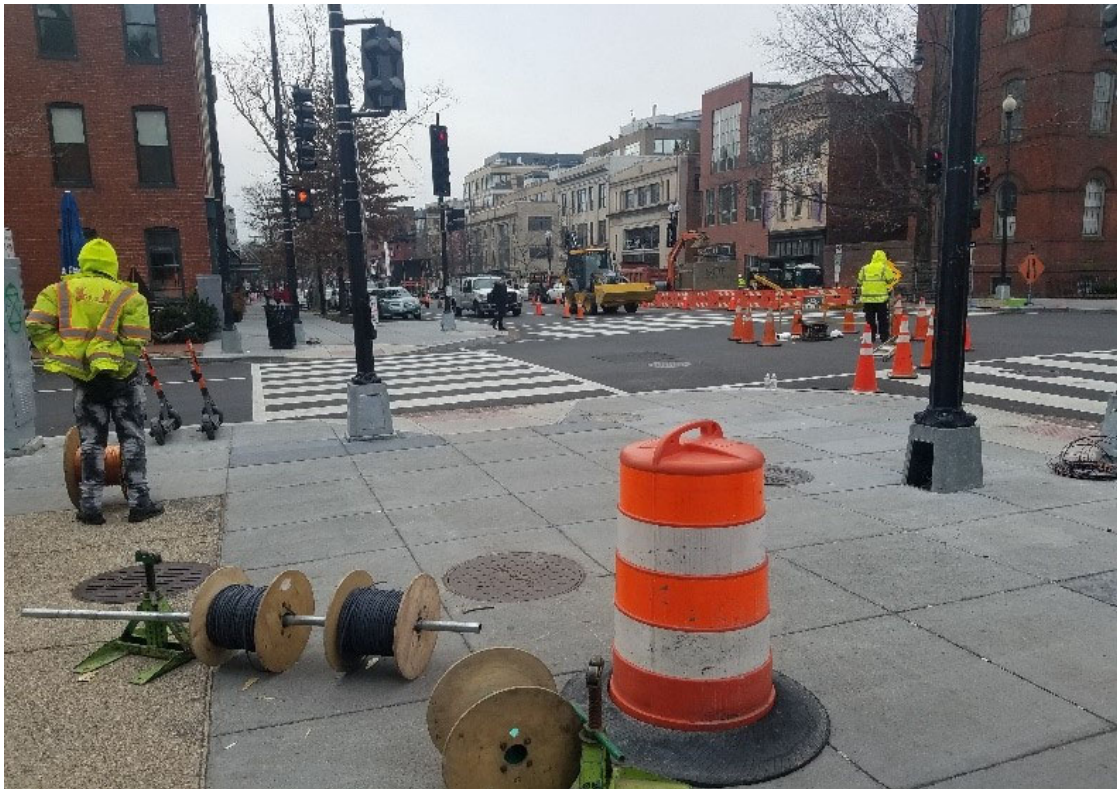
FMCC electrical crew splicing cable at 14 th & Q St
