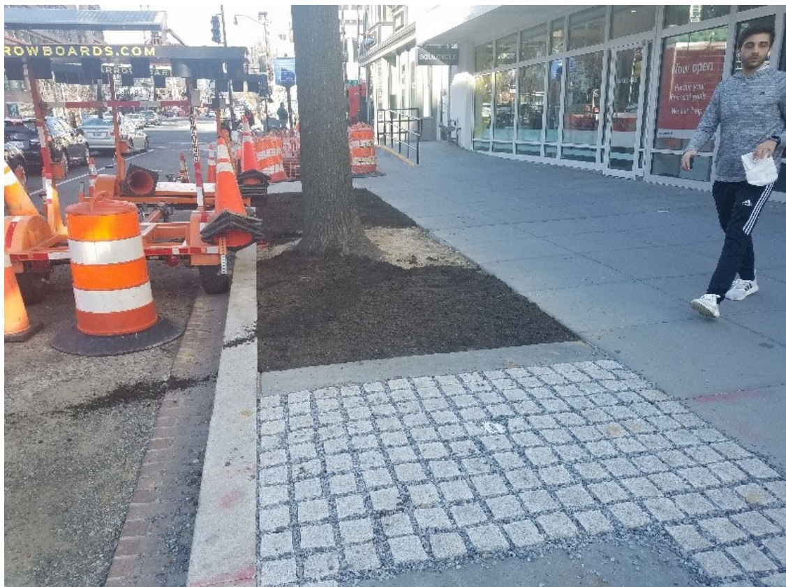
Continued placement of topsoil by landscaping crew
