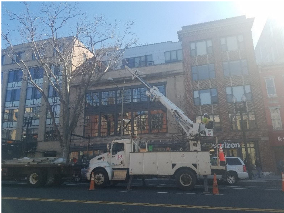
Existing pole R31 being removed by FMCC electrical crew
