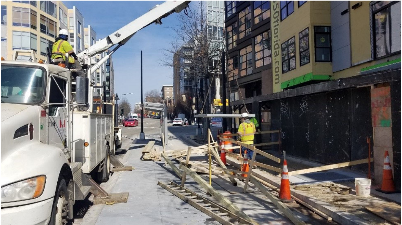
Vault delivered and setup in front of Ellisdale
