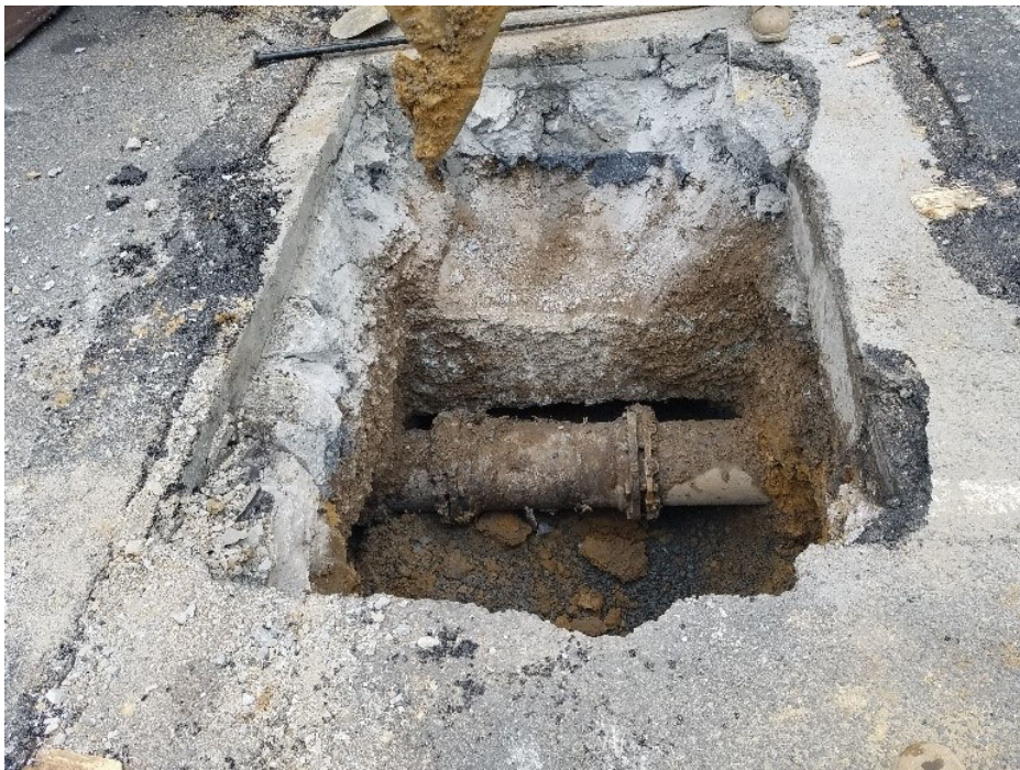
Existing water main exposed in preparation for connection to new 12" main
