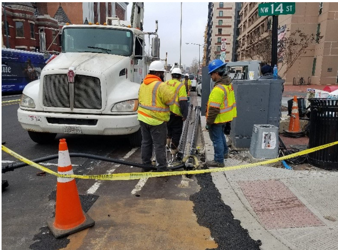
FMCC electrical crew at NWC of 14 th & U St installing signal poles
