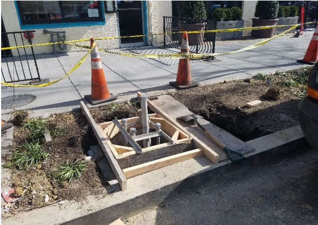
Foundation L82/T20 formed and ready for concrete placement
