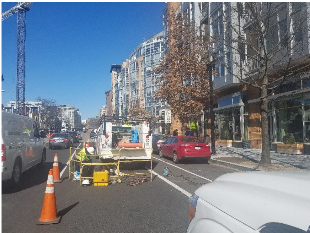
FMCC electrical crew splicing cable at 2000 block south of V St
