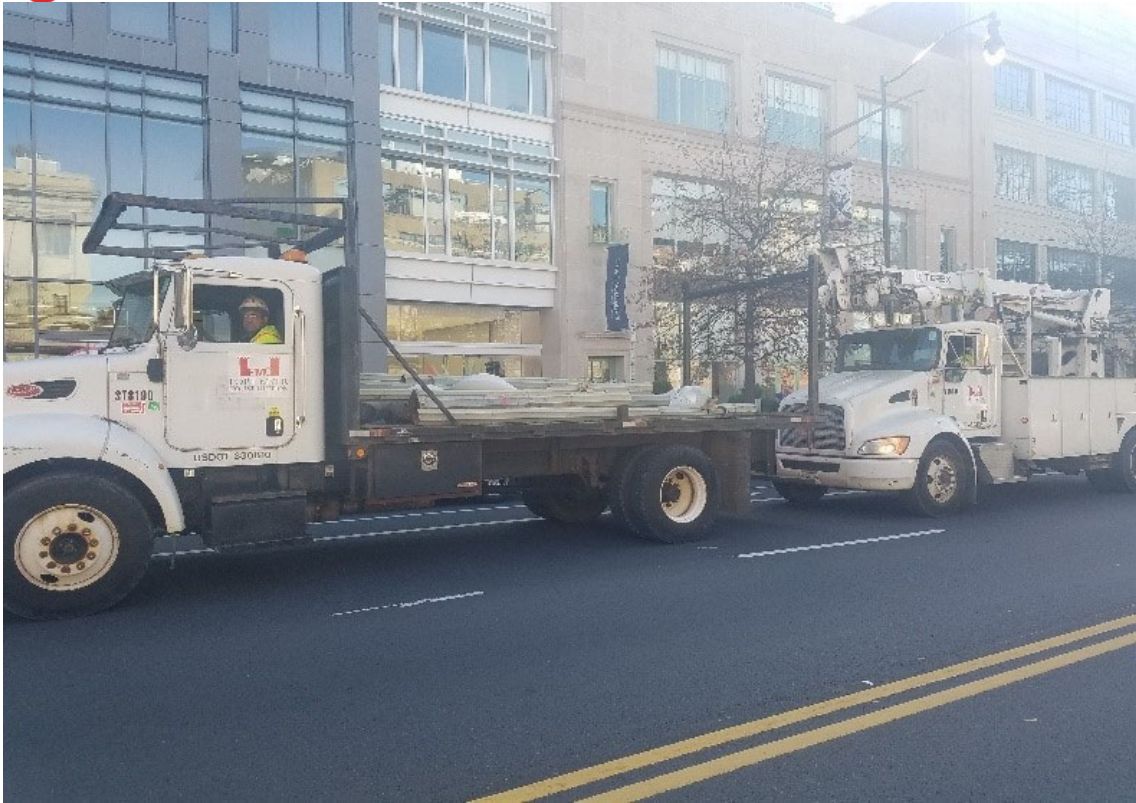
Poles loaded on truck via crane truck
