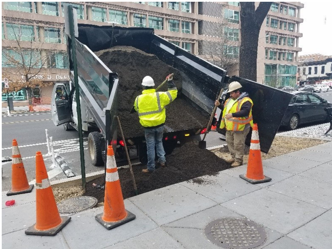
Landscapers placing topsoil at 2000 block of 14 th St
