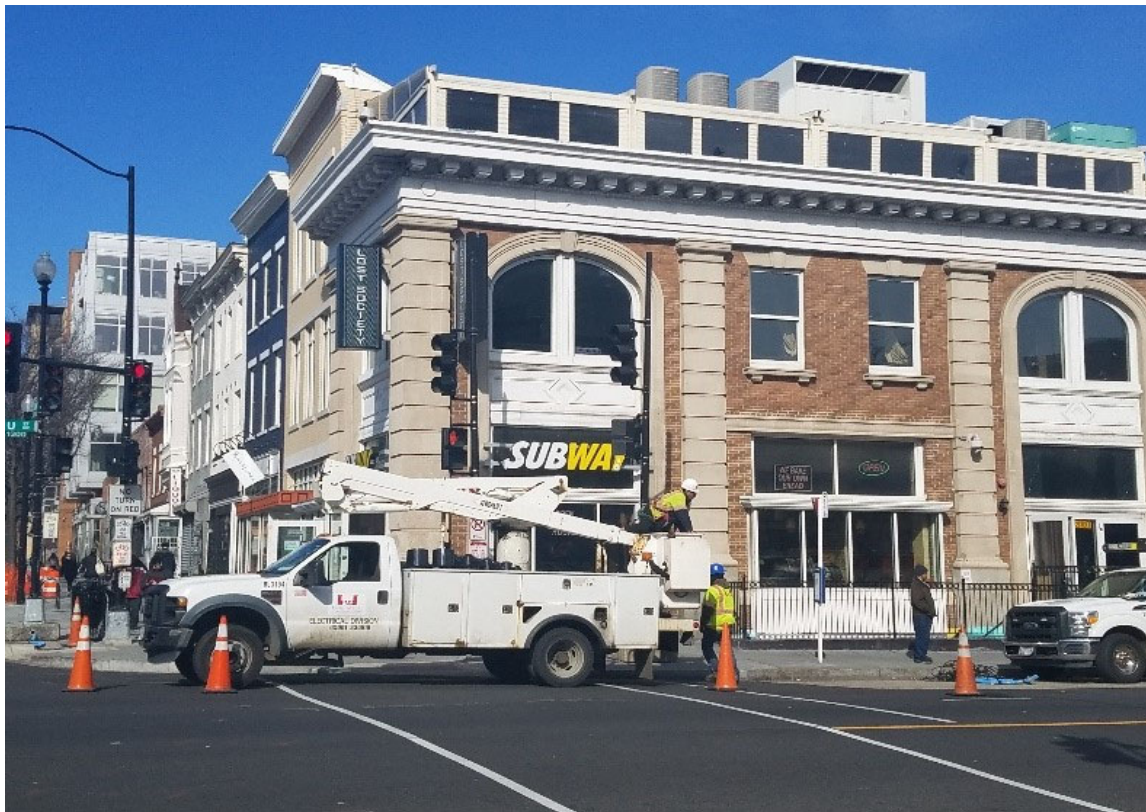
FMCC Electrical crew at NEC of 14 th & U St
