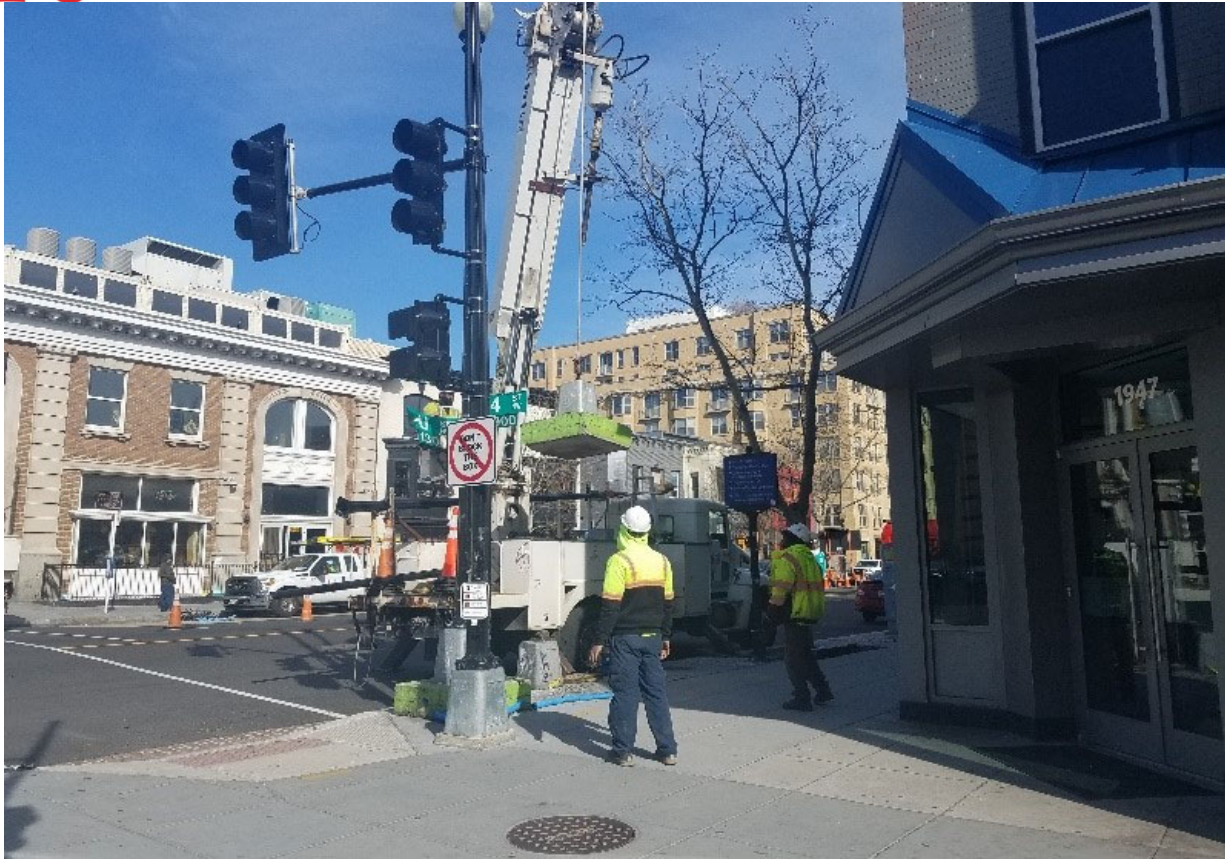
Removal of temporary traffic pole and base
