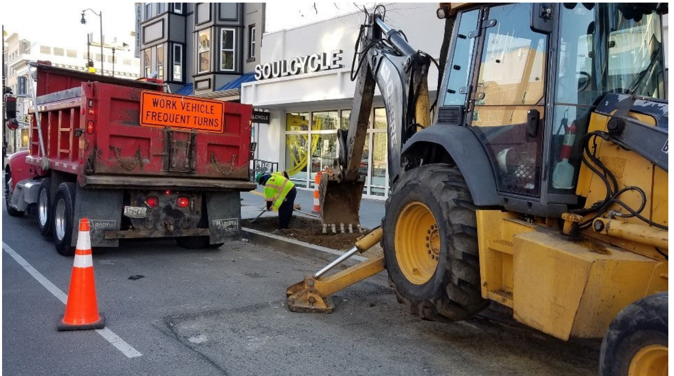
FMCC setup for landscaping work at multiple locations
