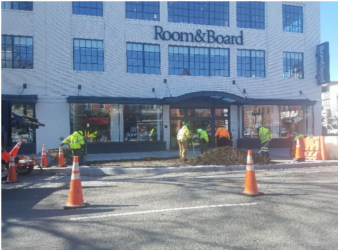
FMCC assisting landscapers with placement of topsoil at planter area
