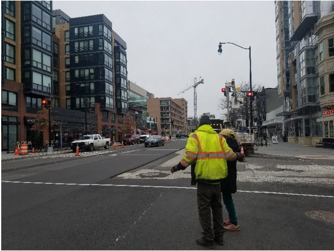
FMCC electrical crew testing push button at Wallach St
