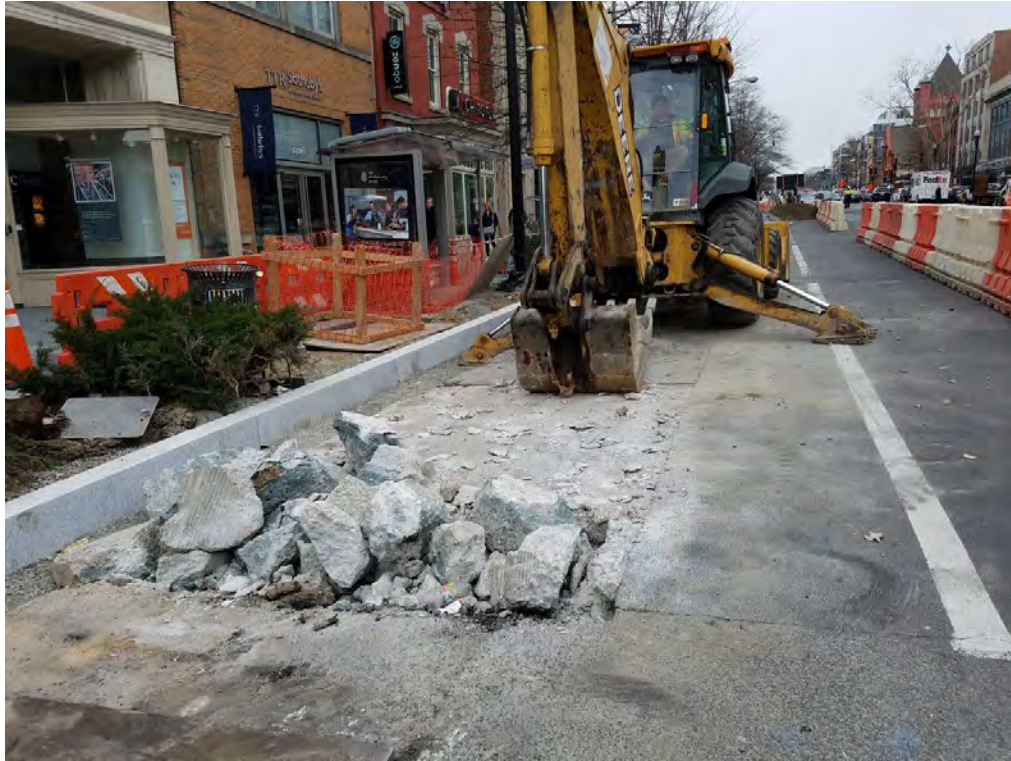
Demo of Existing Bus Pad
