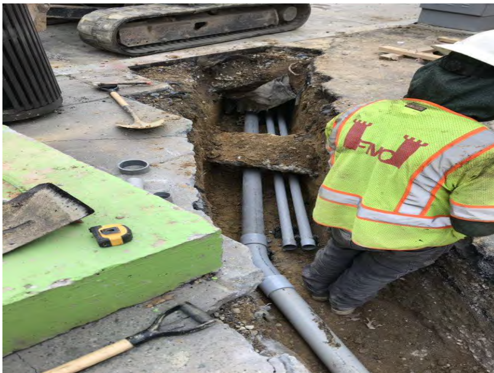
Installation 2" and 4" PVC Electrical Conduit
