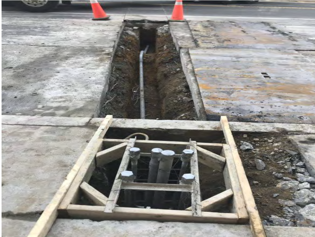
Streetlight Foundation and 2" PVC Conduit
