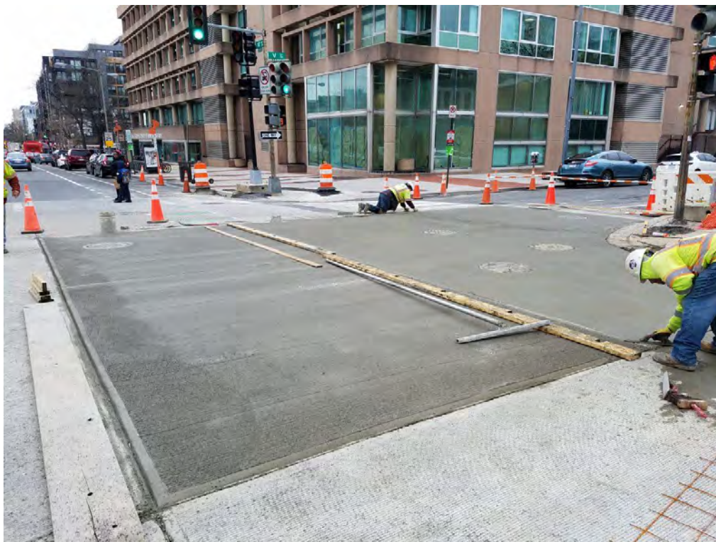
PCC Pavement Repair between V Street and W Street
