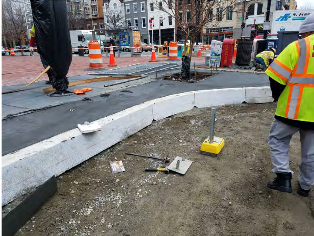
Compaction Testing of GAB Stone
