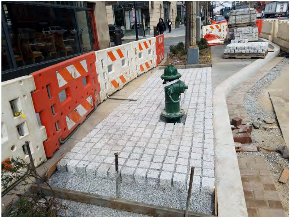
Installation Granite Cobble Stone
