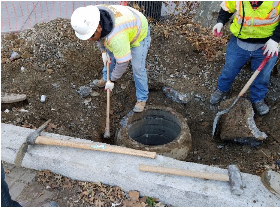
Sewer manhole adjustment near 1831 14th St by FMCC
