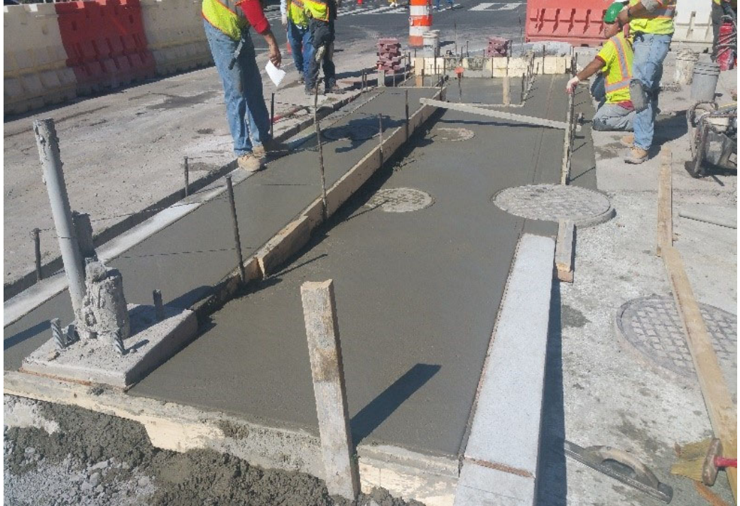
Utility manholes adjusted at SEC of 14th & T St
