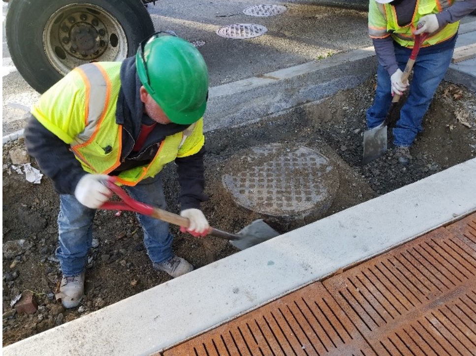
Second Pepco manhole to be adjusted by FMCC
