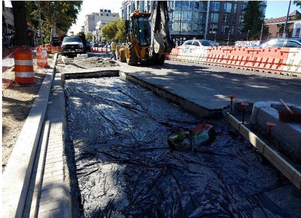
Location near SEC of 14th & T St where bus pad was removed for new directional bus island.
