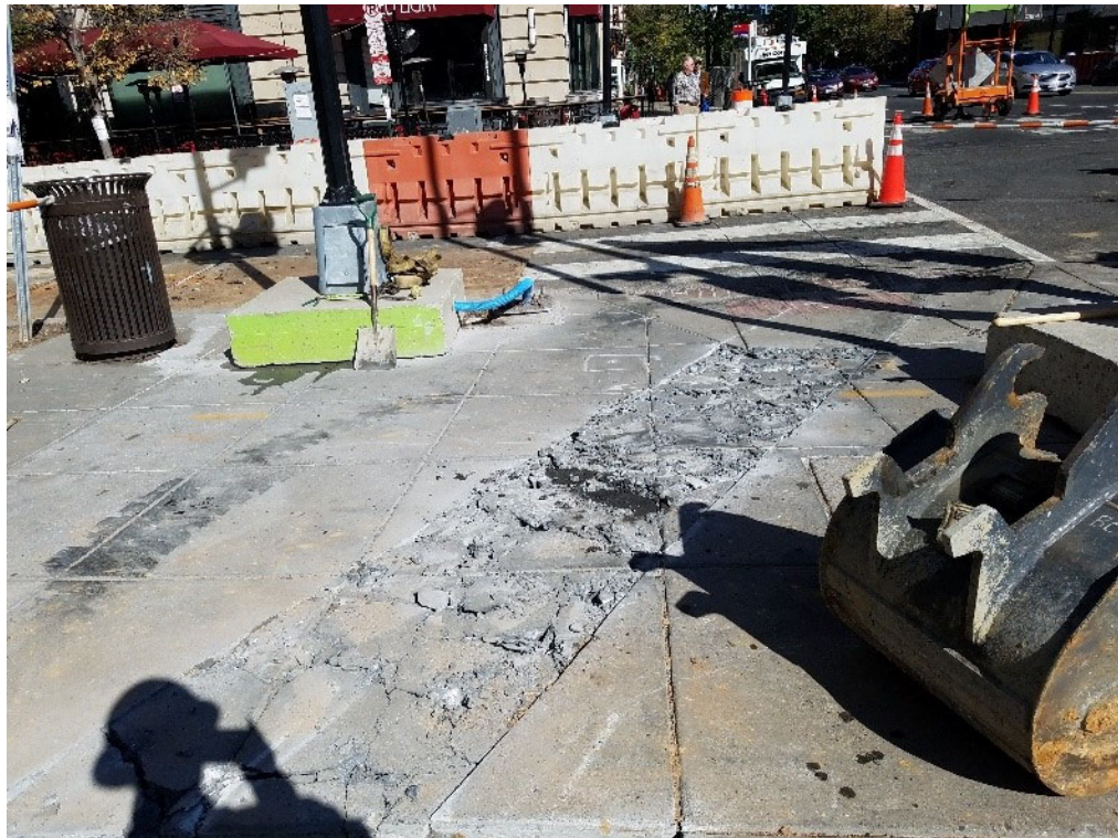
Trench to be excavated by Omni from M44 to EM05.
