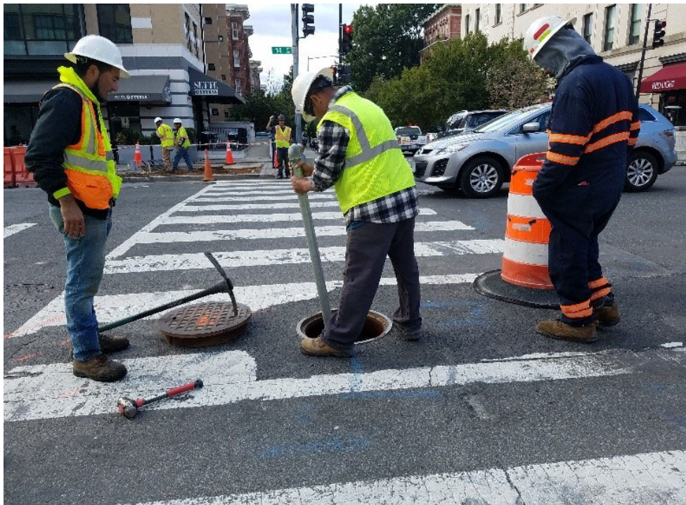
Omni Working at 14th & R St during pressure test.
