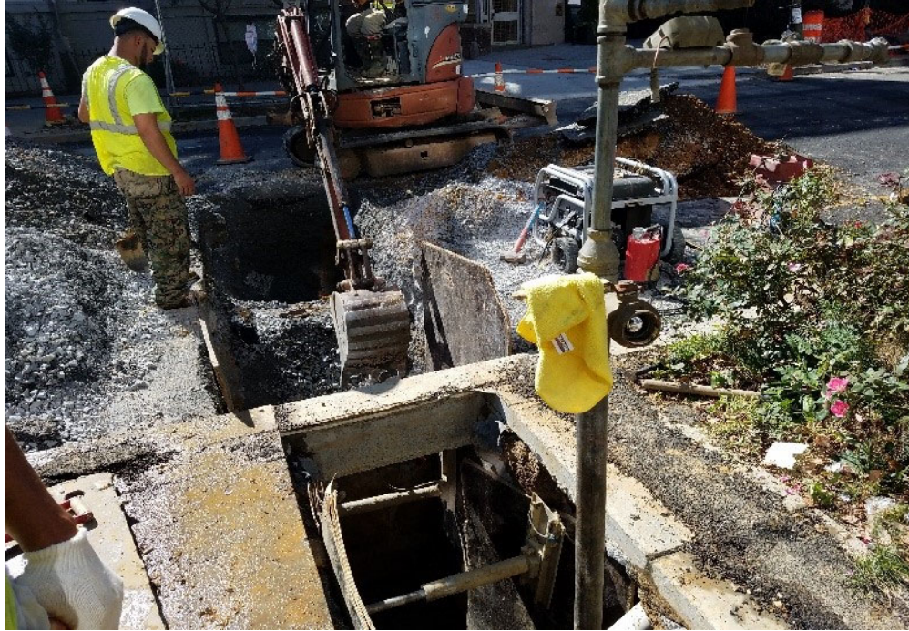
Trench opened at new 8" D.I.P. for leak found
