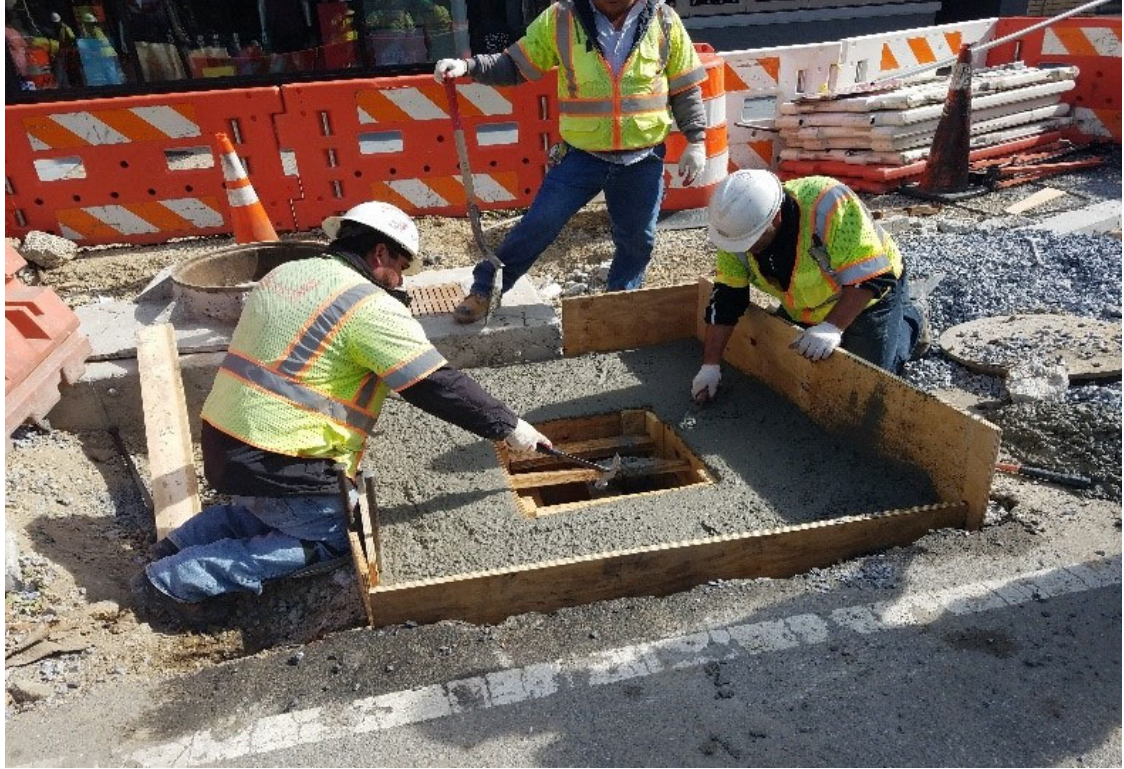
Concrete placed atop PEPCO manhole by FMCC
