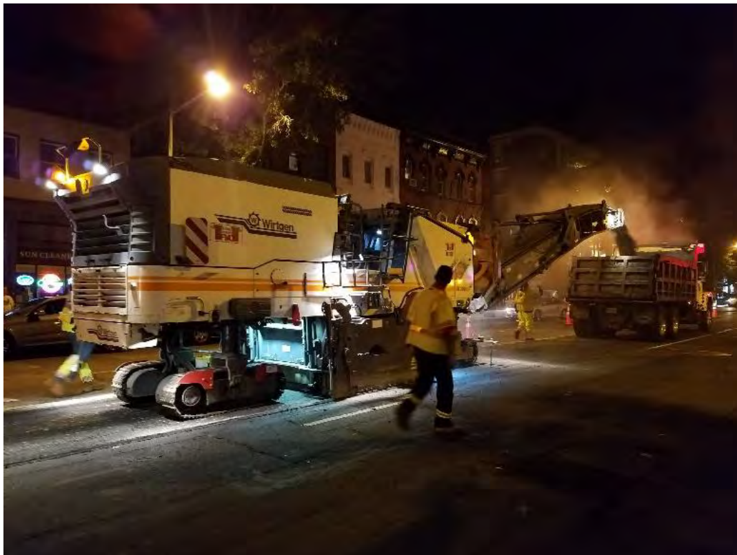
Milling of 14 th St. NB by FMCC between Rhode Island Ave & P St.
