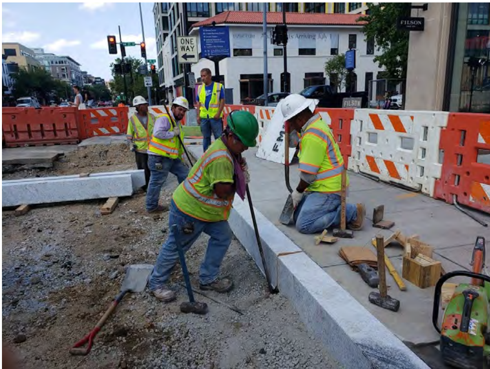
Straight Granite Curb install at 14 th St. NW & R Street
