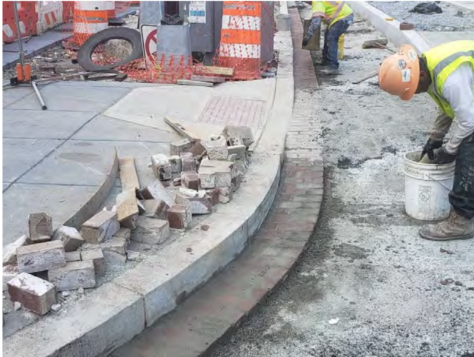
FMCC completing brick & gutter work at 14 th St. NW & U St.
