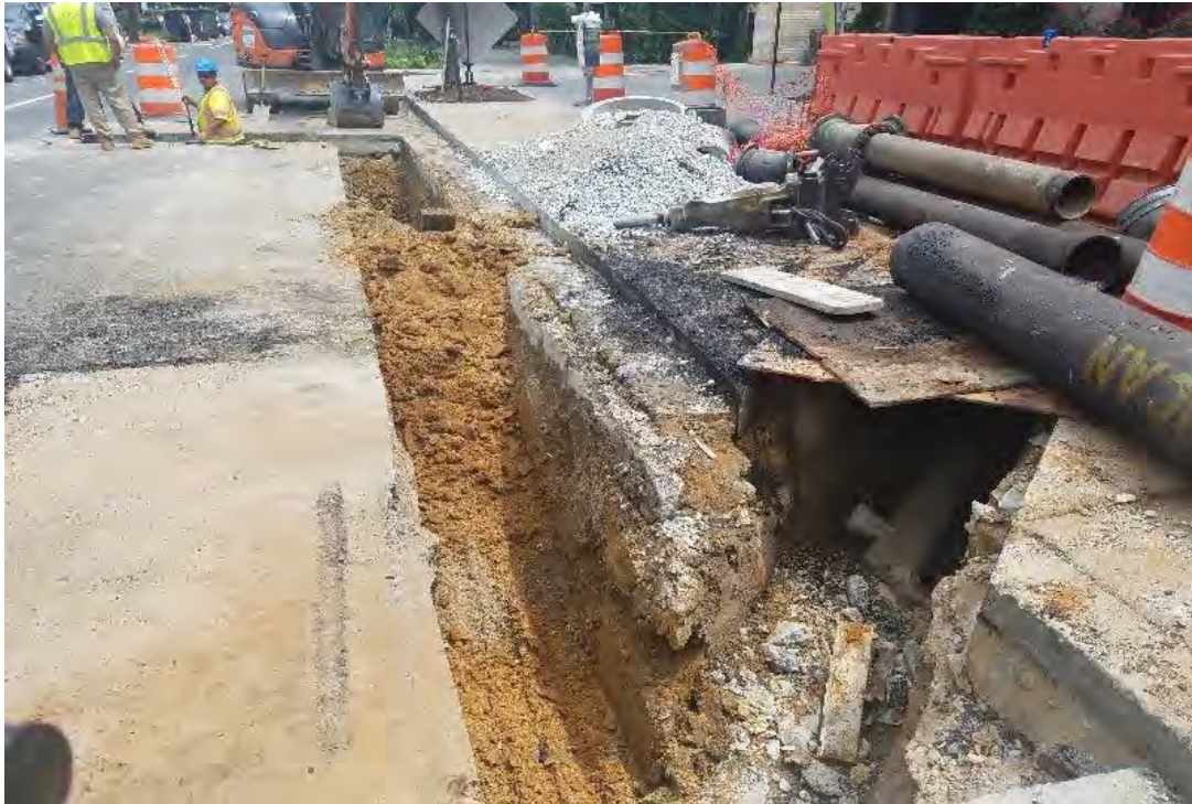
Excavation for watermain installation work at 14 th & R St.
