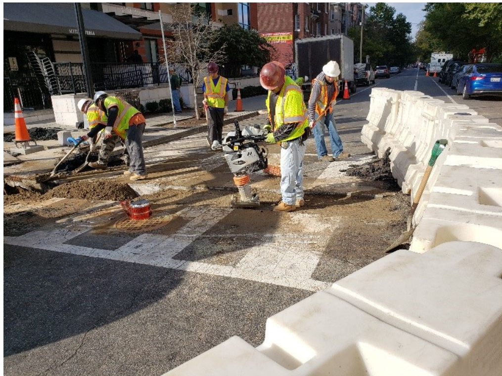
OMNI, Inc. crew backfilled a Conduit Trench (Duct-Bank) Trench at Crosswalk on R St. & 14 th St. NW Intersection between NWC and SWC of Intersection on Monday, 10-21-2019.
