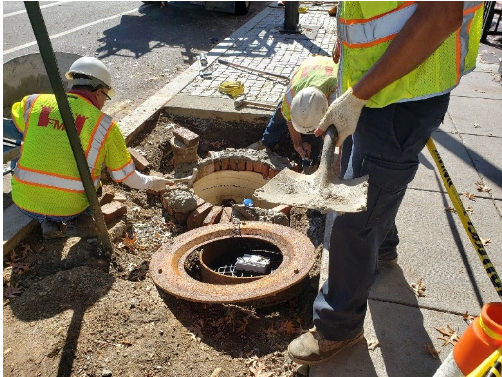
FMCC Landscaping Excavation crew adjusted 2 Utility MH on Wed. 10-23-2019
