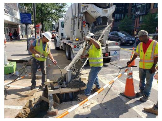
OMNI Pouring traffic pole foundation at 14th St. NW & U St.
