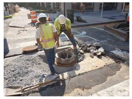
Adjusting manhole elevation to match finish grade at 14th St. & R St. NW
