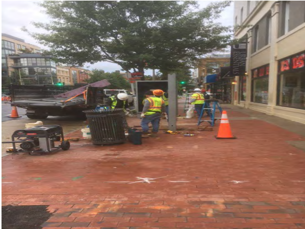
Clear Channel Subcontractor removing Bus Shelter at 14 th and Rhode Island
