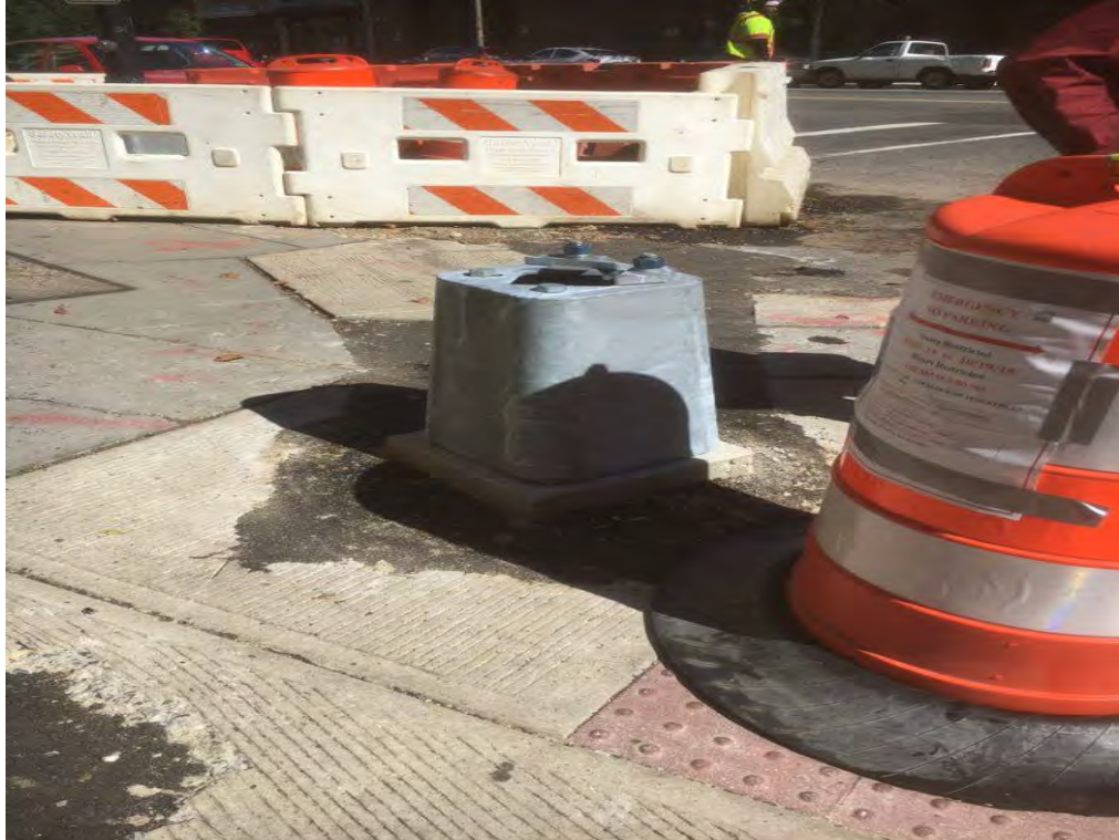
Installation of the Transformer Bases onto New Traffic Signal / Pendent Poles
