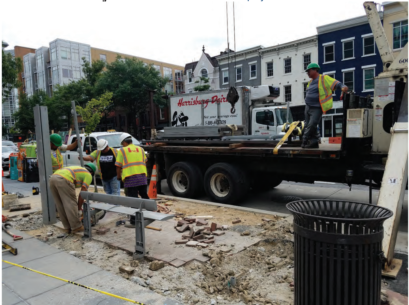
Bus Shelter removal by FMCC at NWC of 14 th & W St.
