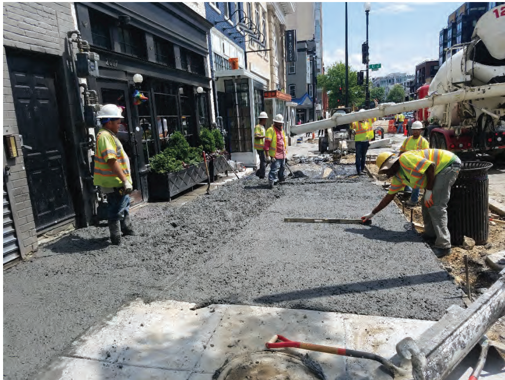
Placed and finish sidewalk between V and U St NW.
