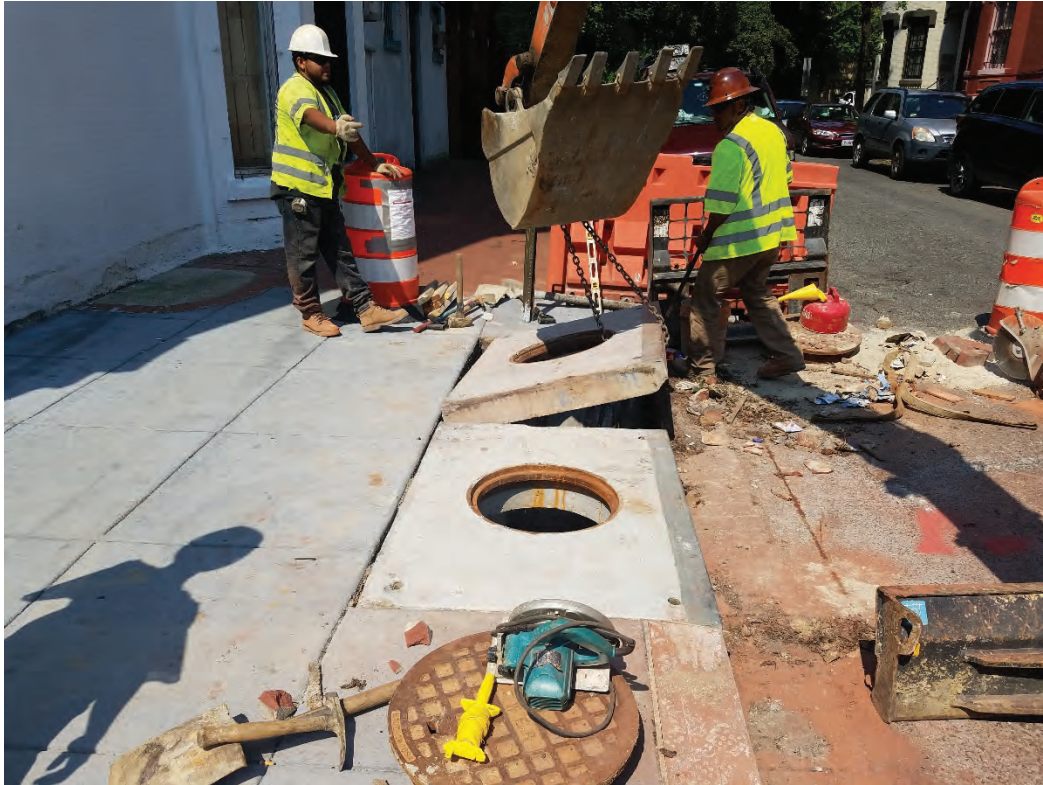
Adjustment of catch basin frame top at Corcoran St by Omni.
