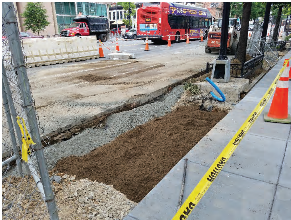
Structural soil placed at tree zone near 2013 14 th St.
